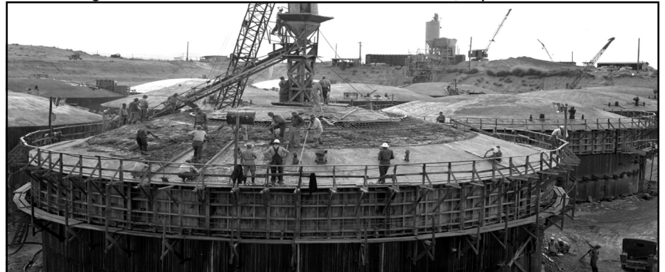
Waste Storage Tanks under Construction at DOE's Hanford Site, September 1947
