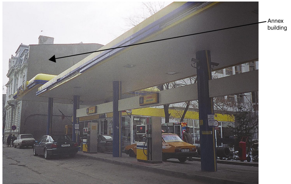
Figure 2: Public Gas Station behind an Embassy Annex Building Poses Security Concern
