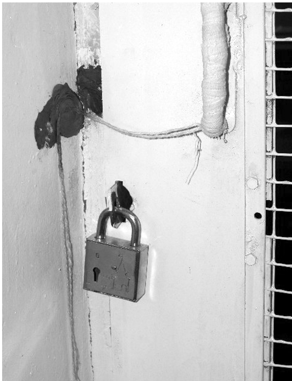
Figure 6: Wax and String Seal Securing Room with Dangerous Biological Pathogens
