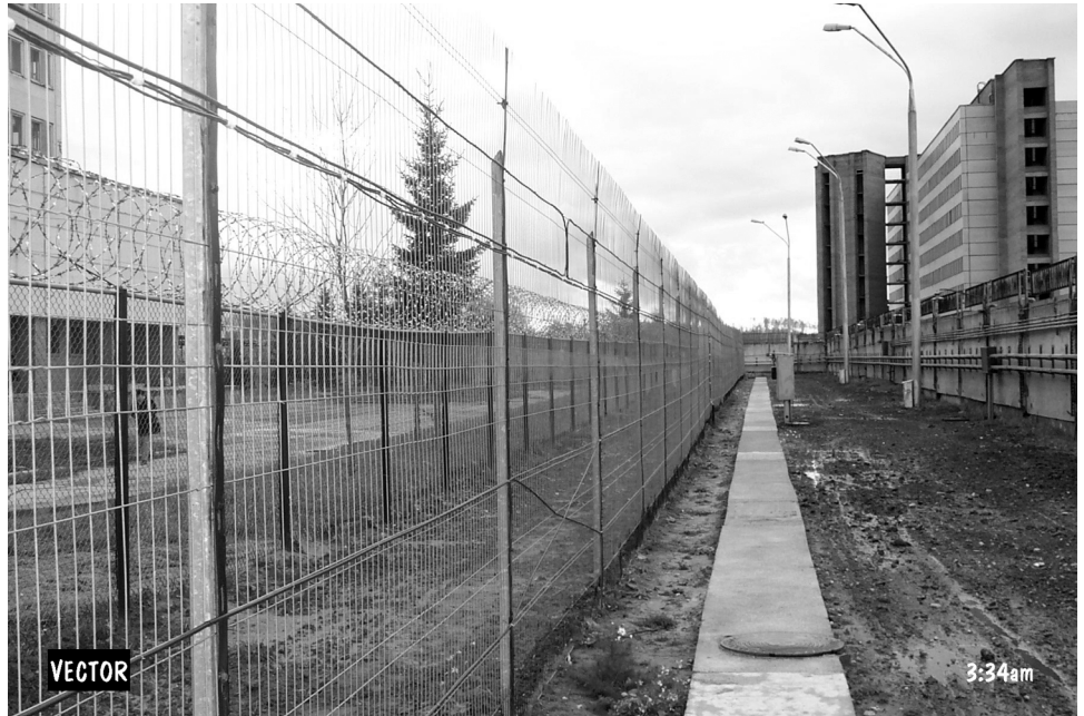
Figure 7: DOD-Funded Three-fence Perimeter around Buildings at Vector with Smallpox and Other Dangerous Pathogens
