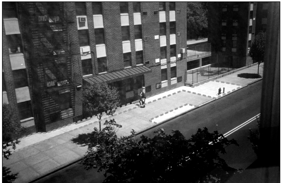
Figure 3: Sidewalk Repairs at HUD Property
