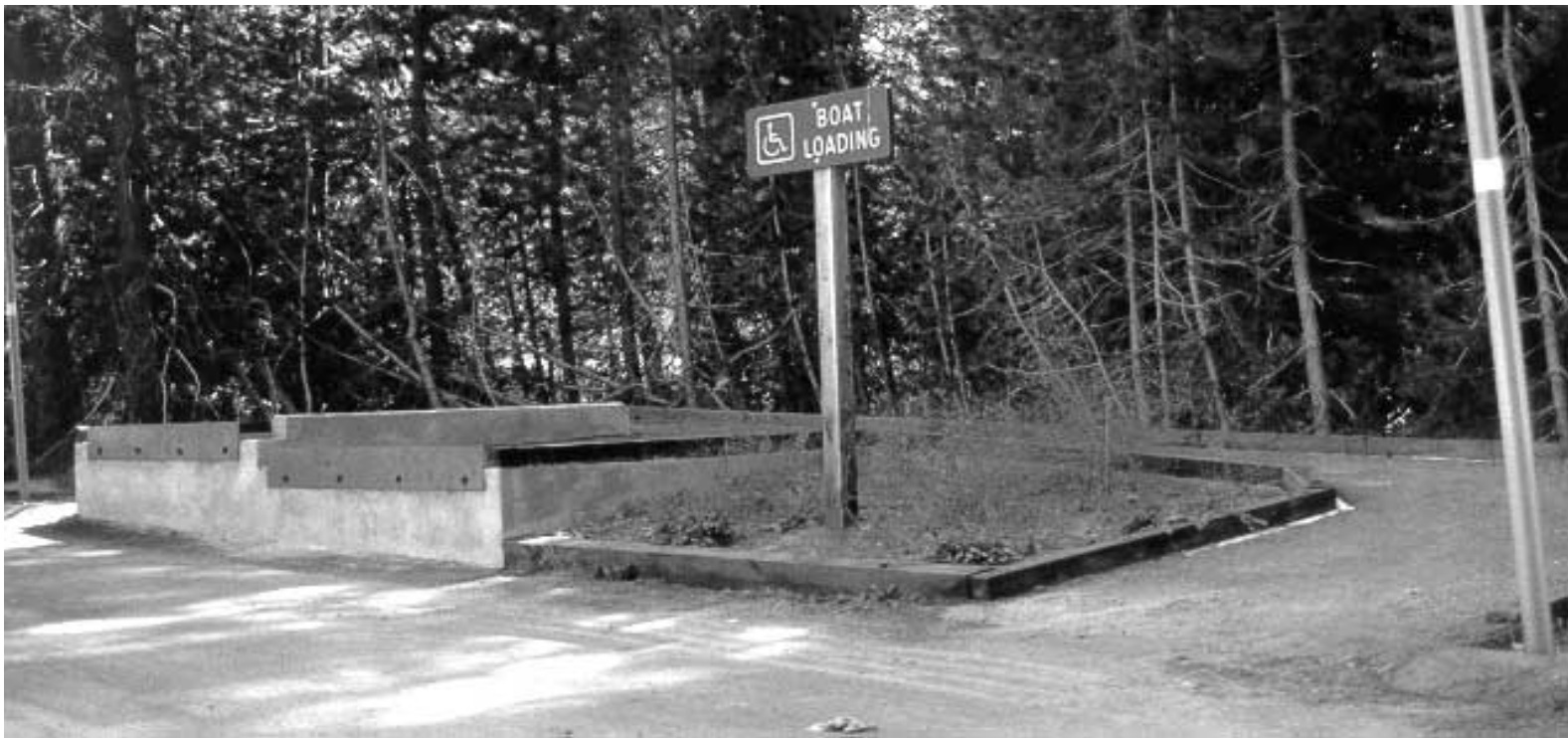
Figure 3- Split-level concrete ramps allow easy access to boats of different heights.
