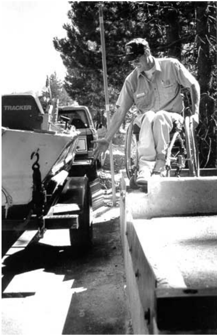
Figure 8 - A ramp recessed behind curbs makes loading and unloading difficult.
