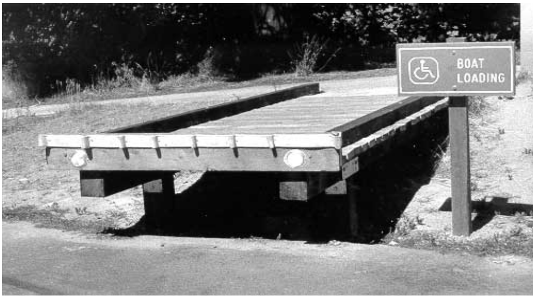
Figure 4-A typical timber ramp.
