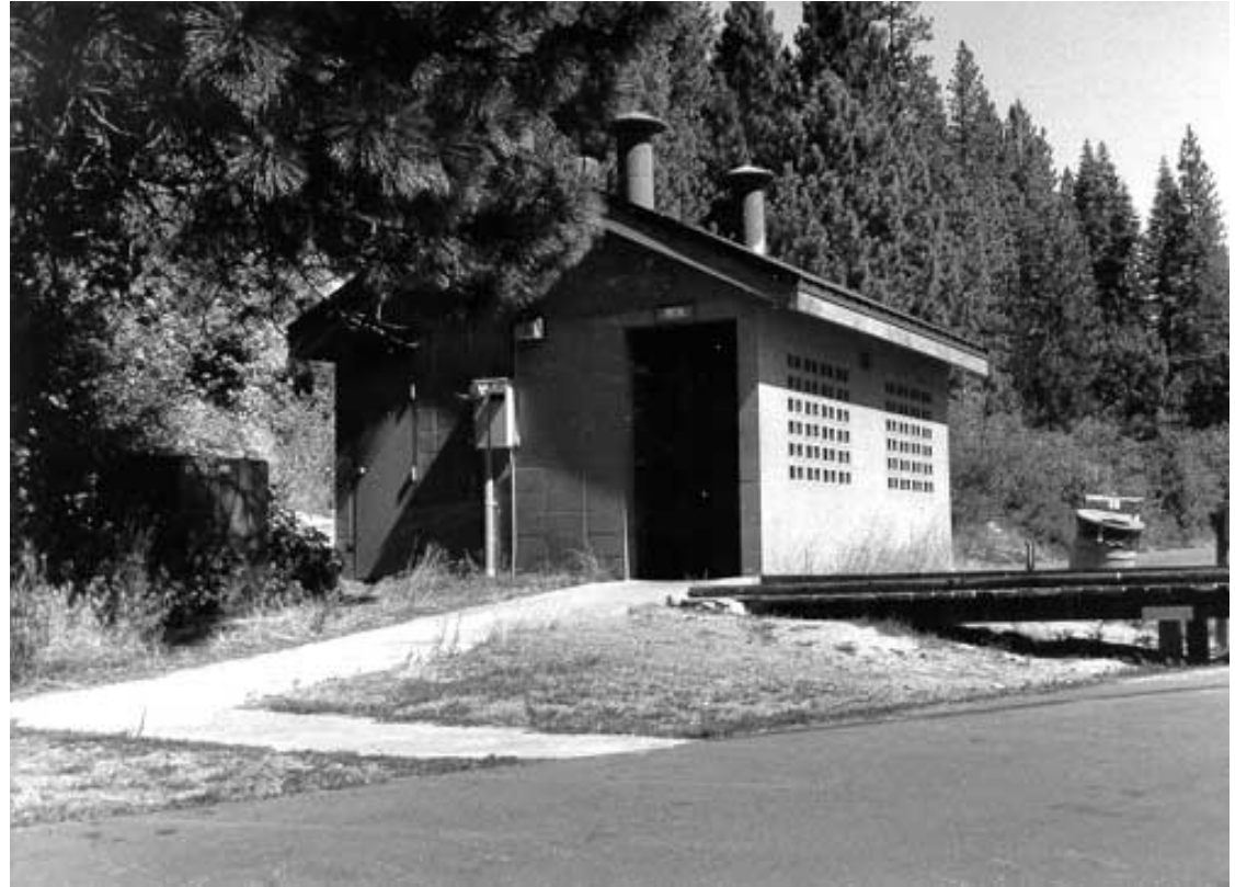
Figure 7 - A timber boarding platform built alongside an existing restroom.
