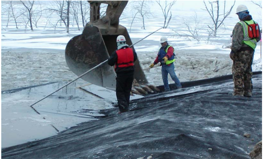
Placing fabric on embankment before placing rock (riprap)
