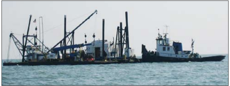
This barge is sucking up shoaled material from the bottom of Saginaw Bay and pumping it into a nearby disposal facility, popularly known as Channel Island.
