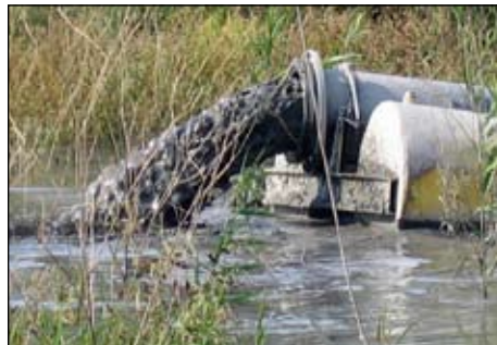
A slurry of shoaled material flows into the Saginaw Bay Confined Disposal Facility. The pipe spewing the muddy water is connected to a nearby hydraulic dredging barge in Saginaw Bay.
