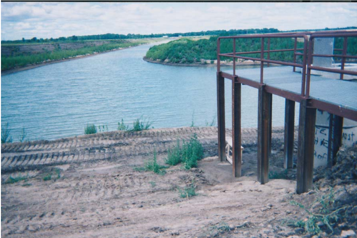
Photo#6 – picture of perimeter dike outlet weir.
