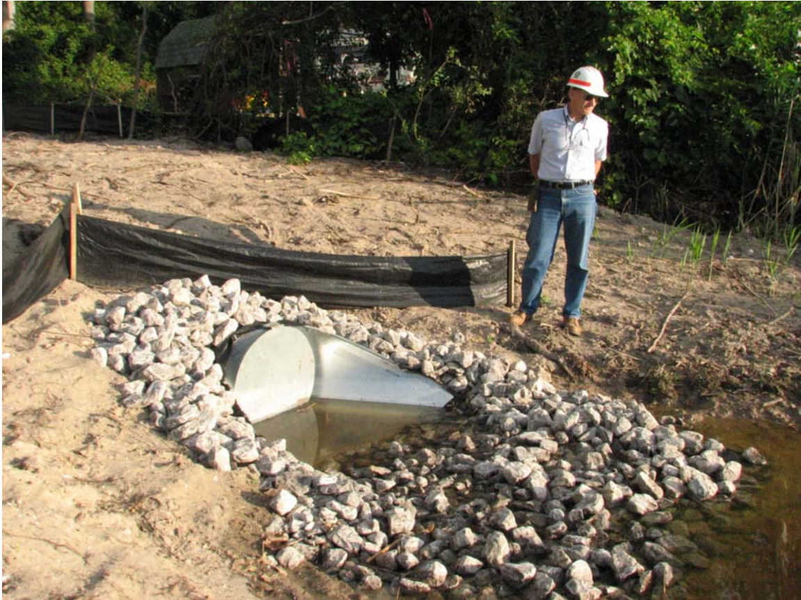
Photo #5 – picture taken of outfall into Saginaw River.
