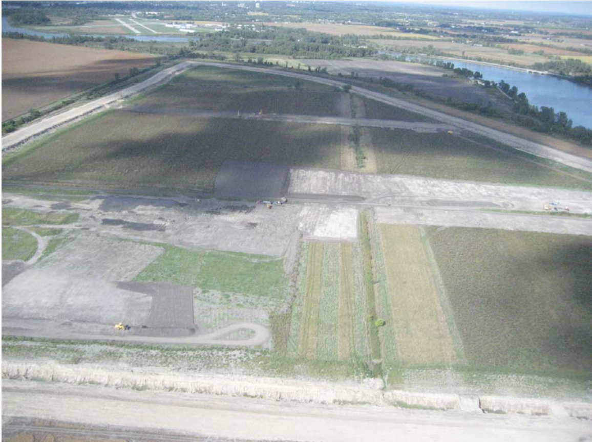
Photo #2 – Aerial photograph of entire site prior to construction of the new DMDF
