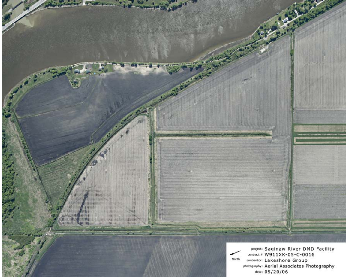
Photo #1 – Aerial photograph of entire site prior to construction of the new DMDF
