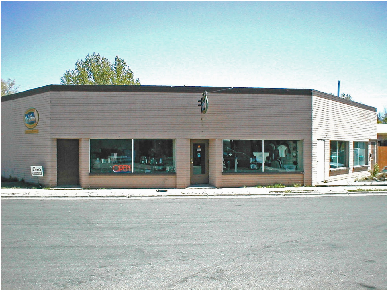
Figure 30-(b) current appearance of the front of the old Rock Lab building at 16-18 Mike's Pike; now occupied (at the time of this writing) by Flag Tee Factory; digital photo G. Schaber 13 May 2002.
