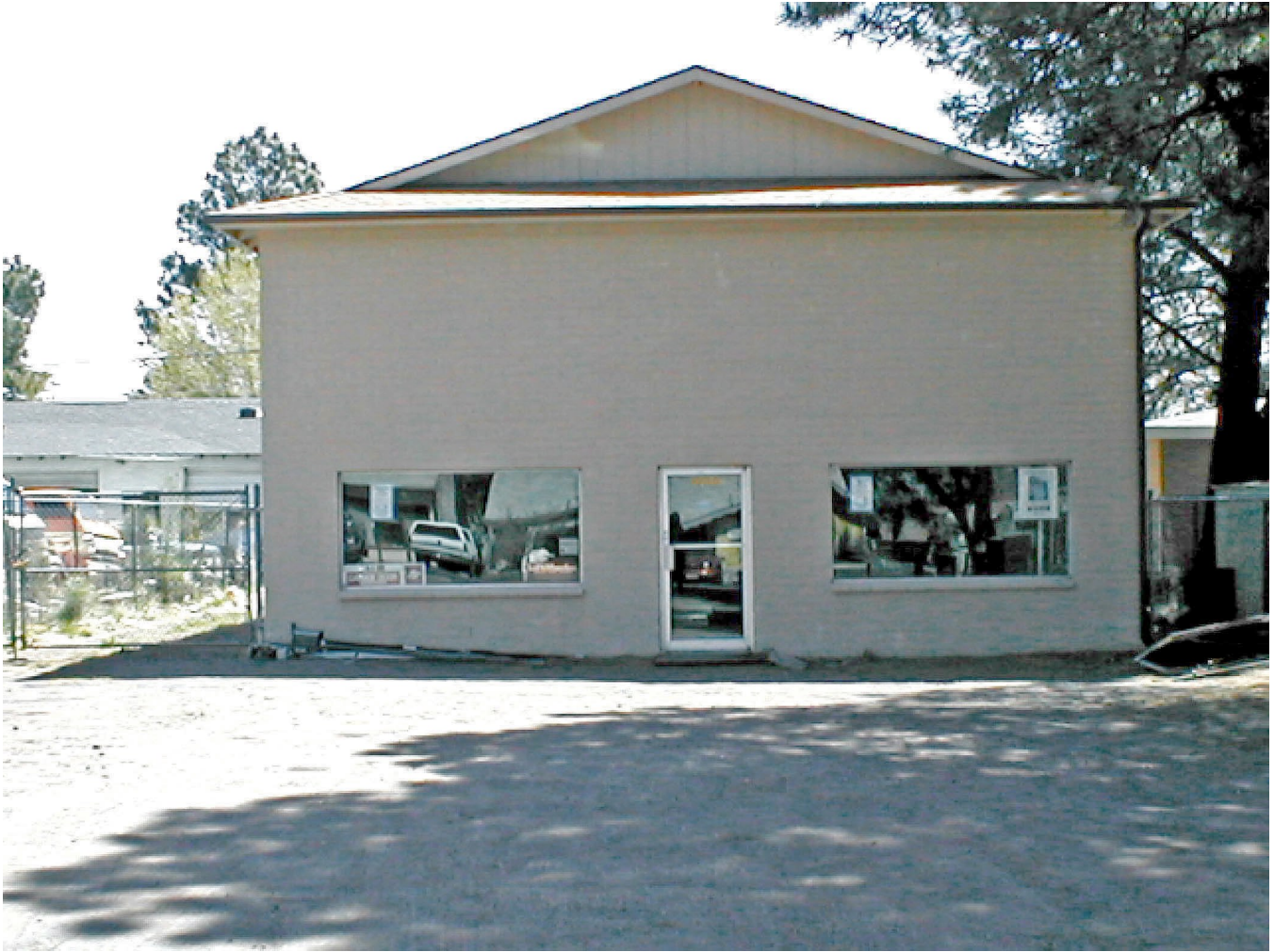
Figure 21-(a) Current exterior view of the machine shop that was located at 1733 N. West Street in the Sunnyside area of East Flagstaff-after it was relocated from the Museum of Northern Arizona; digital photo-G. Schaber, 6 May 2002
