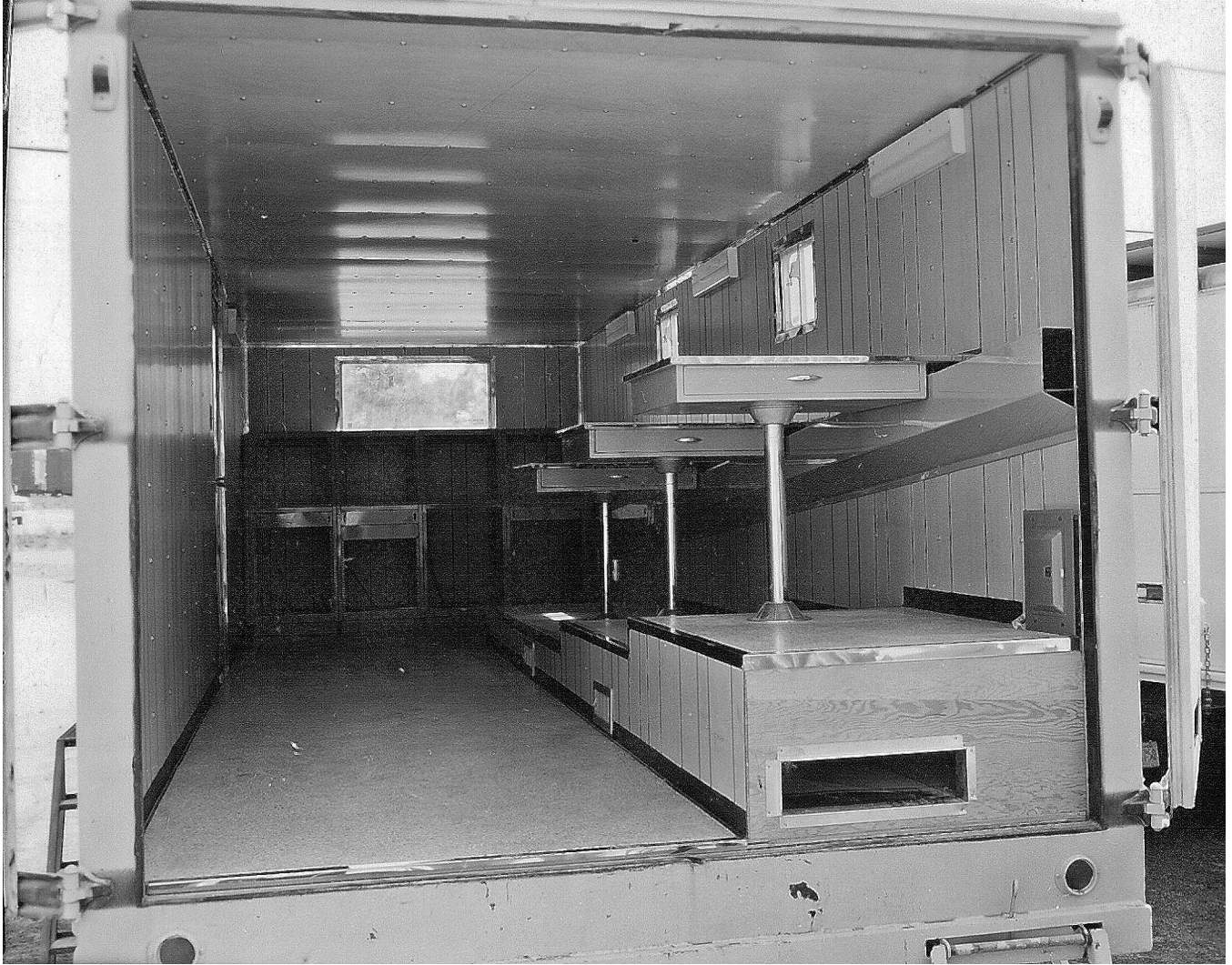
Figure 28-(b) inside view of interior of ADF trailer (under construction); USGS photo P609, F66896.
