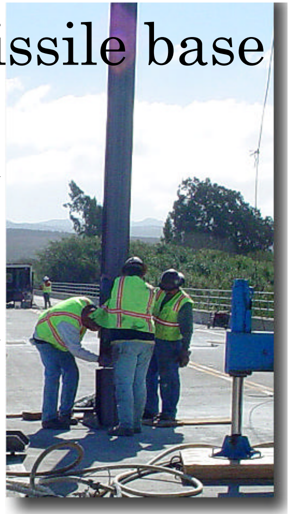
Corps contractors guide 50-foot micropiles
