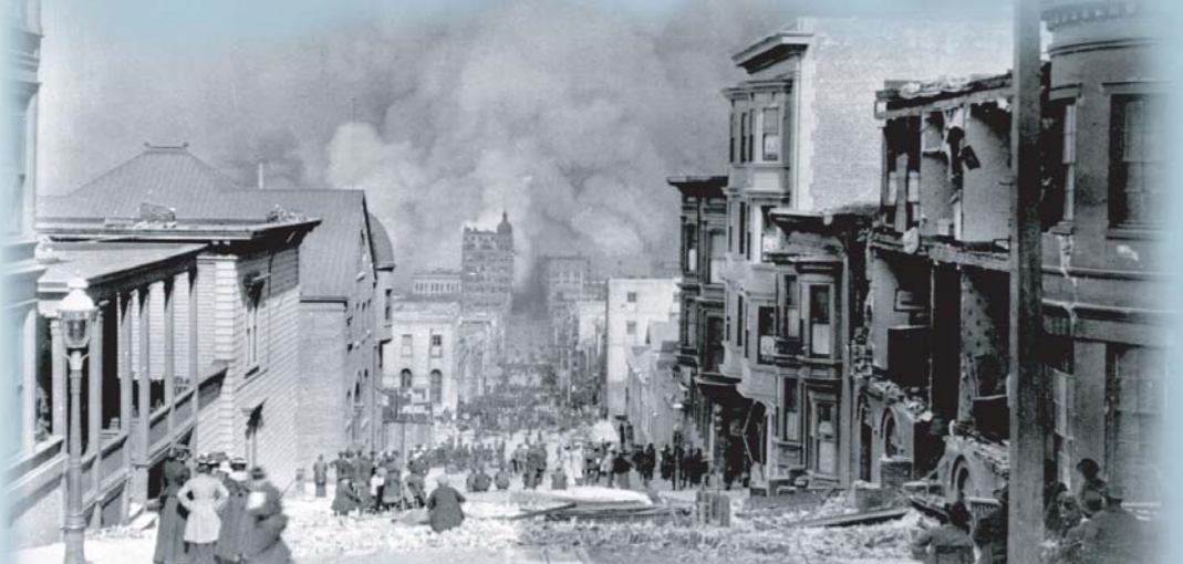
Figure 3. —View down Sacramento Street in San Francisco showing building damage caused by the earthquake of 1906. Smoke in background is from approaching fires that were ultimately more damaging than the shaking itself. Photograph by Arnold Genthe (American 1869–1942); silver gelatin print; image 200 x 329 mm (7 7 / 8 x 12 15 / 16 in). Courtesy of Fine Arts Museums of San Francisco, Museum Collection A046248.
