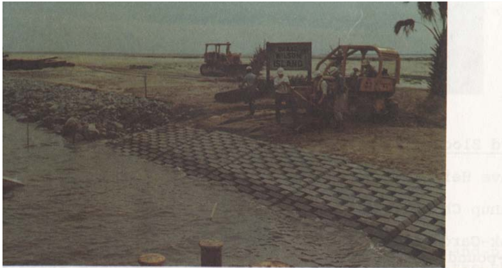
Figure B-11 Terrafix Block Revetment (Photo Courtesy of Erosion Control Products, Inc.)
