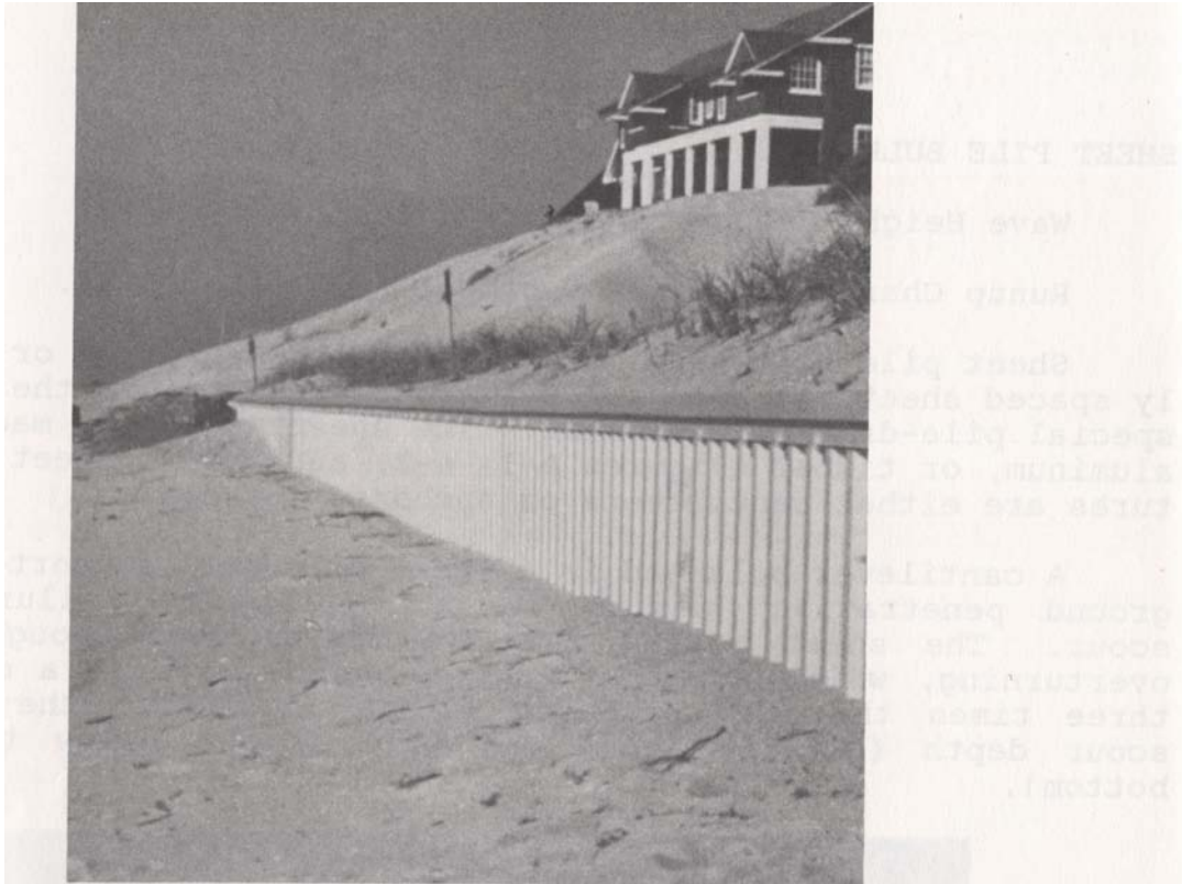
Figure A-2 Aluminum Sheet Pile Bulkhead (Photo Courtesy of Koppers Company, Inc.)
