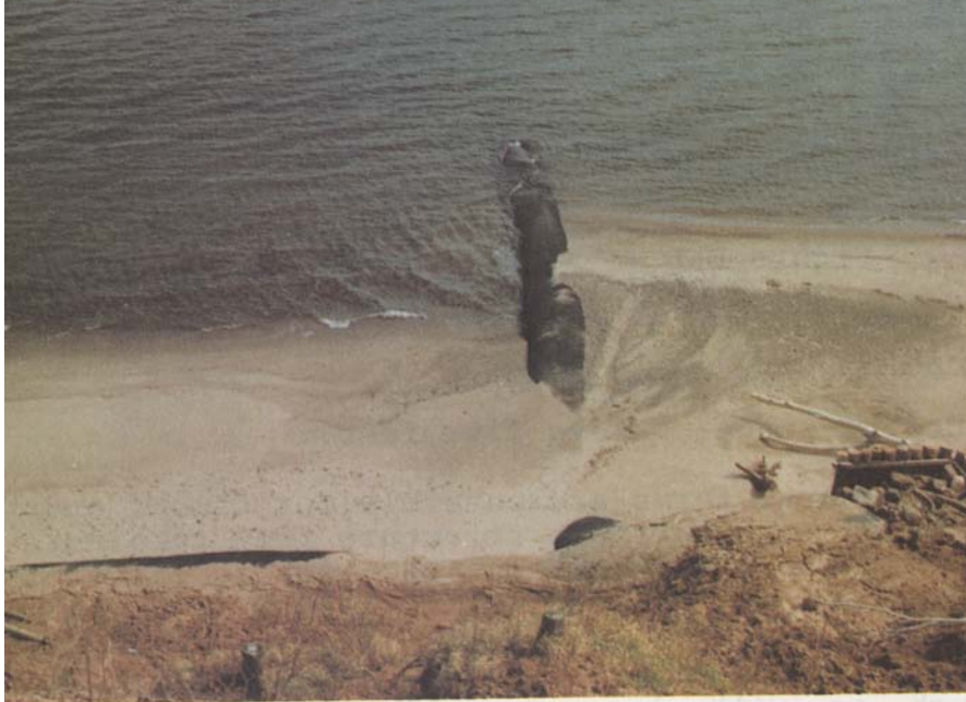
Figure D-4 Longard Tube Groin
