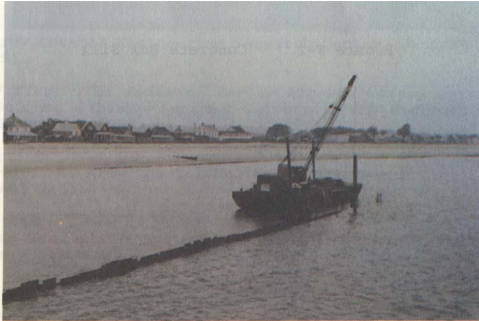
Figure F-1 Timber Sheet Pile Sill Under Construction
