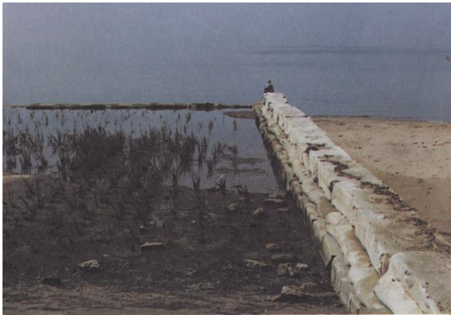
Figure D-1 Stacked Bag Groin
