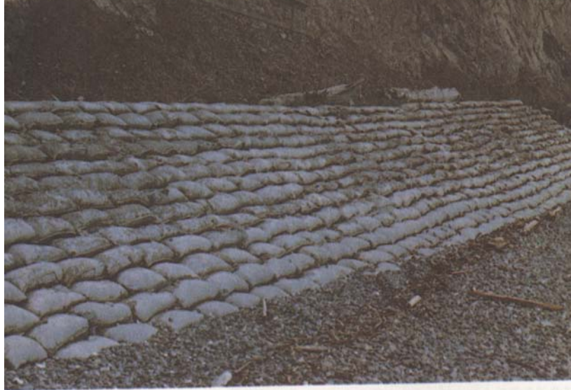
Figure B-12 Stacked Bag Revetment
