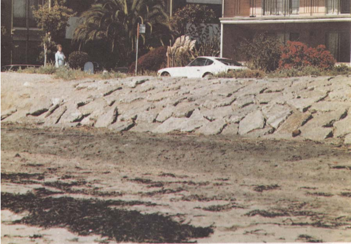
Figure B-2 Concrete Rubble Revetment
