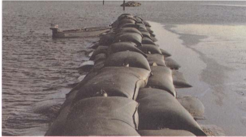
Figure C-3 Sand-Filled Bag Breakwater
