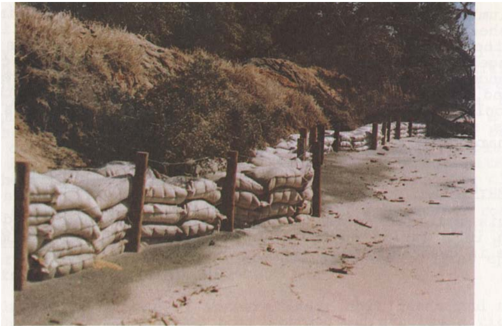
Figure A-7 Hogwire Fence and Stacked Bag Bulkhead
