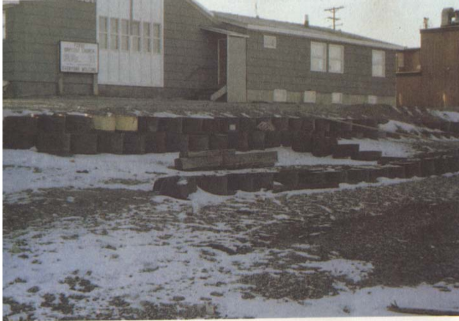
Figure B-16 Steel Fuel Barrel Revetment
