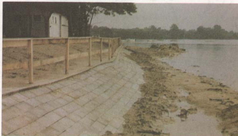
Figure 16 Concrete Block Revetment
