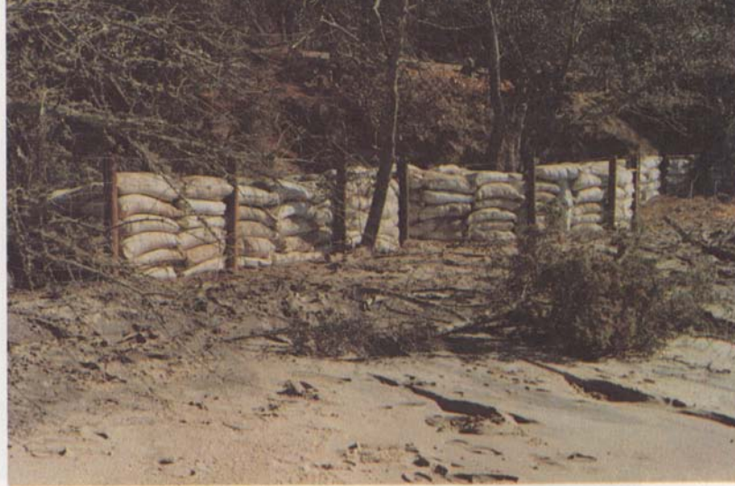
Figure 35 Hogwire Fence and Sand Bag Bulkhead (December 1978)
