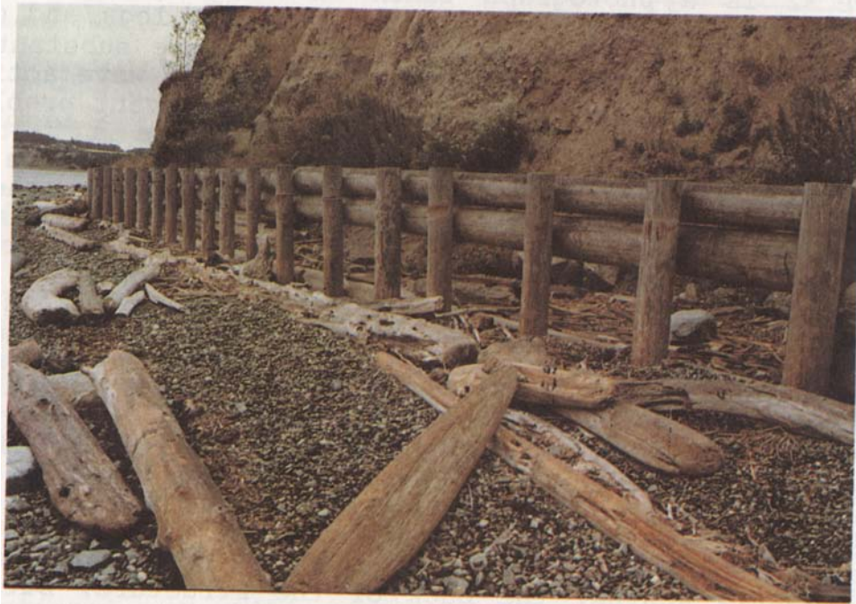
Figure 33 Untreated Log Bulkhead (February 1979)
