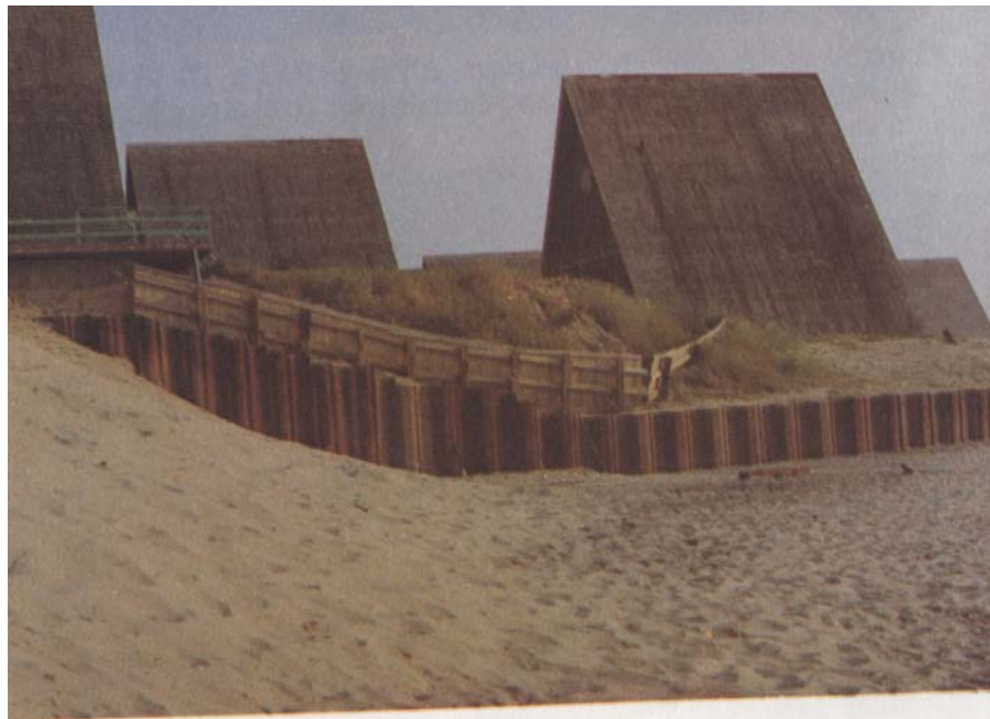
Figure A-1 Steel Sheet Pile Bulkhead
