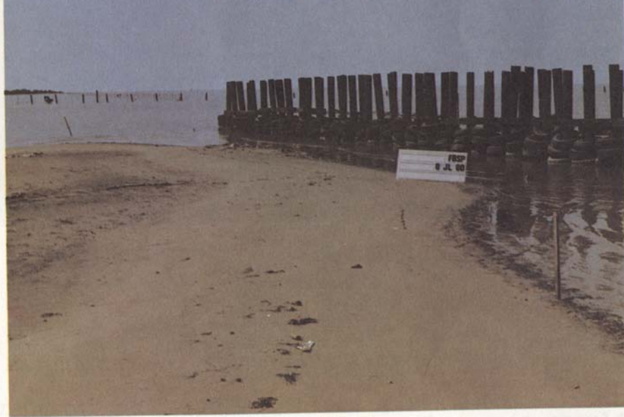
Figure C-12 Used Tire and Timber Pile Breakwater
