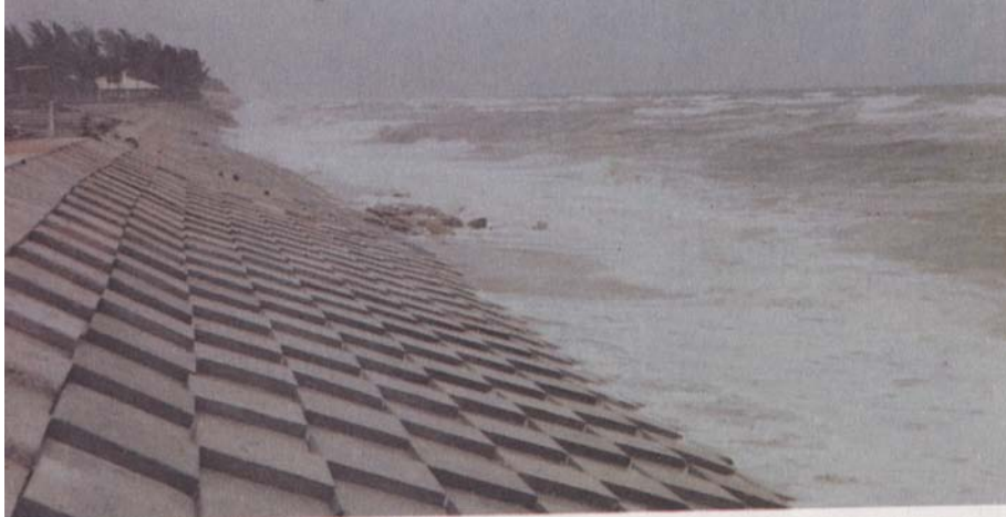
Figure B-9 Shiplap Block Revetment
