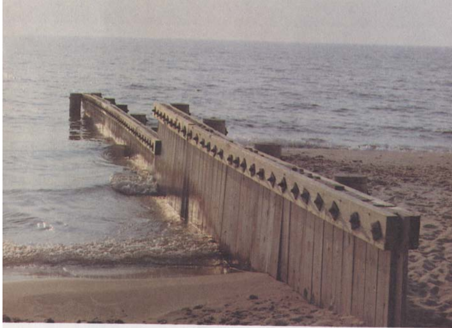
Figure D-5 Timber Sheet Pile Groin
