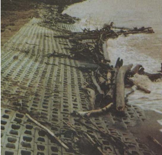
Figure B-8 Control Block Revetment
