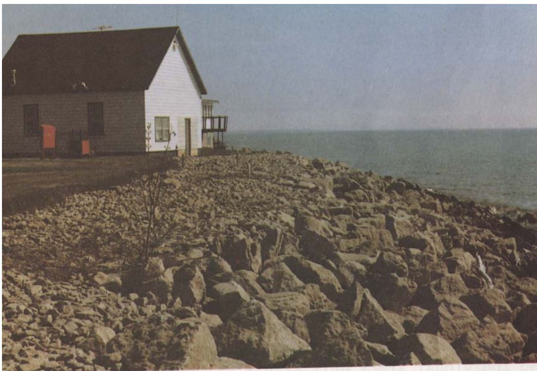
Figure B-1 Stone Revetment
