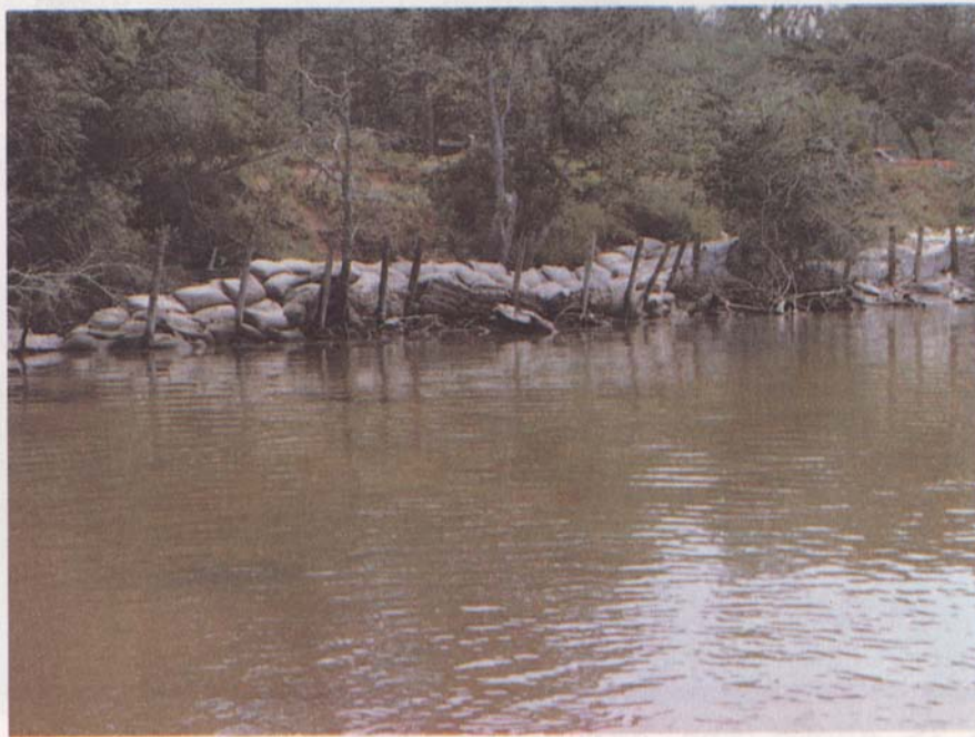
Figure 36 Hogwire Fence and Sand Bag Bulkhead (June 1979)
