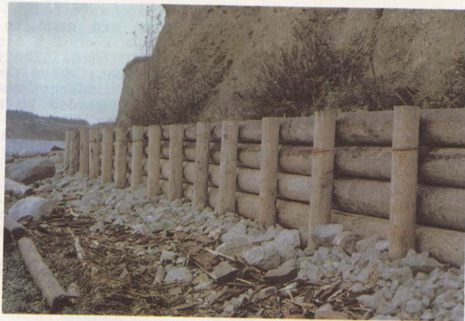
Figure 32 Untreated Log Bulkhead (November 1978)
