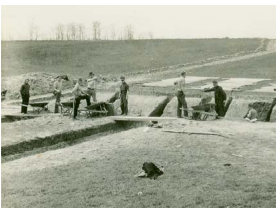
CCC and WPA workers constructing NAEW lysimeters in 1939
