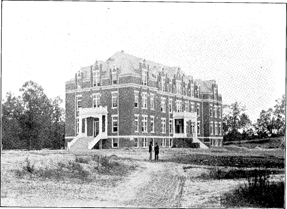
Marist Seminary at Catholic University, Washington, D. C. A. O. von Herbulis, Architect. Floors and stairways in ferro concrete.
