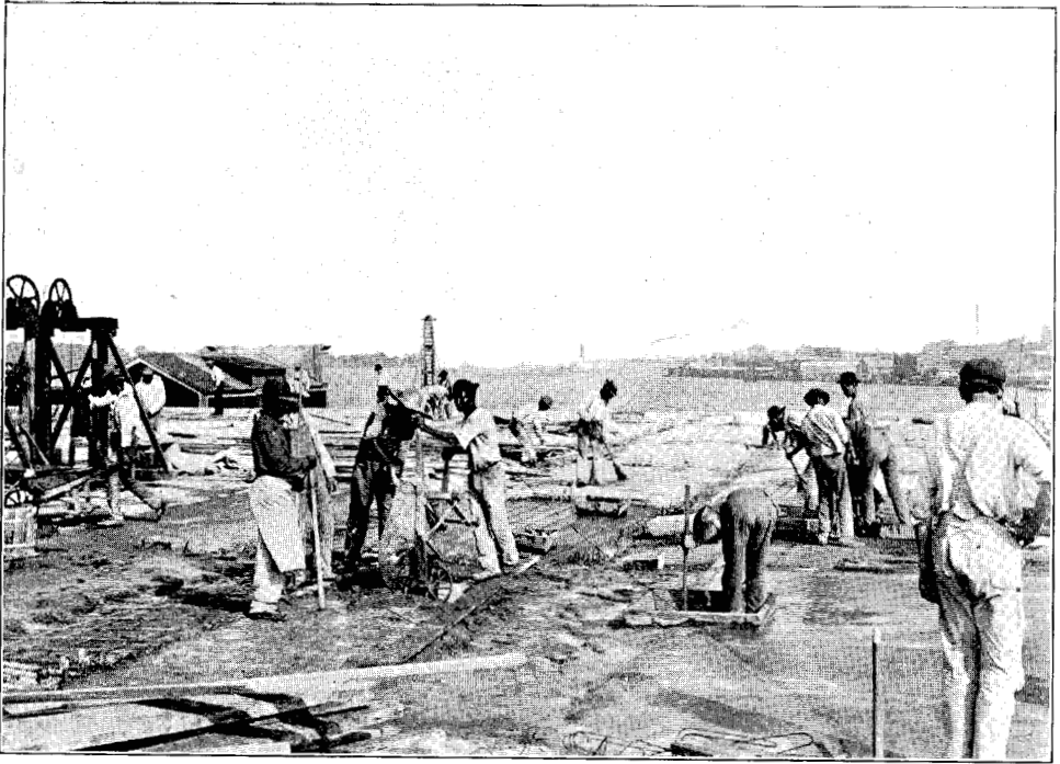
Wine Warehouse at Berkley, Va. (See page 27.) Construction of a floor.
