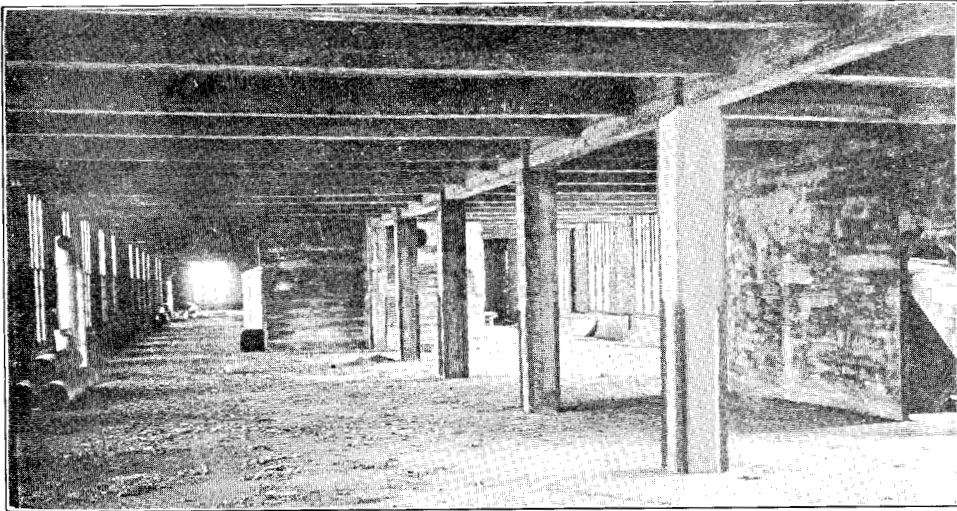
The J. L. Mott Iron Works. New Plant at Trenton, N. J. Third floor of the Brass Shop (see page 34).
