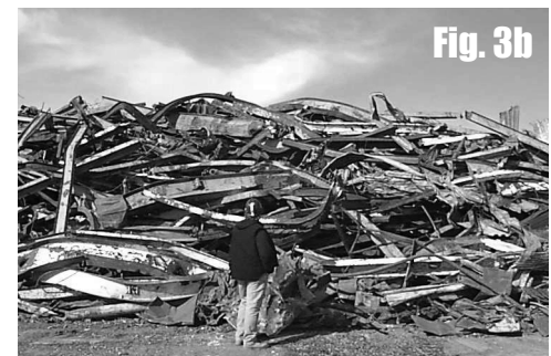
Building 845 after demolition
