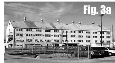
Building 845 before demolition
