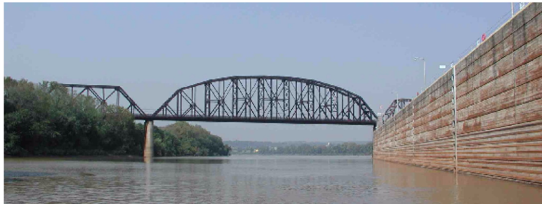
K & I RAILROAD & HIGHWAY BRIDGE (Ohio River Mile 607.4)
