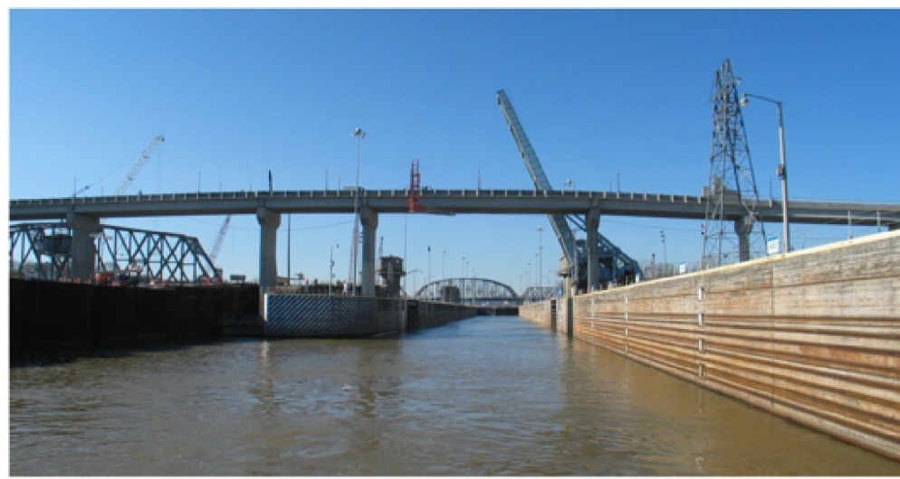
McALPINE LOCKS BRIDGE (Ohio River Mile 606.8) Downstream View
