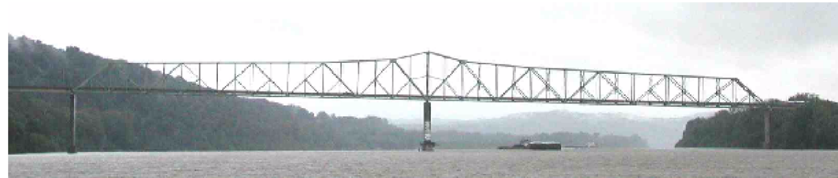
MATTHEW E. WELSH HIGHWAY (SR 135) BRIDGES (Ohio River Mile 647.8)
