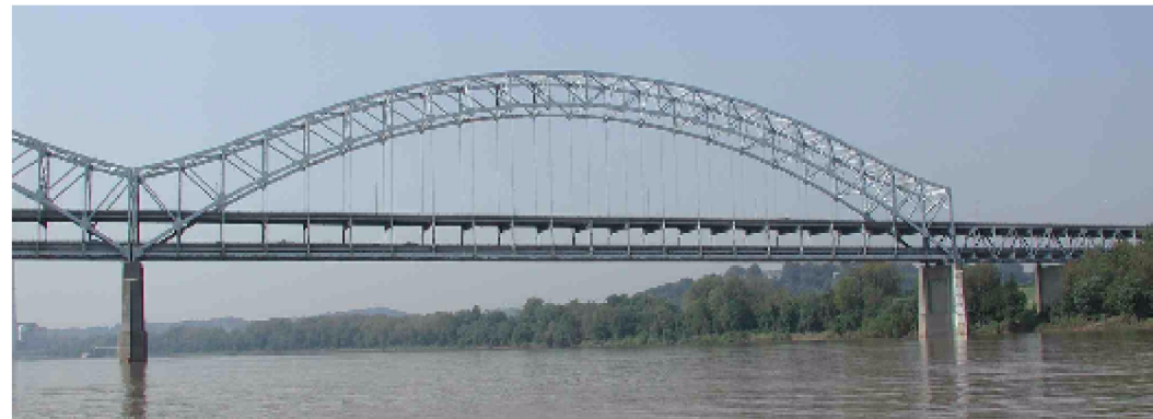
SHERMAN MINTON HIGHWAY (I-64) BRIDGE (Ohio River Mile 608.6) Downstream View
