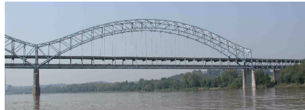
SHERMAN MINTON HIGHWAY (I-64) BRIDGE (Ohio River Mile 608.6)
