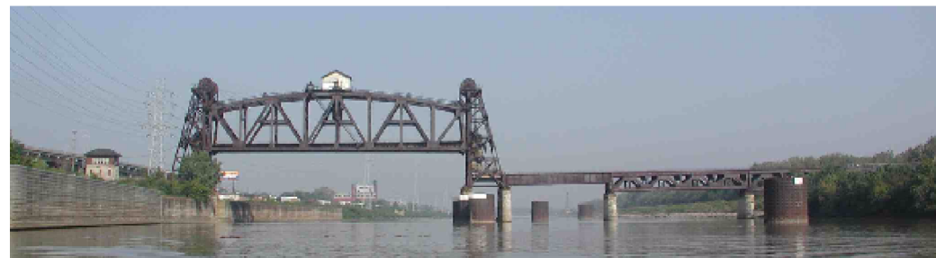
LOUISVILLE & INDIANA RR BRIDGE (Ohio River Mile 604.4)
