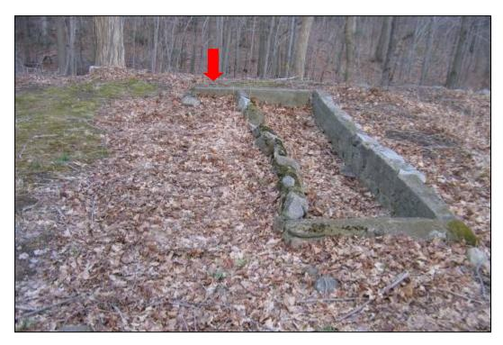
**Figure 3.2**. Original carriage house, rubble foundation wall and abutting concrete greenhouse foundation with partial rubble facing (2006). Red arrow indicates extension of greenhouse foundation under southeast corner of the carriage house.
