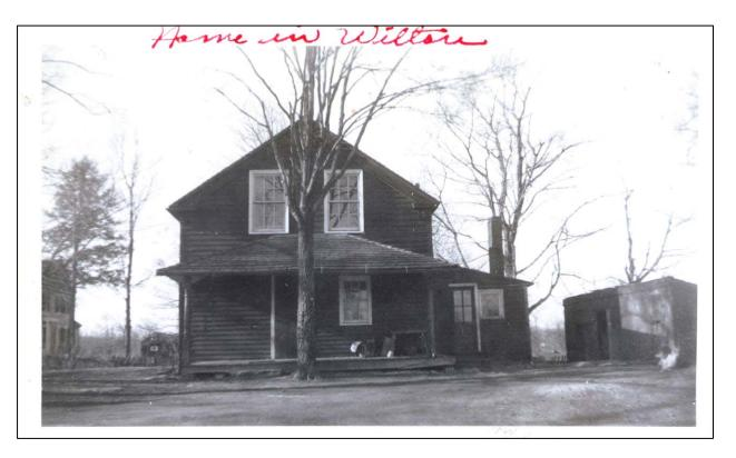
**Figure 1.11.** Bass family photograph, showing south elevation of caretaker's house with enlarged second-story windows (mid 1930s- 1944).
