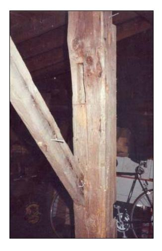
Figure 3.11. Caretaker's garage: Interior view, showing reused post with empty mortises (1994).
