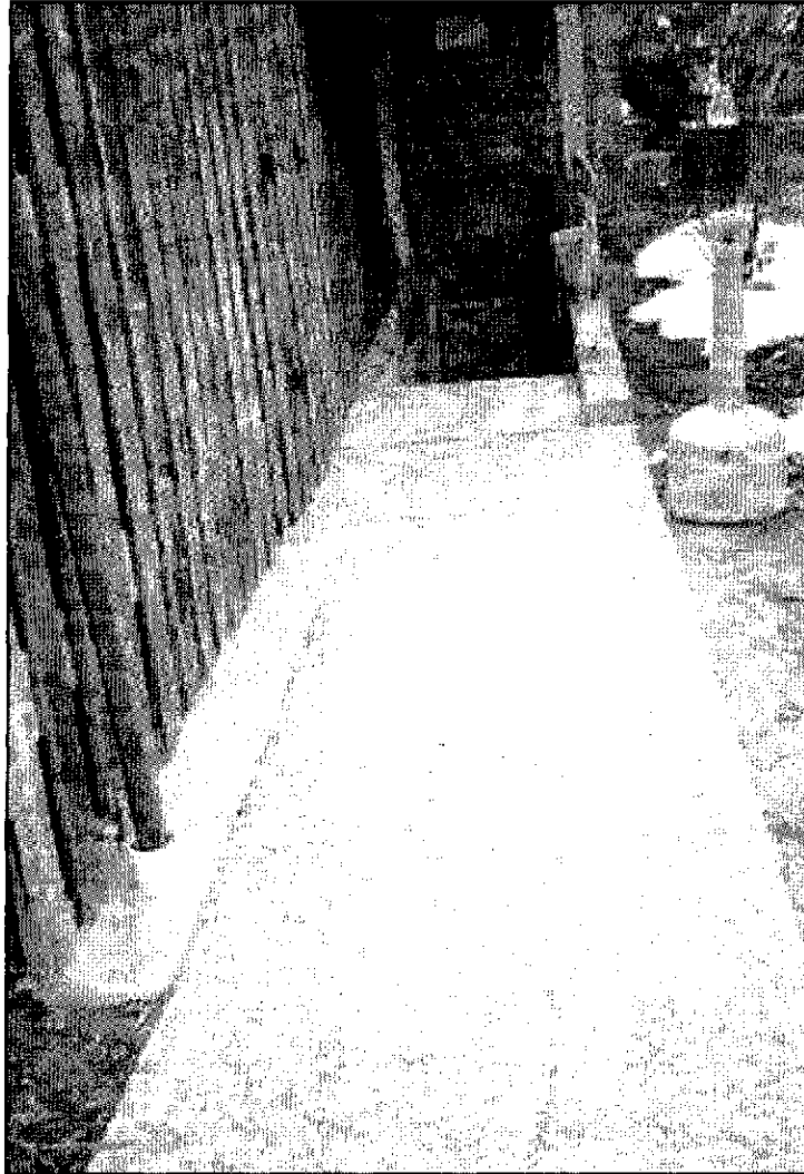
Figure 4.4: Pedestrian path to basement entry, view to southeast.
