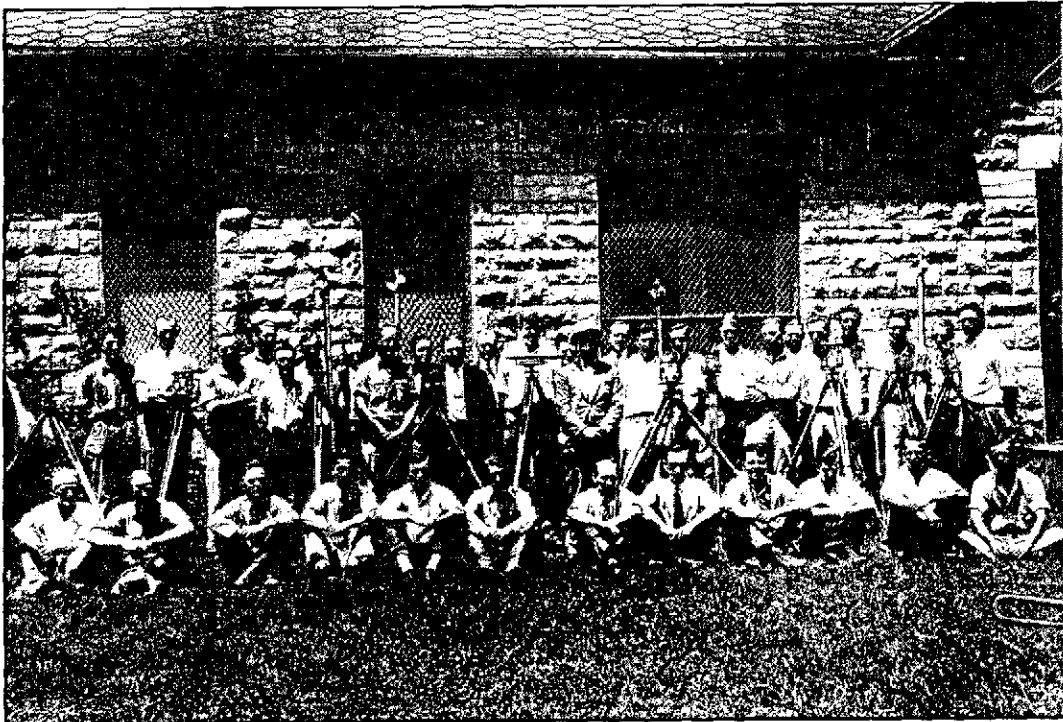
Figure 2.7: July 7, 1932, photograph of a survey crew outside the Survey Lodge. Note the metal screens over the windows and the hexagonal asphalt shingle roof (NPS-NCR Collection).
