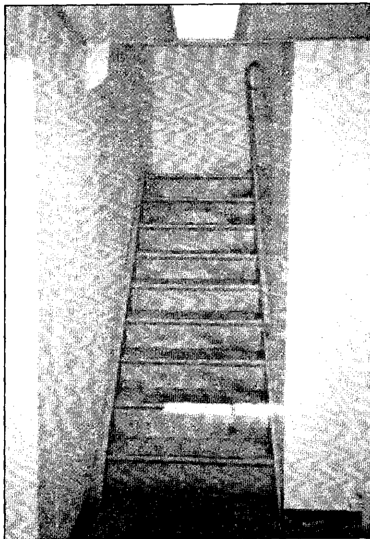
Figure 4.29: Stair, view to northeast from basement floor landing.
