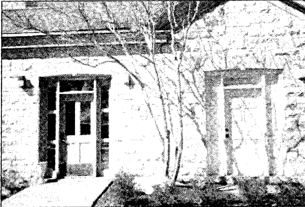
Figure 4.8: Southeast elevation with current entry on left and historic entry on right.
