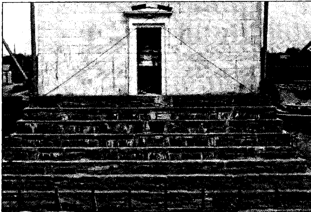
Figure 3.2: View of earlier stepped stone foundation and portal door. (NPS-NCR Collection.)
