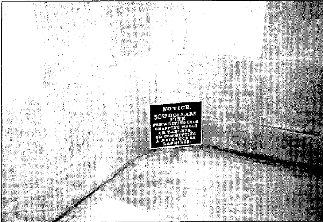
Figure 4.41: No-vandalism signs were added in 1904 to every other landing.
