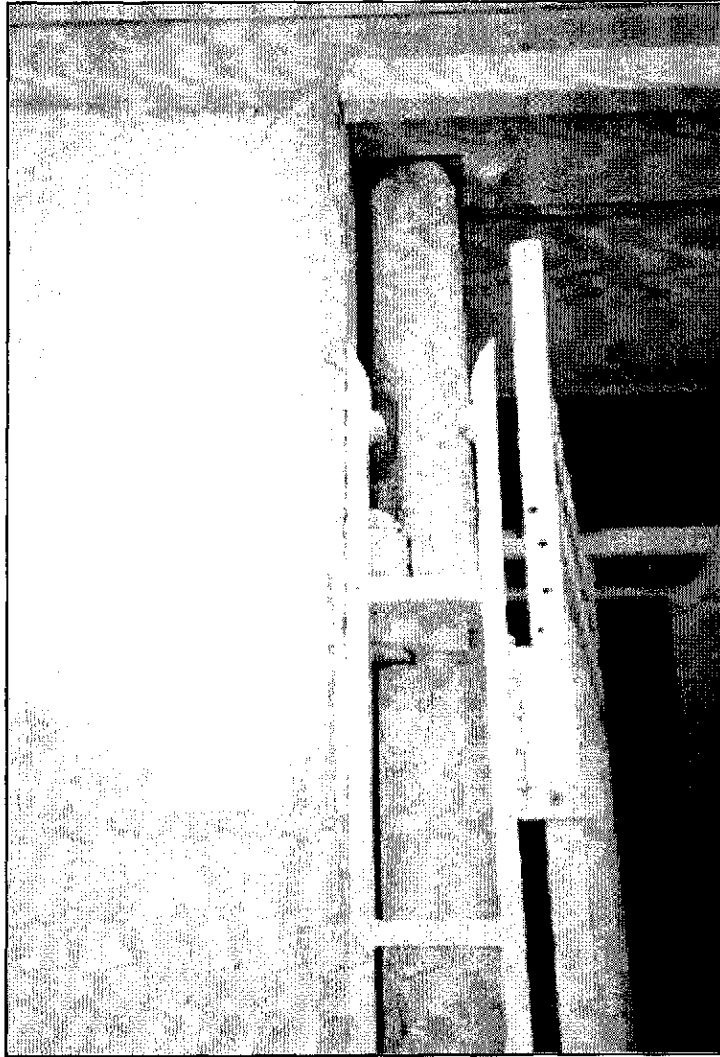
Figure 4.53: Interim security building, west room. view to the west showing the marble door and metal gate connection.
