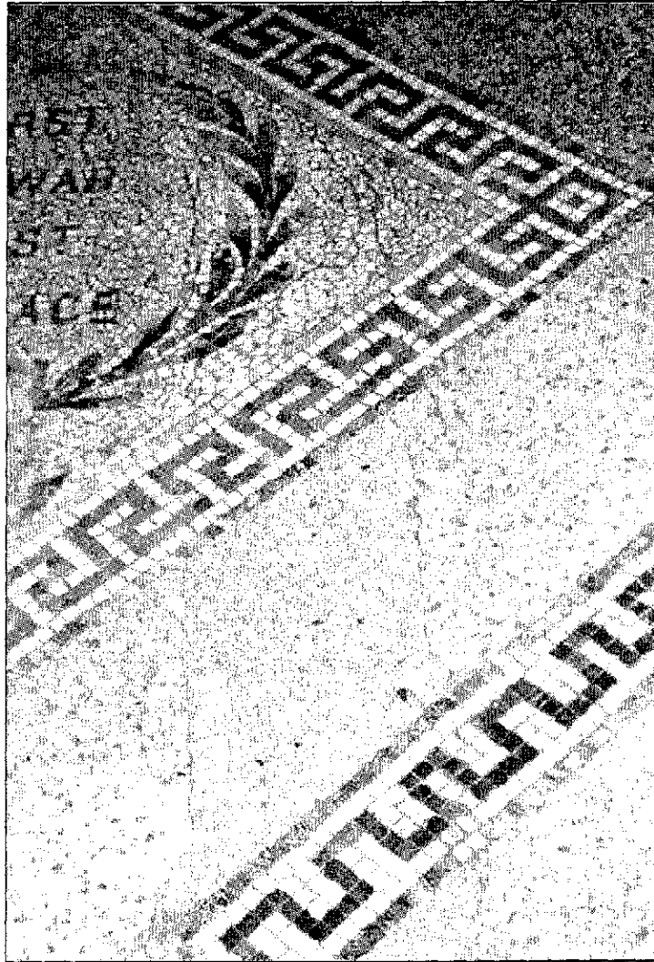
Figure 4.32: South corridor, east end showing terrazzo floor repair.
