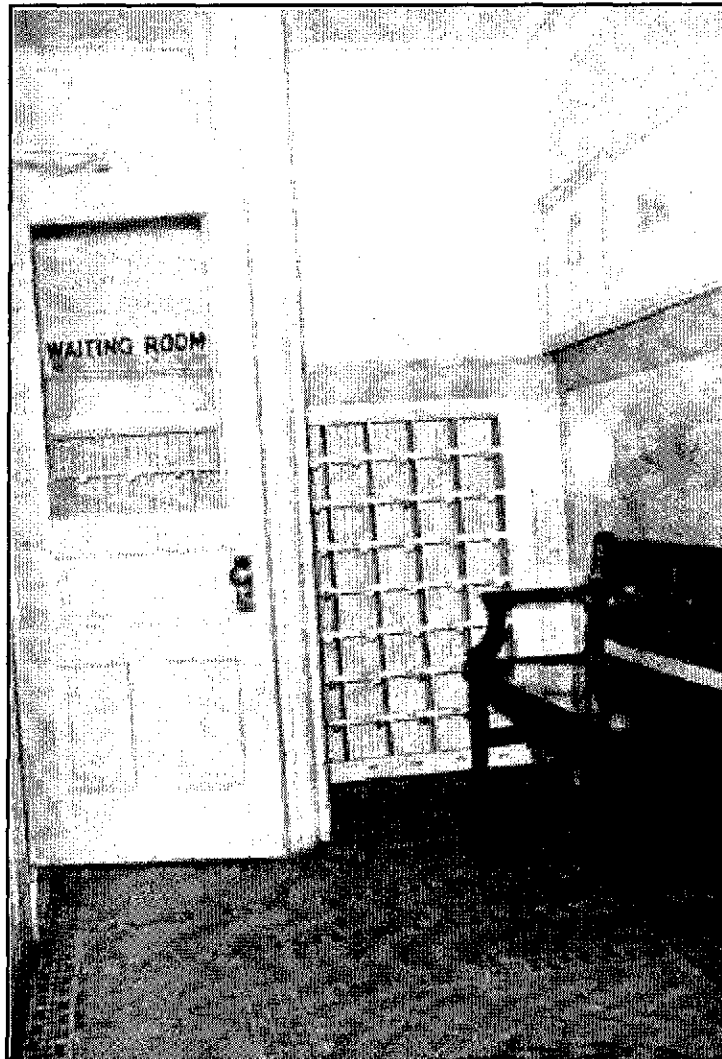
Figure 3.26: Southeast corner of Washington Monument Waiting Room, c. 1940s, NPS-NCR Collection.
