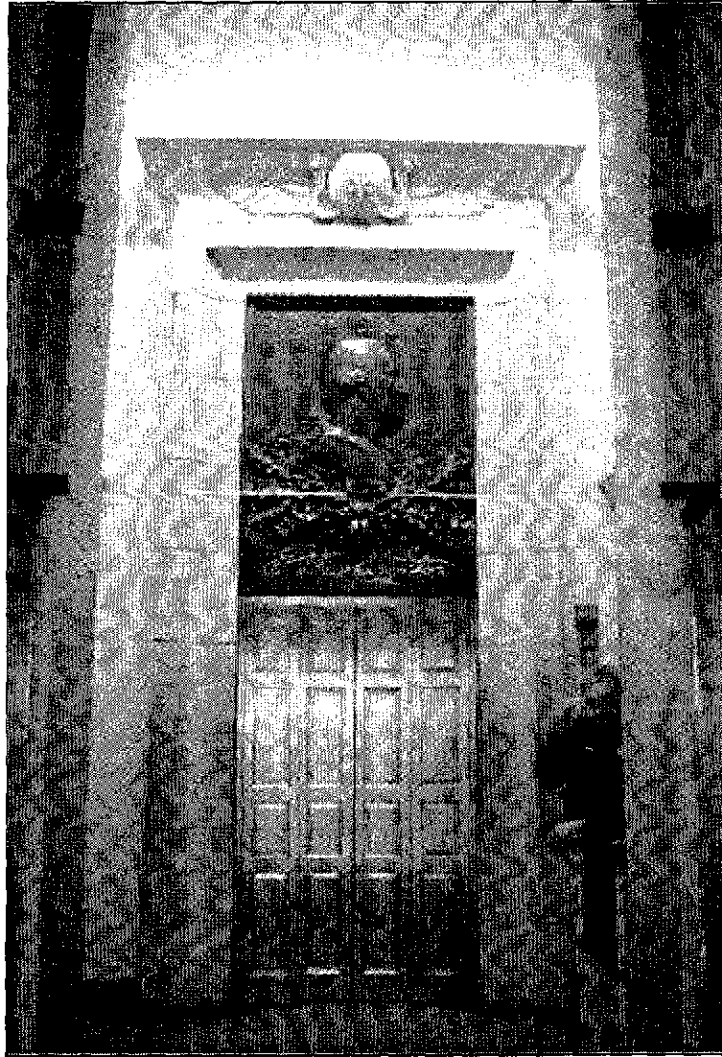
Figure 4.30: East elevator lobby, view to the west, showing the elevator doors, bronze transom panel, and limestone door surround.
