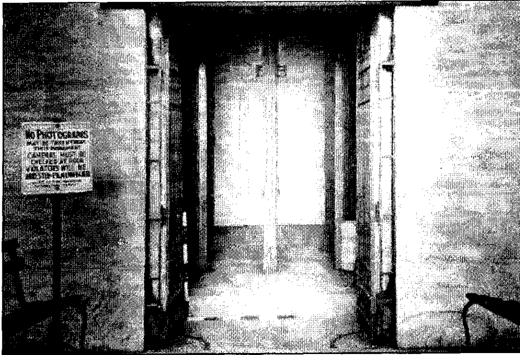
Figure 3.27: Washington Monument East Entrance, looking in, c. 1940s, NPS-NCR Collection.
