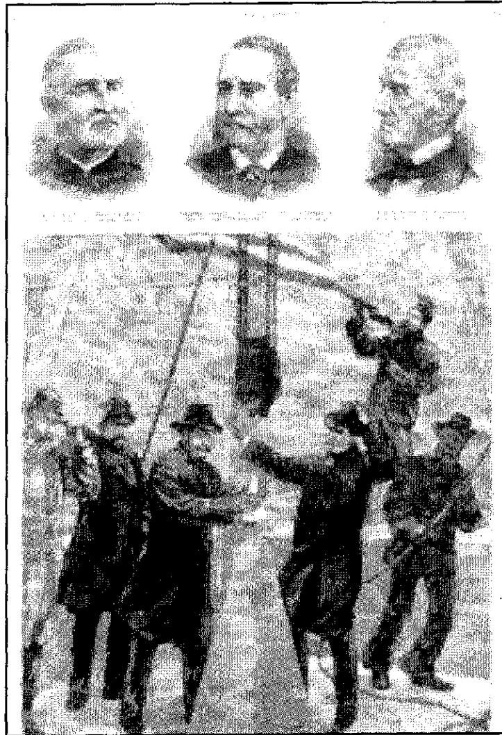
Figure 2.12: Setting the capstone on the Washington Monument, December 6, 1884. (S. H. Nealy. "572 feet high – Setting the Capstone on the Washington Monument." Harper's Weekly , 20 December 1884, p. 839; Prints and Photographs Division, LC-USZ62-89199, Library of Congress, Washington, DC.)
