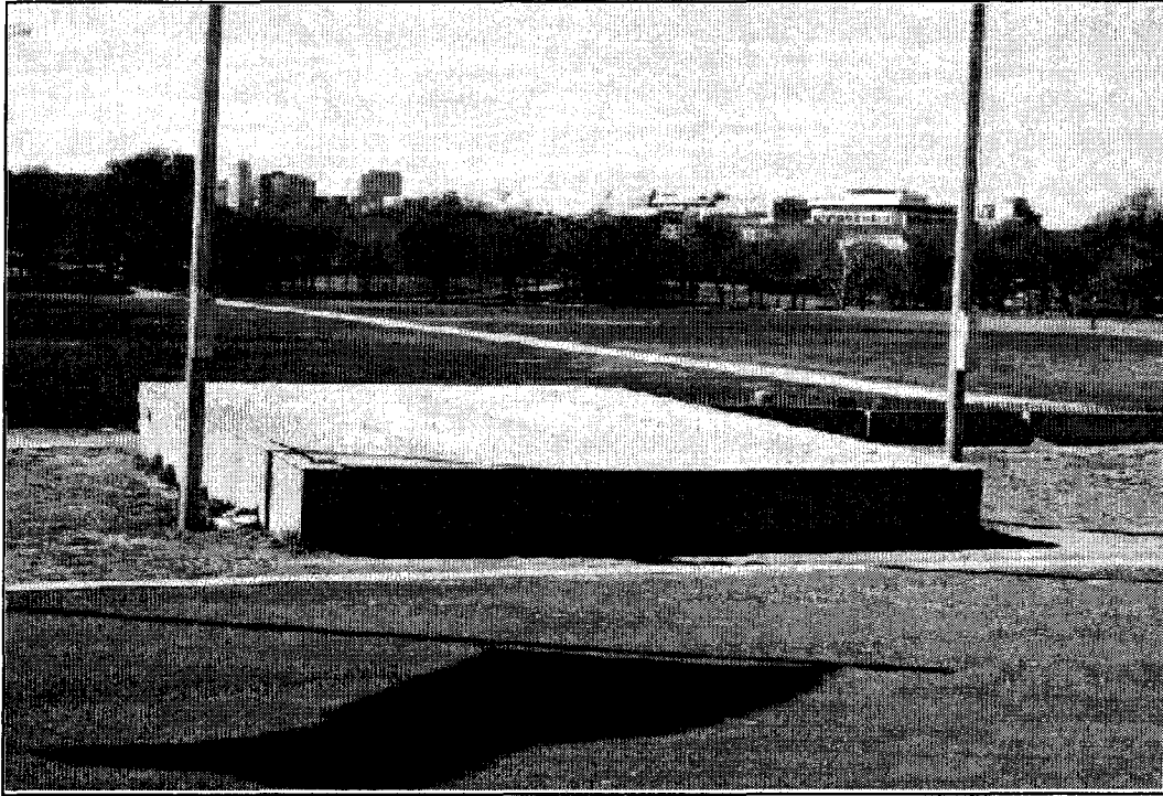
Figure 4.5: Floodlight vault, view to the west.
