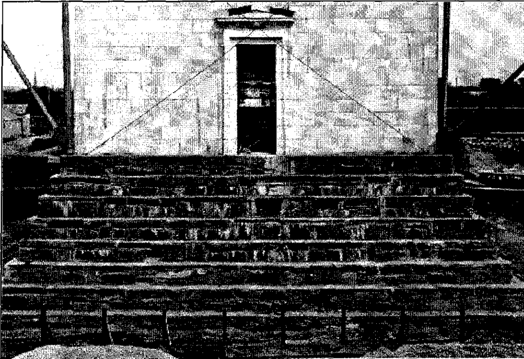
Figure 4.8: Historic construction photograph showing the original stepped blue gneiss foundation of the Washington Monument. ("Foundation of Washington Monument, from the south," August 14, 1879, Prints and Photographs Division, LC-USZ62-30613, Library of Congress, Washington, D.C.)
