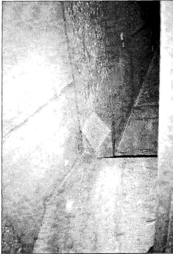
Figure 4.50: Pyramidion interior, view to top, with carved marble brackets sitting on rib. Note stones with brackets were not finished smooth on the interior.
