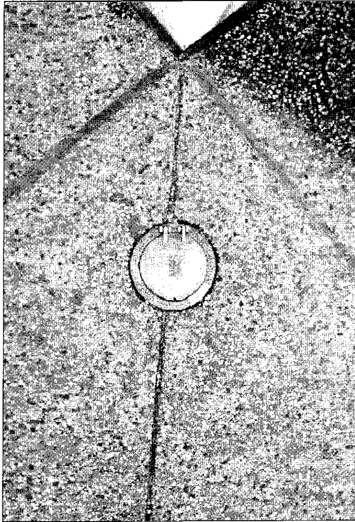
Figure 4.4: Monument Plaza, geodetic control mark access cover at corner of monument.
