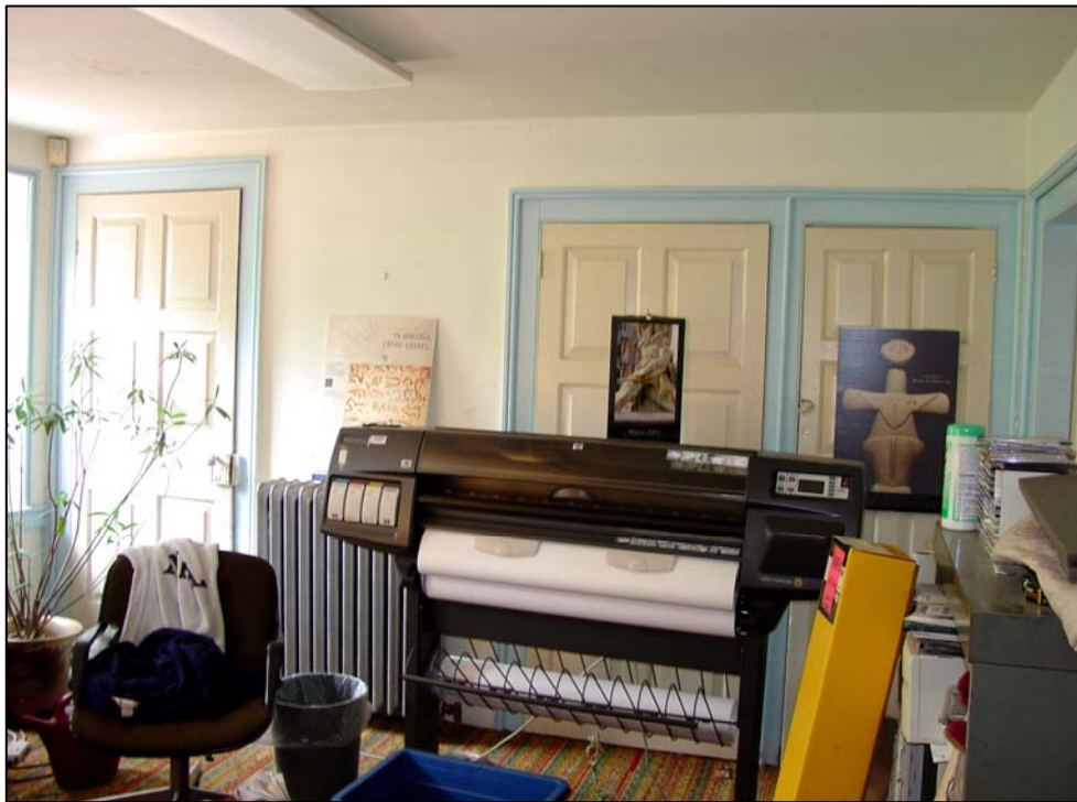
Figure 76. Room 205 (northeast bedroom), east wall, showing three doorways in their original locations. Left to right, they lead to the enclosure for the back stairway to the attic, a large closet (the former location of a back stairway to Room 103), and a small original closet.
