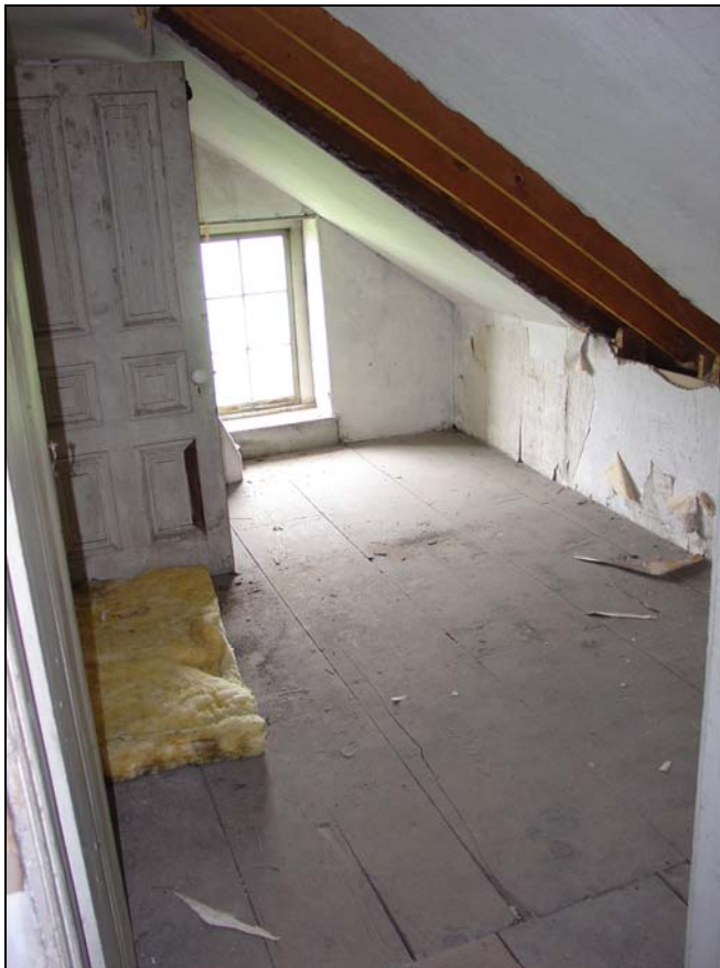
Figure 91. Room 303 (northwest attic room), looking west. At right is an area of ceiling disturbed by the addition of an early 20th- century dormer (removed in 1978). (Note: the door at the right side of the photograph is being stored in the room and is not part of the space.)
