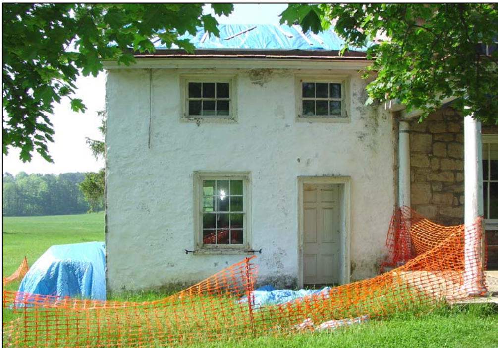
Figure 28. North elevation of the ell during reroofing in 2004.
