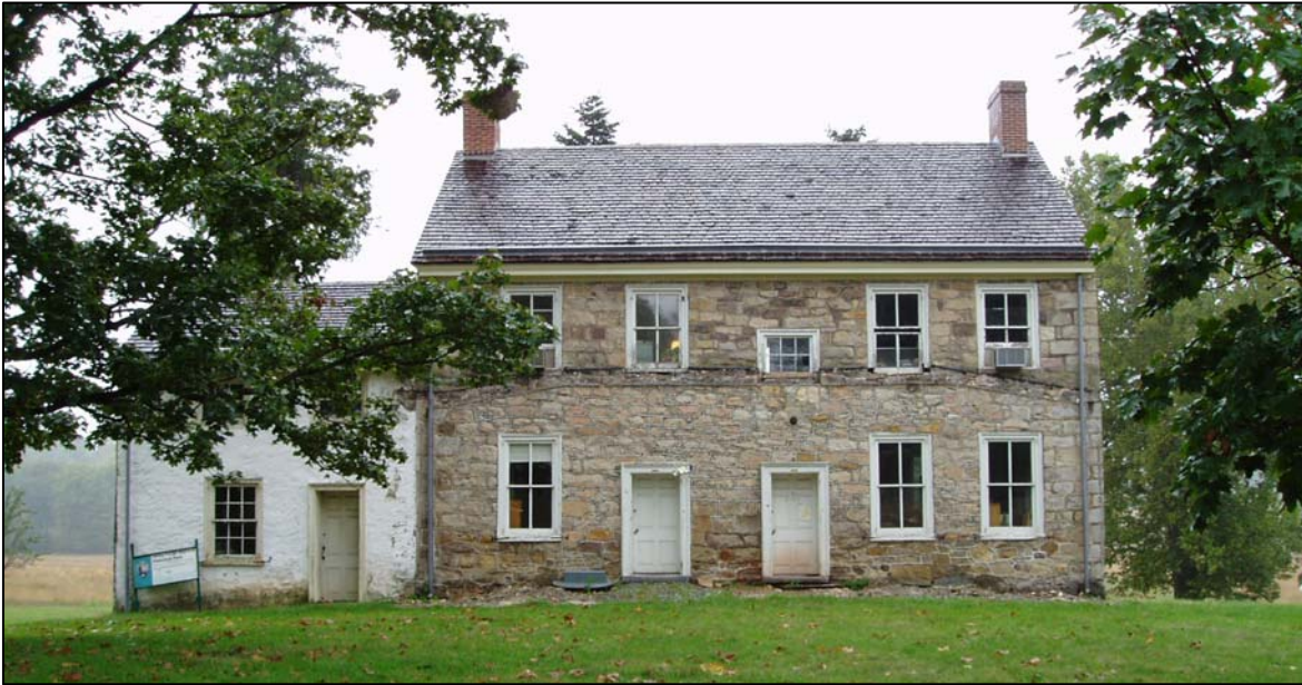
Figure 27. North elevation, showing the two entrances, and the shortened double- hung window that originally illuminated the stair landing.
