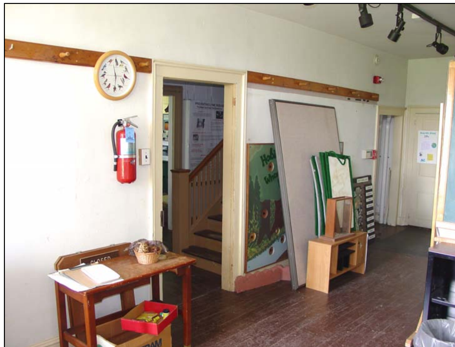
Figure 51. Room 103 (original kitchen), west wall, showing (left to right) the doorway to the center hall, the doorway to the passage to the basement stairway, and the north exterior doorway.
