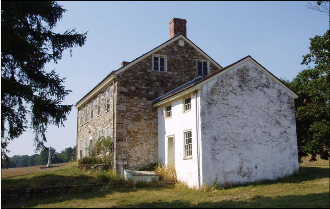
Figure 25. East and south elevations, showing the attic casement sashes, the gable date stone, and the basement bulkhead.
