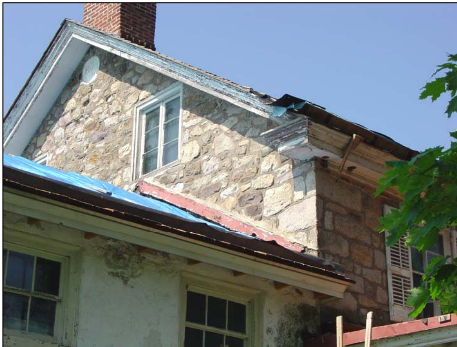
Figure 30. Main house, east end, detail of extended cornice and return. (Photograph taken in 2004.)
