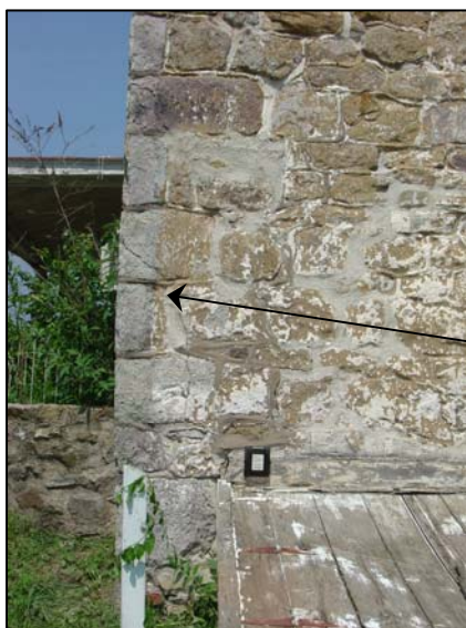
Figure 13. Early v- shaped mortar joint extant at the southeast corner, main house (2004 photograph).
