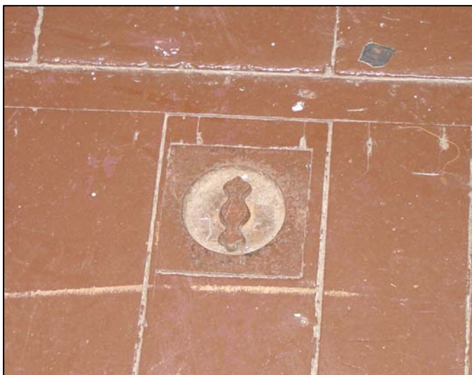
Figure 18. Damper handle set into the floor in front of the first- story fireplace in Room 102 (parlor).
