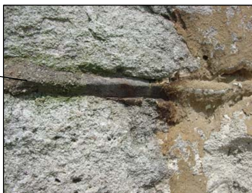
Figure 14. Detail of early v- shaped mortar joint.
