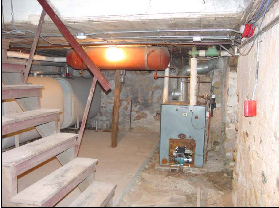
Figure 32. Room 001 (north basement), east side.
