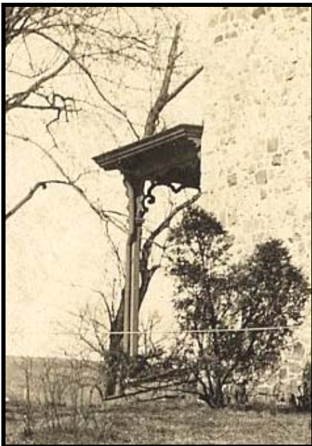
Figure 5. Detail of figure 3: west end of the north (back) porch, showing bracket and porch overhang details that differ from those of the south porches.
