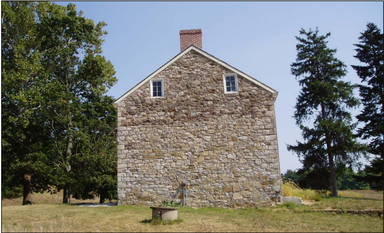
Figure 15. Main house, west elevation, showing the change in masonry partway up the wall.
