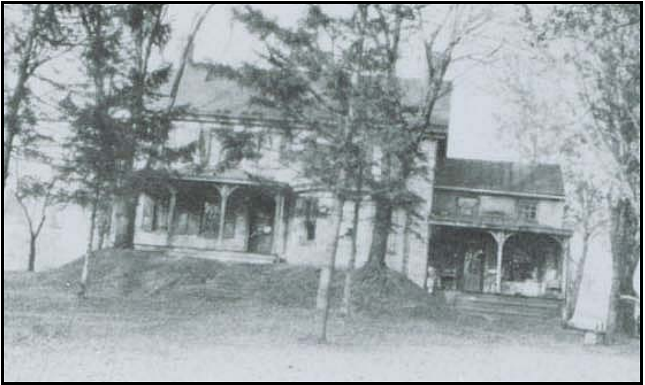
Figure 4. South elevation, showing the early porch and bay window on the main house, and the early porch on the ell, n.d.
