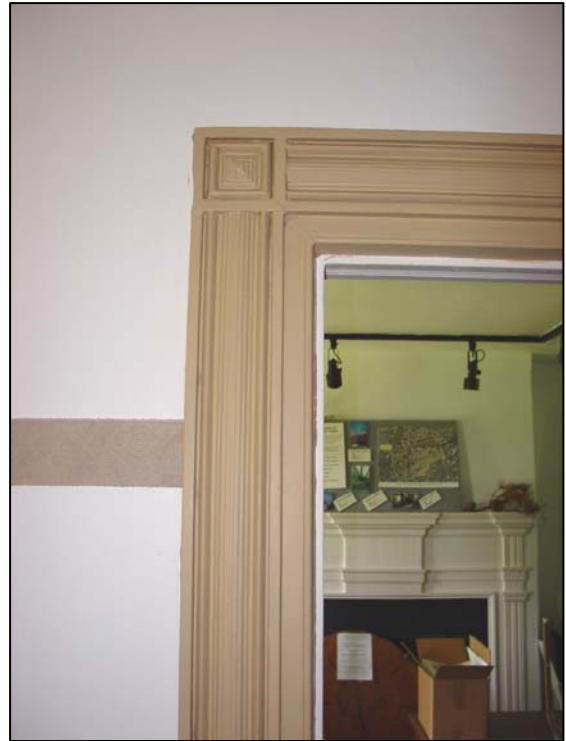
Figure 40. Room 101 (first-story center hall), west wall, reeded casing of a doorway to the parlor.
