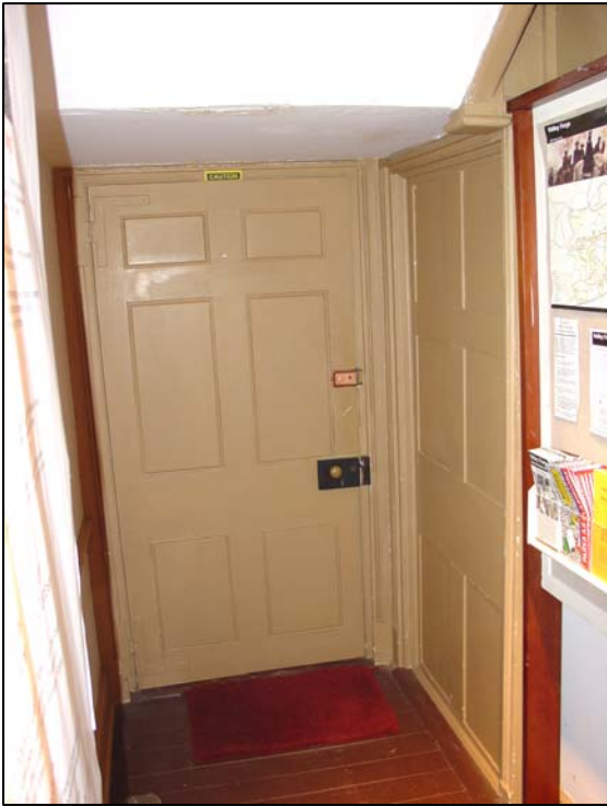
Figure 39. Room 101 (first-story center hall), north exterior doorway. Also shown is the paneling that infills an original doorway to a passage beneath the main stairway, which provided access to the basement stairway and the original kitchen.
