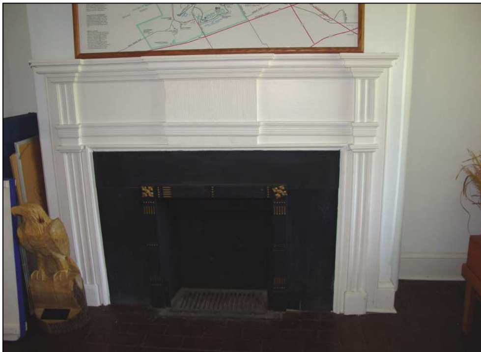
Figure 45. Room 102 (parlor), west wall, showing the north fireplace and mantel.
