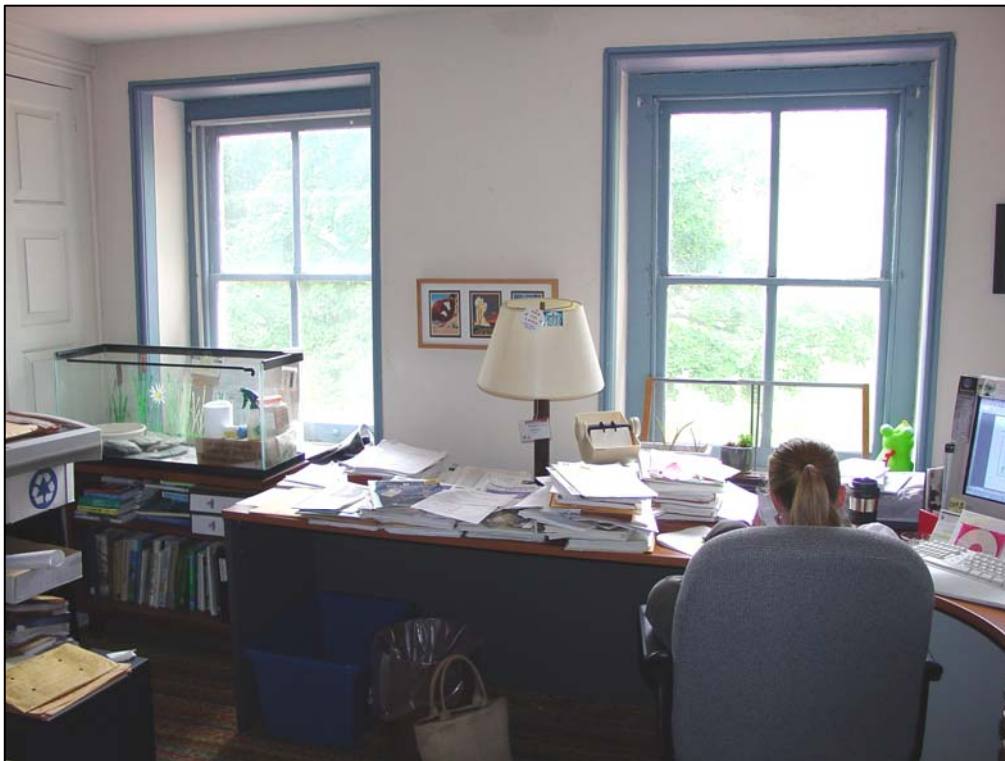
Figure 66. Room 202 (northwest bedroom), north wall, showing the windows with unpaneled reveals.
