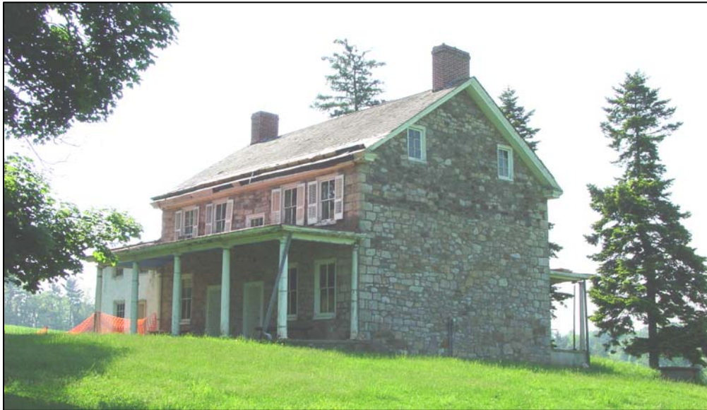
Figure 21. Northwest view of house, showing original second- story blinds still in place.
