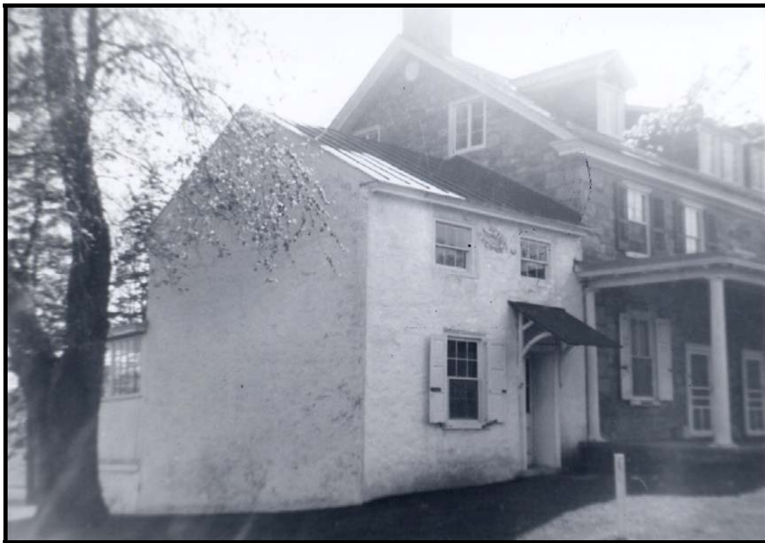
Figure 7. North and west elevations, showing the early doorway hood on the north elevation of the ell, the enclosure of the ell's south porch, and the 20 th - century attic casement sashes.
