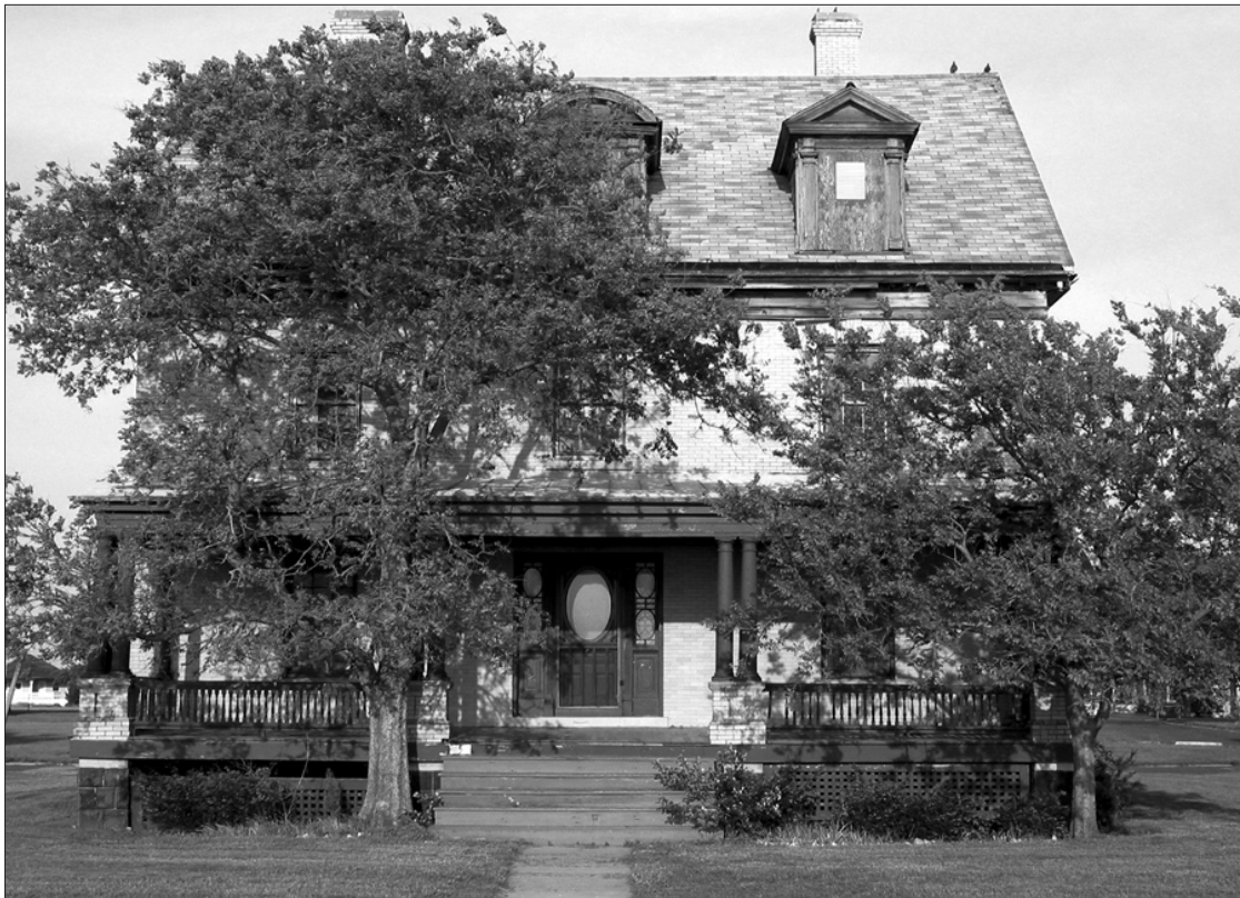
Figure 2.13. Several self-seeded trees have been allowed to mature along side the front porches of Officers Row. These should be removed. OCLP, 2004.
