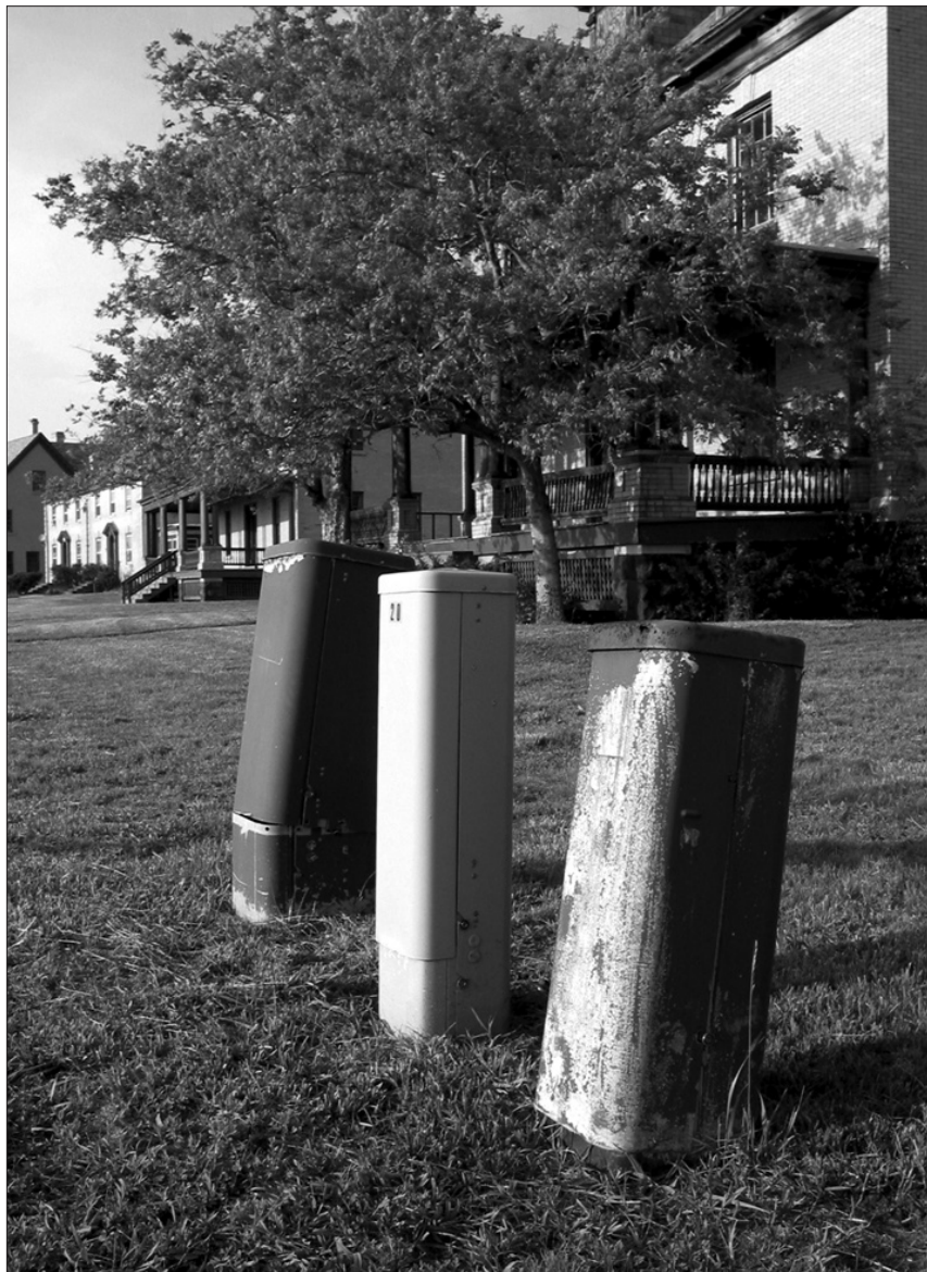
Figure 2.4. Above ground utility boxes are located throughout the study area, notably between the buildings of Officers Row, as pictured above. These fixtures should be located to one side of the gap between Officers Row quarters or underground, rather than in the center of the open space. OCLP, 2004.
