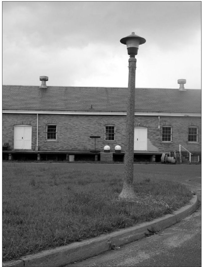
Figure 2.22. A surviving concrete streetlight in the vicinity of Sergeants Row. OCLP, 2005.
