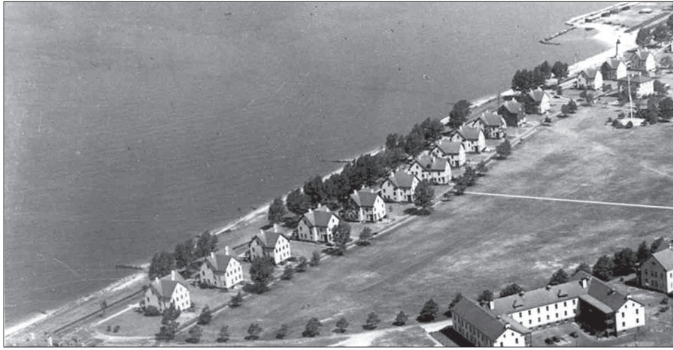
Figure 2.14. 1930 aerial photo shows the inconsistent street tree coverage along Hartshorne Drive that was typical throughout the period of significance. September 1930, National Geographic aerial photograph of Fort Hancock. Copy in Gateway NRA Museum Collection, Catalogue #833.
