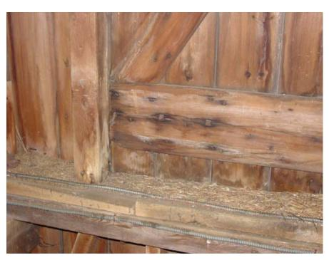
**Figure 15.** New Barn, east- elevation loft door, lower rail depicting extant fasteners for strap hinge, view from interior of barn attic (2005).
