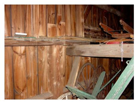
**Figure 20.** New Barn, east- elevation framing, interior view of intermediate post, plate, bridging beam (attached to plate), and 2 by 6 framing, 2005.
