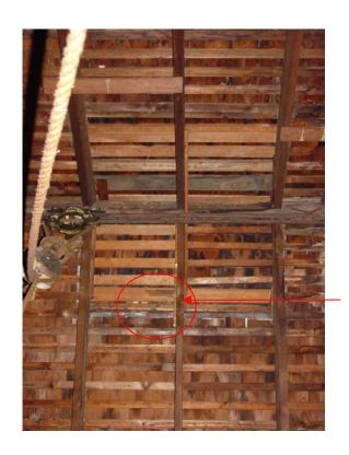
Figure 29. New Barn, interior view of roof framing and extant evidence of barn cupola, note change in sheathing and extant cupola flashing (2005).
