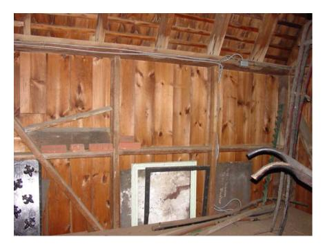
**Figure 21.** New Barn, north- elevation framing, interior view of northeast section showing 2 by 6 studs, blocking and bracing, plate, and corner post (2005).
