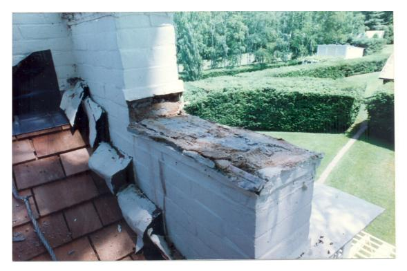
Figure 58. Aspet, deteriorated condition of brick parapet caps, 1993.
