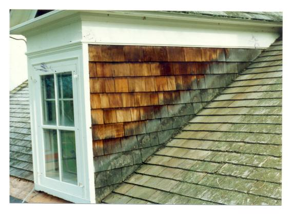
Figure 59. Aspet, dormer showing mold and water damage to shingles; mold and moss also covers adjacent roof shingles, 1993.
