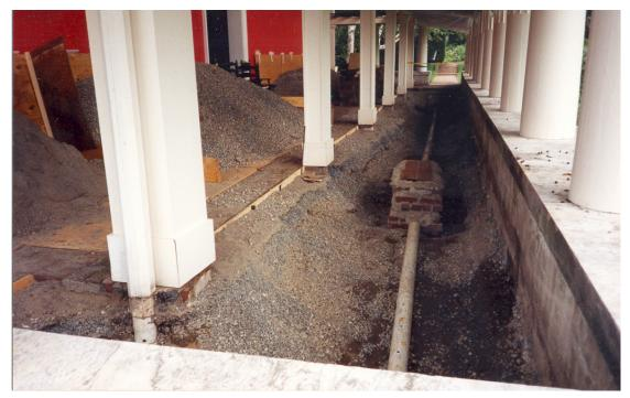
Figure 105. Little Studio, drainage project at south elevation: brick and rock removed to prepare for drain, 1994.
