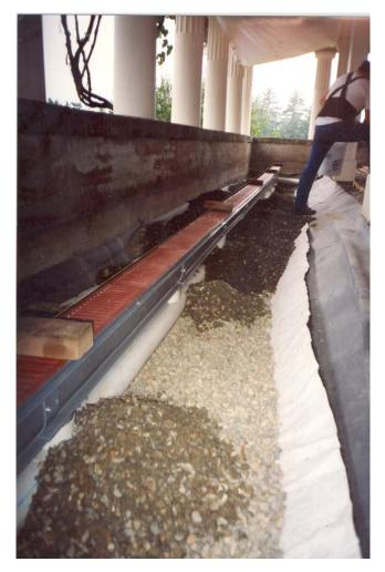
**Figure 107.** Little Studio, drainage project: installation of fabric drain and rock along south elevation, October 1994.
