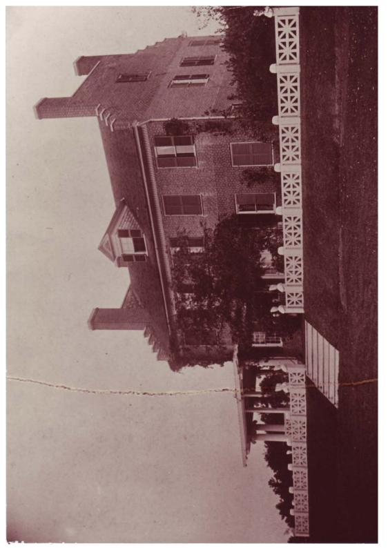
Figure 8. View of Aspet, south elevation, circa 1893, showing west piazza and dormers in place, and gable end walls stepped. View predates east piazza and paint on brick walls.
