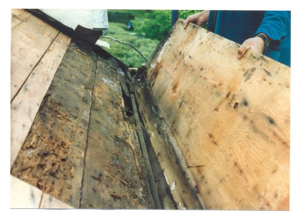
Figure 57. Aspet, rotten sheathing boards exposed, 1993.
