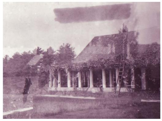
Figure 65. Barn Studio, west end of south elevation, showing rustic poles replaced with columns, circa 1900.
