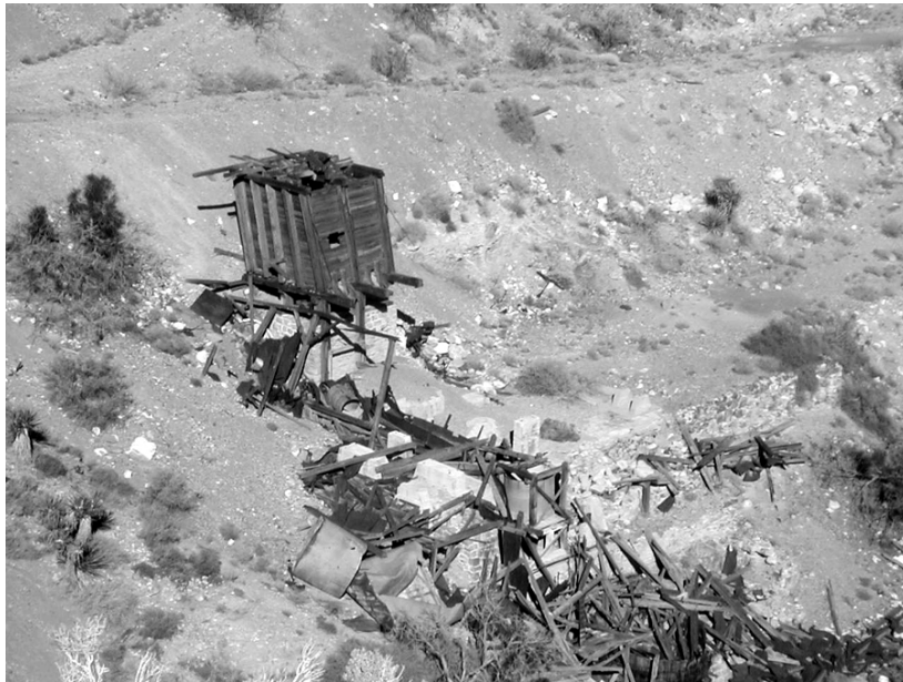
Figure 2 Hundreds of abandoned mines dot the Mojave landscape and although many items have been taken by looters over the years, numerous mining artifacts are included in the collections. The Bonanza King Mine, shown here, dates to the late 1880s.
