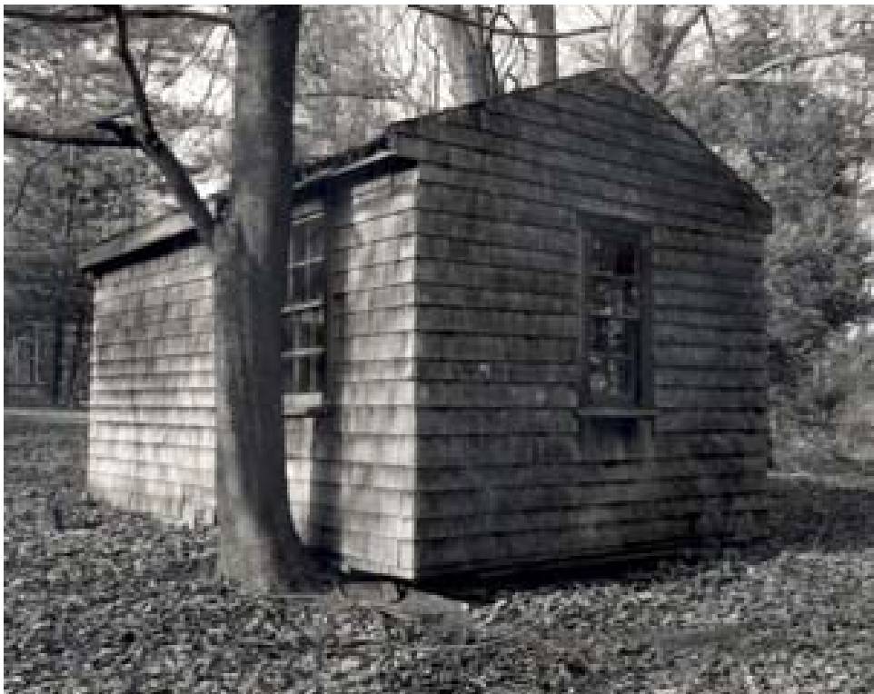
Figure 42. Tool House, views looking southeast and northwest, November 10, 1993.
