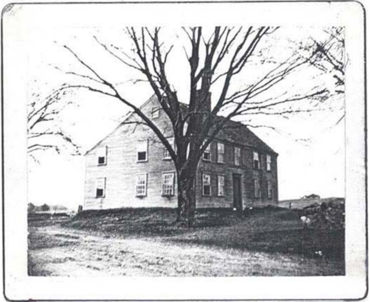
Figure 10. Meriam House exterior, view looking northeast, circa 1900.
