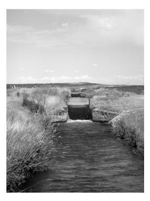
Figure 36. Canal drop in section 6 on lateral 21.3 from Milner-Gooding canal to camp. (Western Archeological and Conservation Center)
