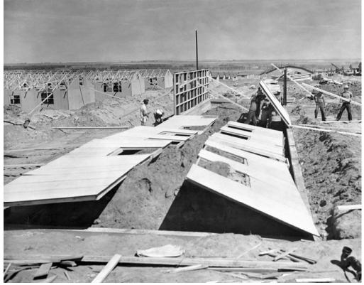
Figure 18. Typical scene of barracks construction with prefabricated section lying in position. (Denver Public Library, Western History/Genealogy Dept., X-6571)
