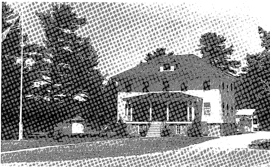
Fig. 5.4. Munising's Coast Guard Station was built in 1931, and currently serves as headquarters for the Pictured Rocks National Lakeshore. NPS photo.
