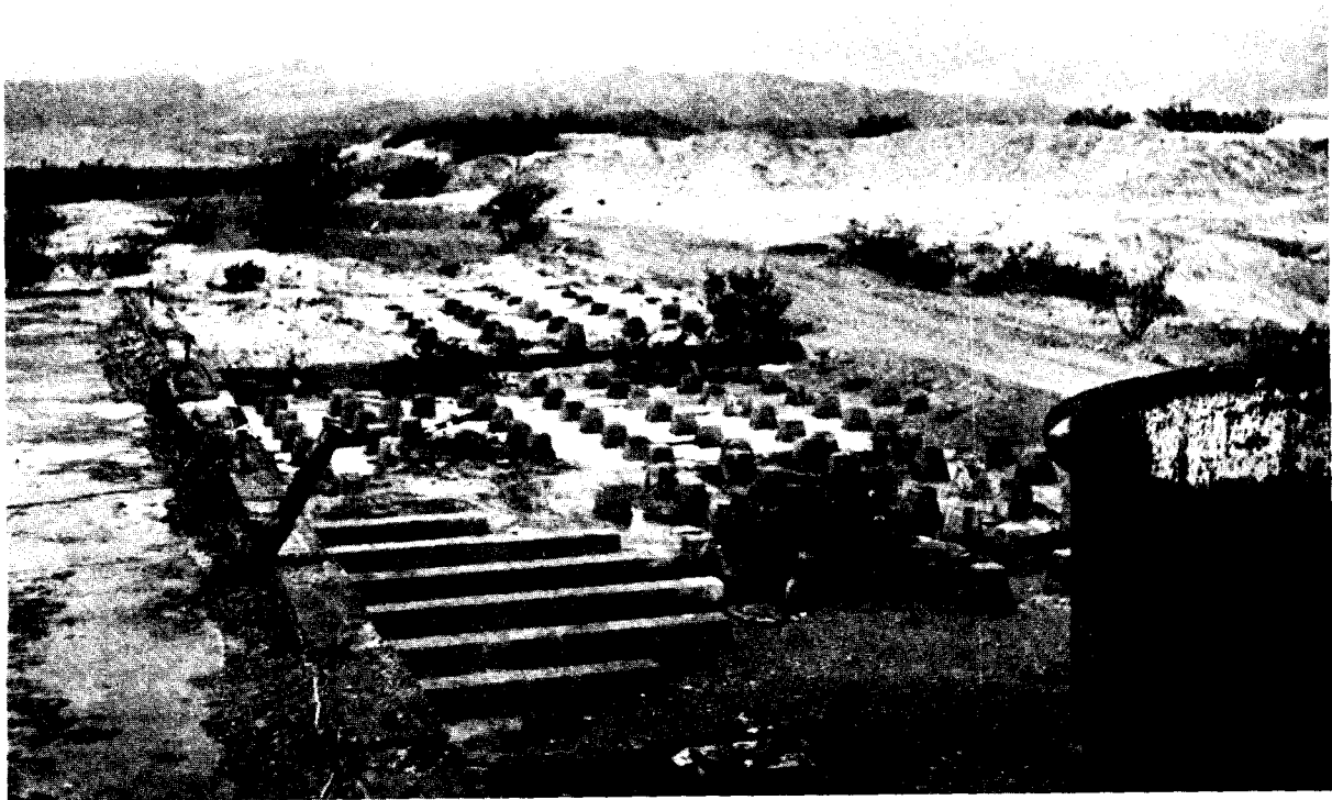
Plate 10. Katherine Mill Site. Foundations for tanks and vats.
