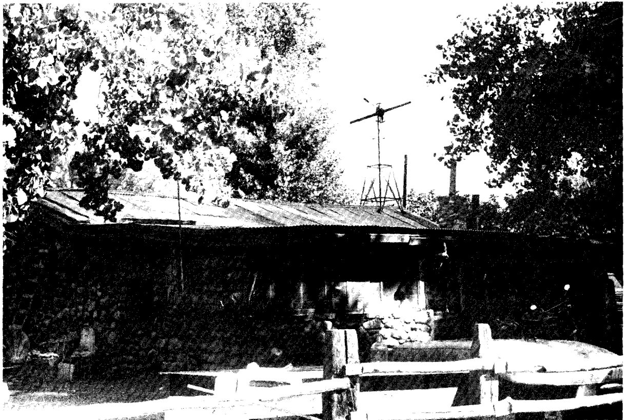
Plate 16. Tasi. Main house built by Ed Yates in 1938.
