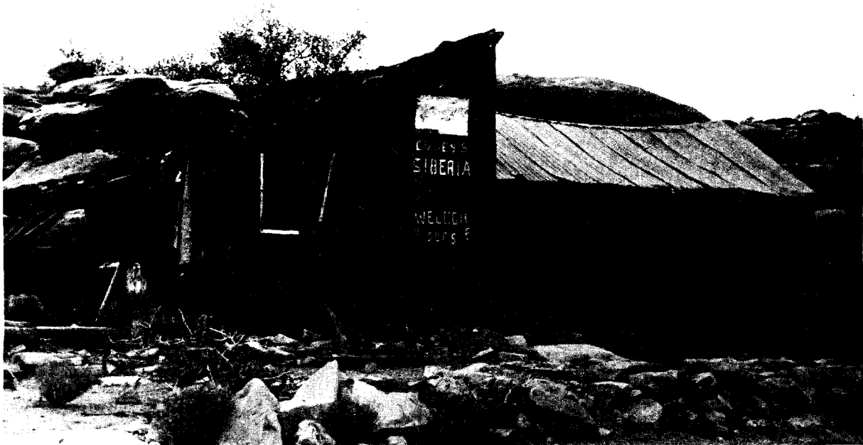
Plate 6. Copper Mountain Mine. Shack nestled into bedrock. Typical board and batten construction and corrugated iron roof.
