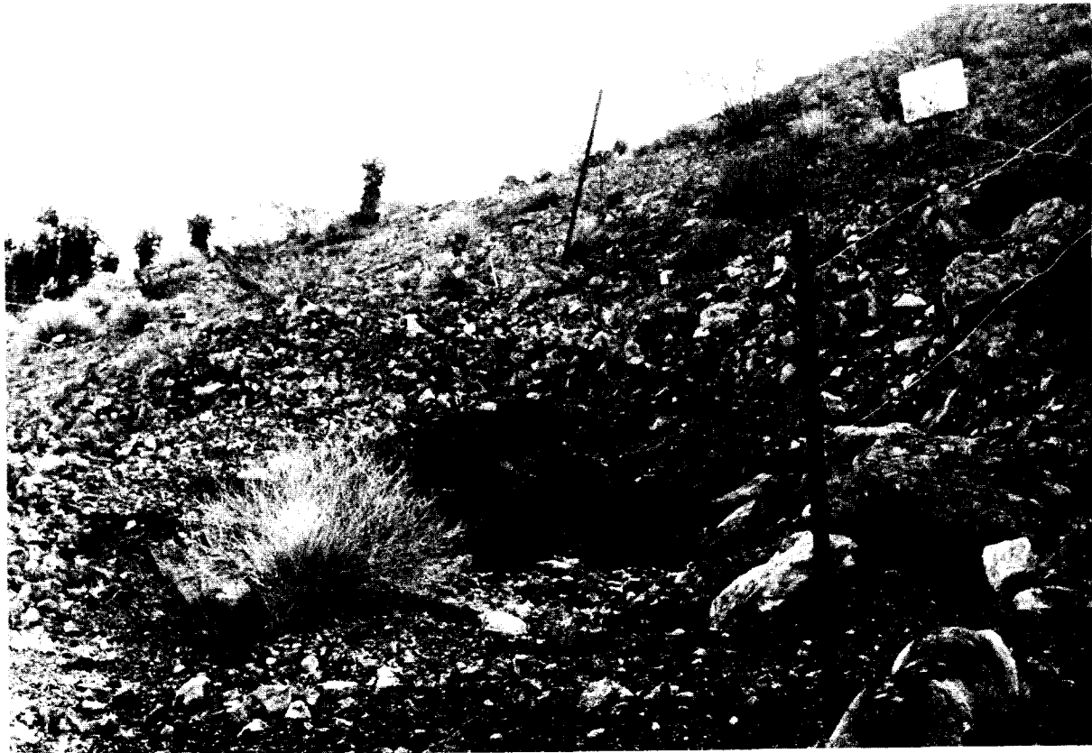
Plate 1. Old Pope Mine. This collapsed, inclined shaft is in hazardous condition typical of many LMNRA mines.
