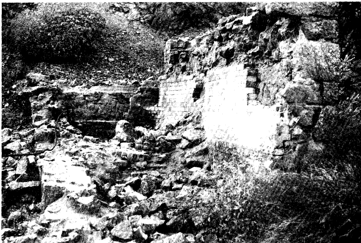
Plate 12. Homestake Mine. Boiler foundation.
