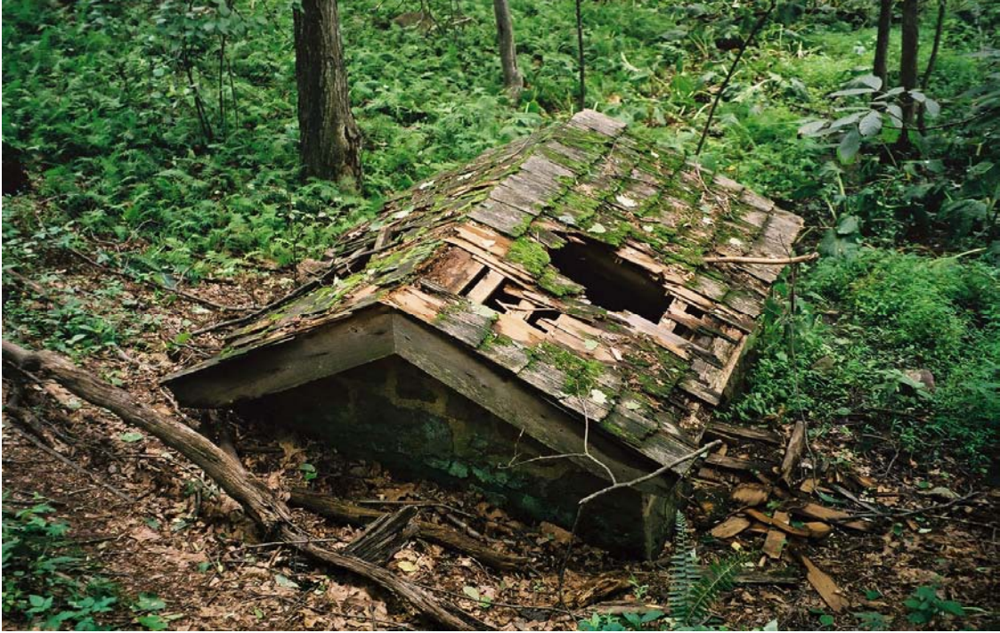
Figure 20 – CCC-constructed springhouse near Baptism Creek Picnic Area. (Robinson & Associates photograph, 2003.)
