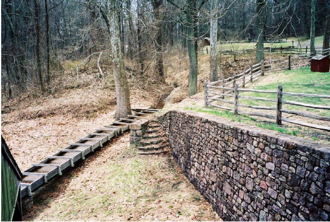
Figure 3 – The reconstructed West Head Race, originally built circa 1805. (Robinson & Associates photograph, 2003.)
