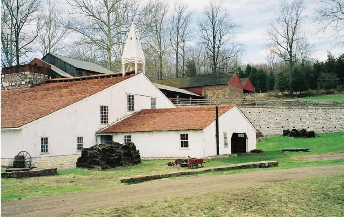
Figure 4 – The reconstructed furnace complex at Hopewell, including the Cleaning Shed, Cast House, Molding Sheds, Furnace Stack, Bridge House, Wheel House, Connecting Shed, and Charcoal House. (Robinson & Associates photograph, 2003.)
