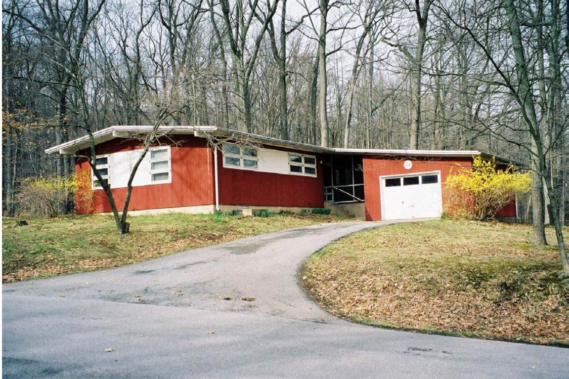
Figure 23 – Quarters 99, constructed during the Mission 66 program. (Robinson & Associates photograph, 2003.)
