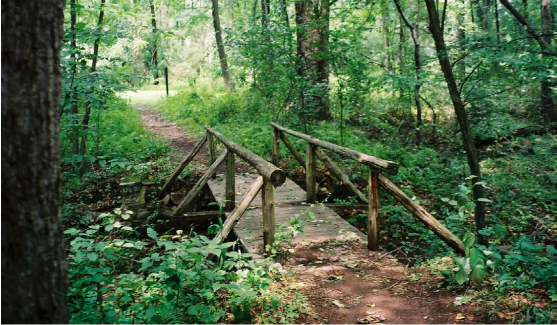
Figure 19 – CCC-constructed vehicle bridge near Baptism Creek Picnic Area, now supporting a pedestrian bridge. (Robinson & Associates photograph, 2003.)
