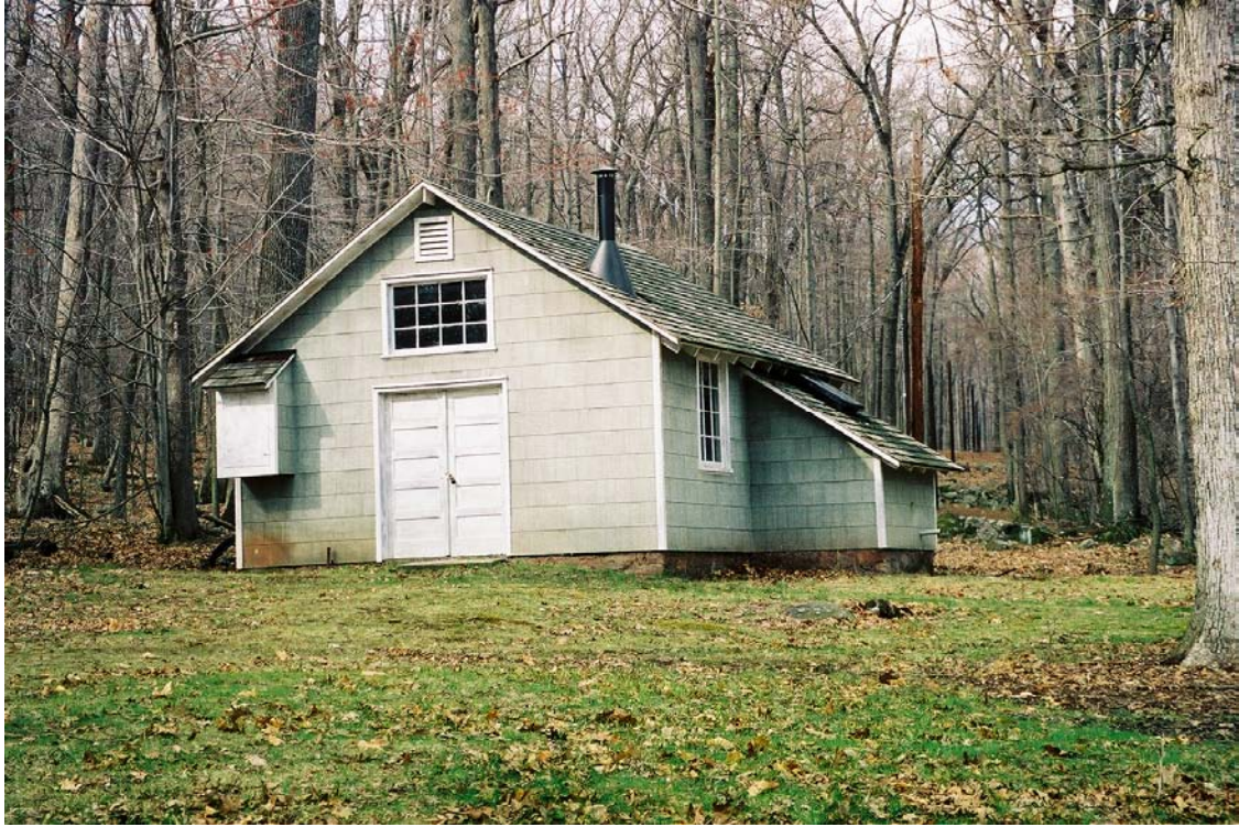
Figure 16 – Civilian Conservation Corps Pump House. (Robinson & Associates photograph, 2003.)
