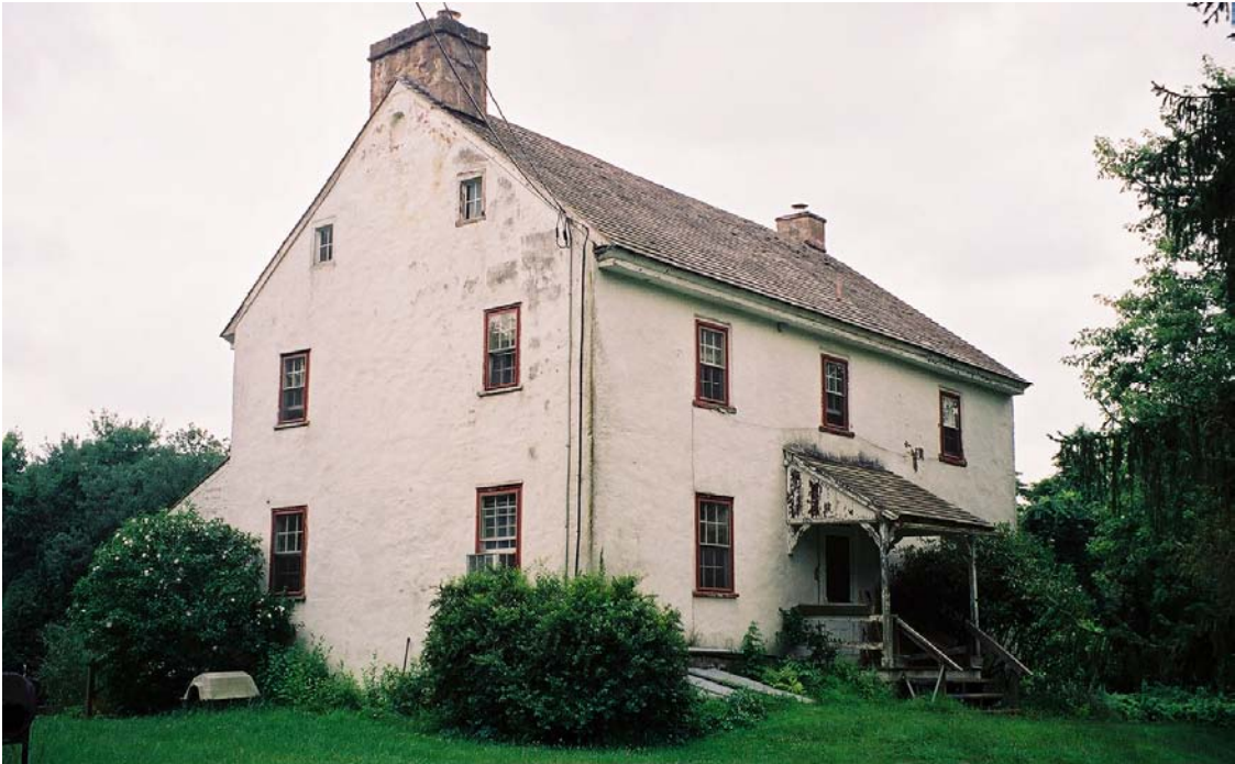
Figure 10 – The Thomas Lloyd House, now used as a residence for a park employee. (Robinson & Associates photograph, 2003.)
