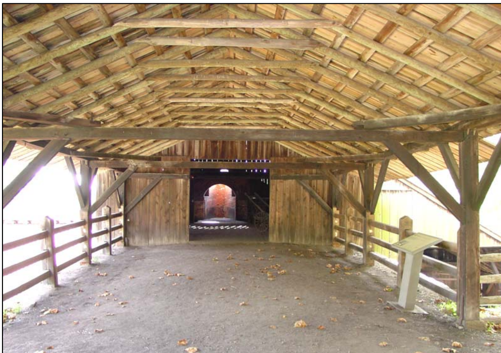
Figure 90. Interior view of the connecting shed, looking south towards the enclosed bridge house, September 2006.
