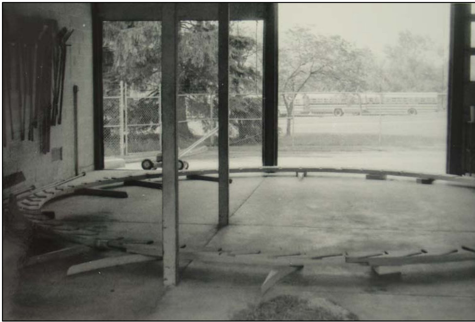
Figure 71. Construction of new water wheel, May 30, 1978.
