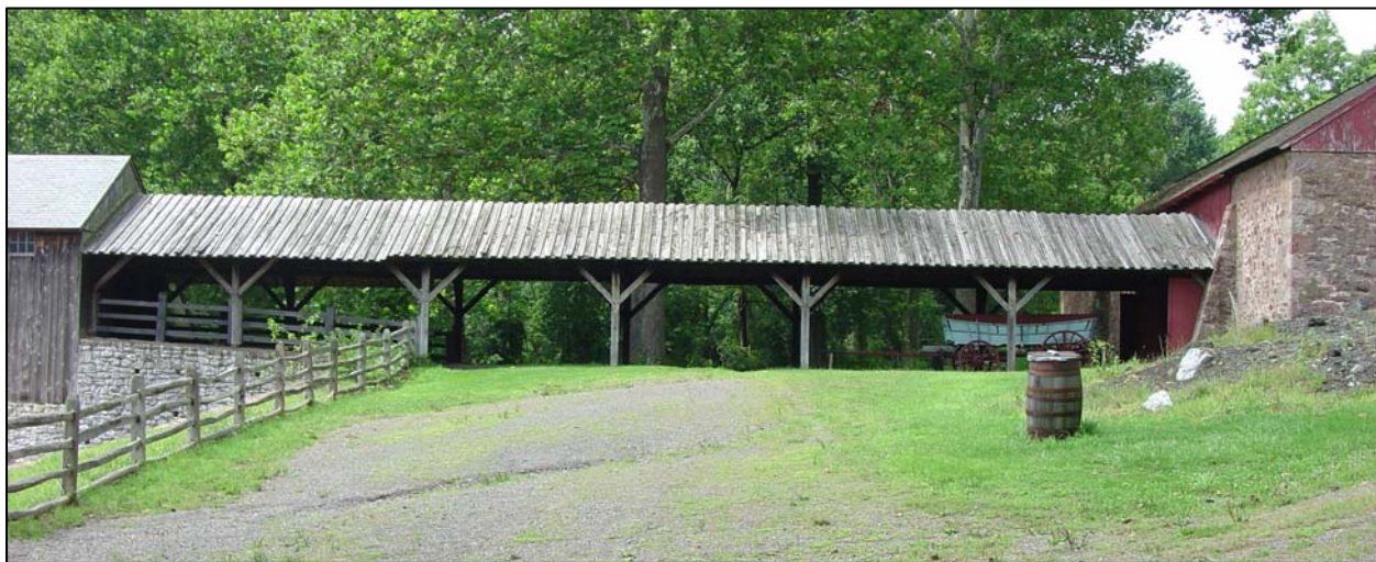
Figure 86. East elevation of the connecting shed, July 2006.
