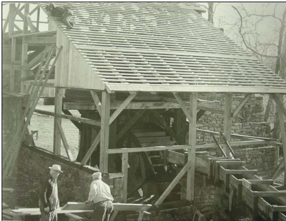
Figure 50. Reconstruction of the wheel house, November 7, 1957.
