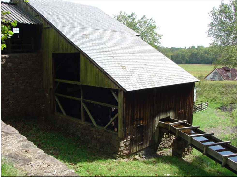
Figure 101. North and west elevations of the wheel house, September 2006.
