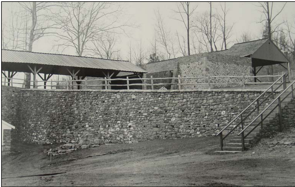
Figure 65. South and east elevations of the charcoal house following demolition of the roof and south extension, June 1965.
