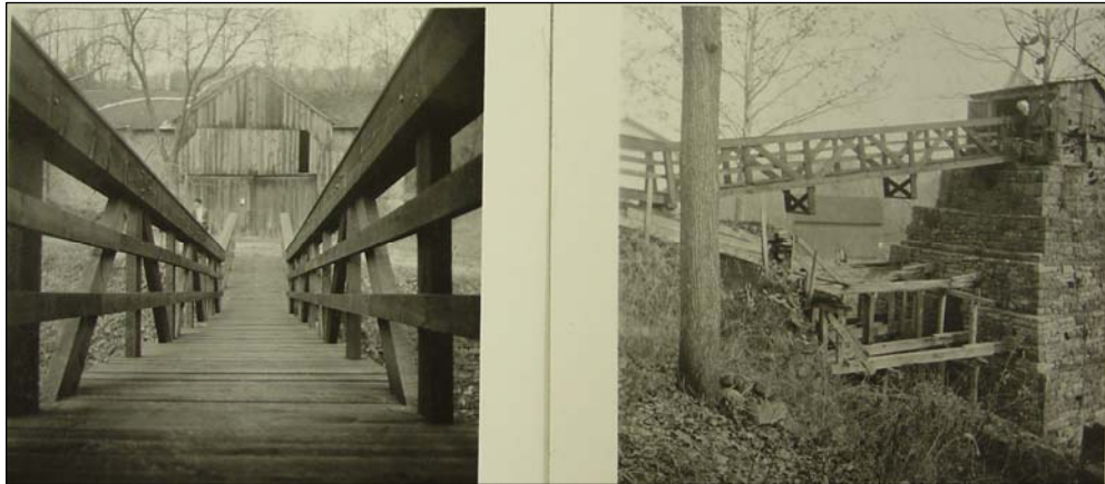
Figure 39. New “temporary” furnace walkway, November 7, 1947.
