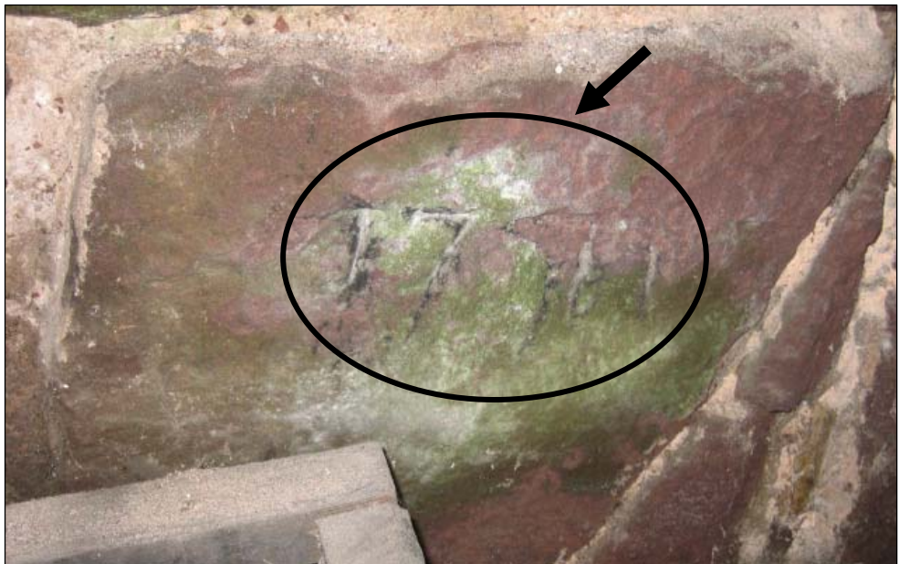
Figure 80. Detail of carved date "1771" on the south side of the cast arch, September 2007.
