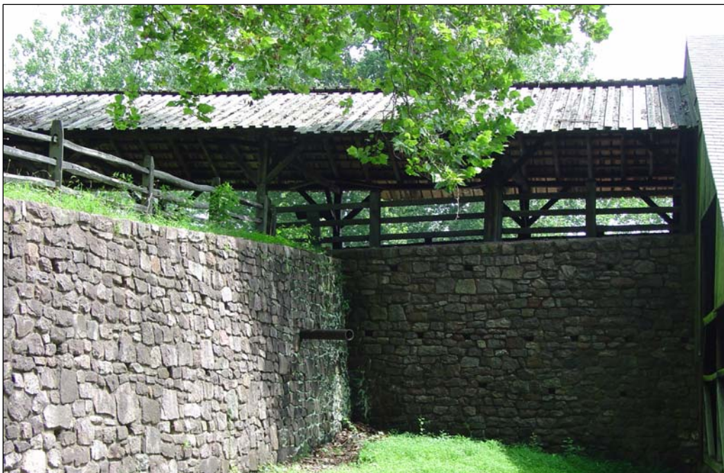
Figure 88. West elevation of the connecting shed, July 2006.
