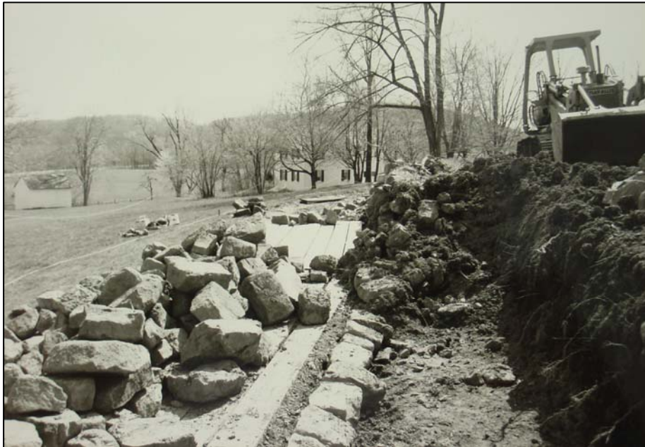
Figure 72. Wall restoration at the east head race, on the west side of Route 345, spring 1984.
