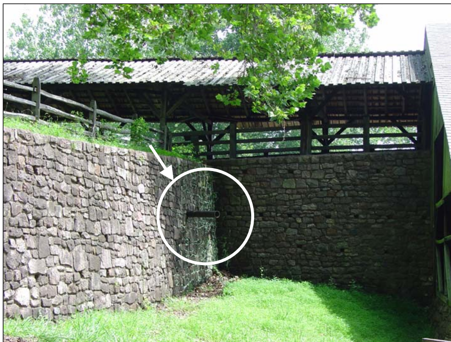
Figure 105. Truncated pipe (at arrow) that conveyed water from the east head race to a wooden flume (now missing) north of the water wheel, July 2006.
