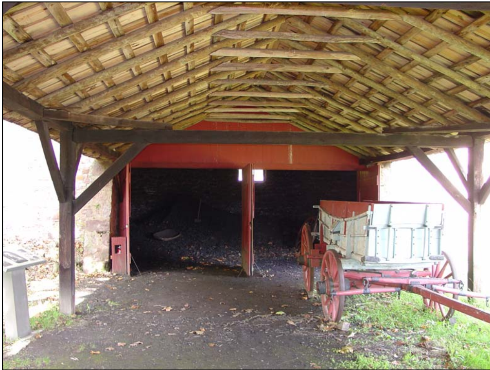
Figure 89. Interior view of the connecting shed, looking north towards the charcoal house, September 2006.
