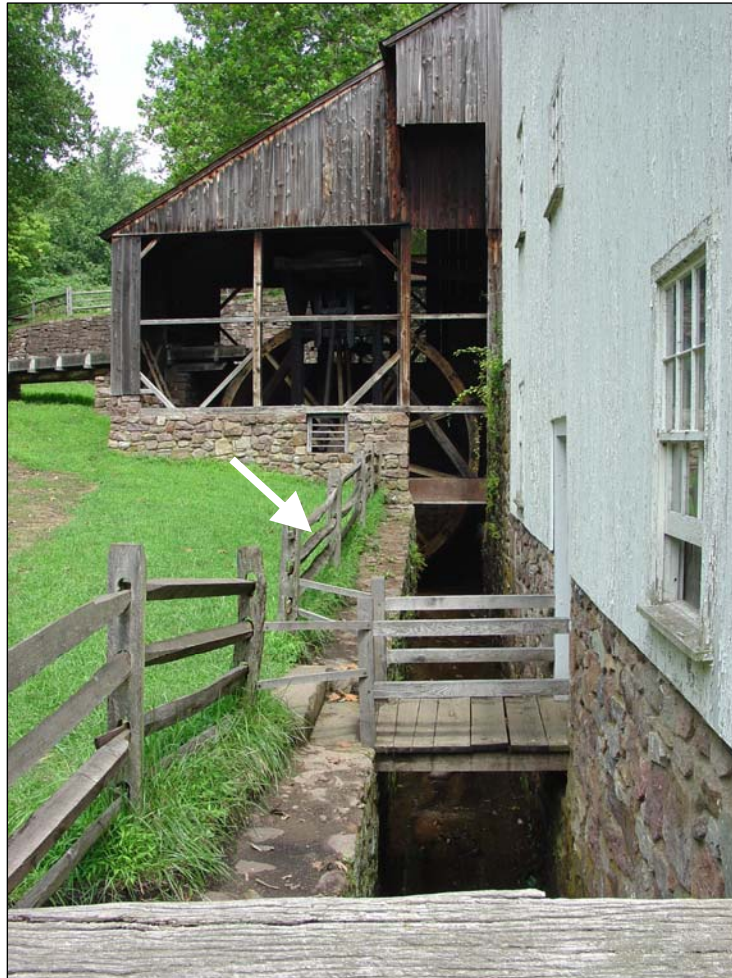
Figure 109. Open portion of the tail race (at arrow), on the west side of the cast house, July 2006.
