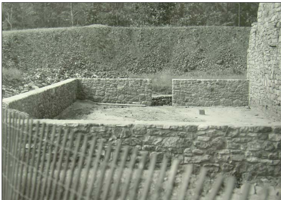
Figure 58. Rebuilt stone foundation walls of the cast house, south of the furnace, October 1962.
