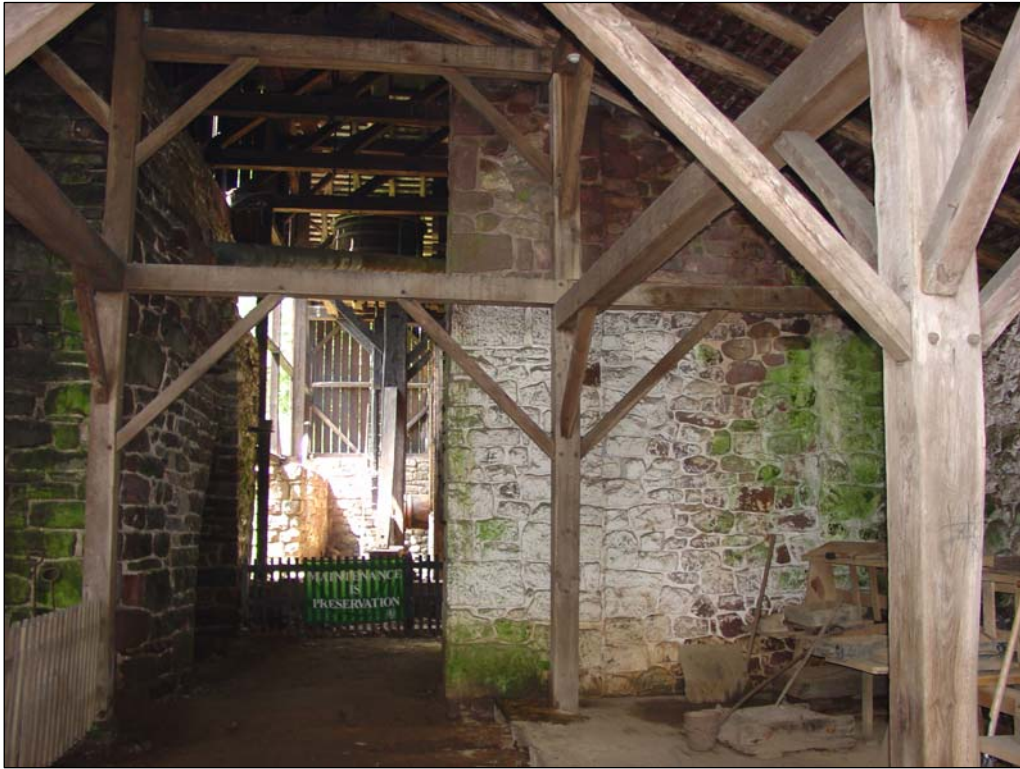
Figure 116. Interior north side of the cast house, view looking west, July 2006.
