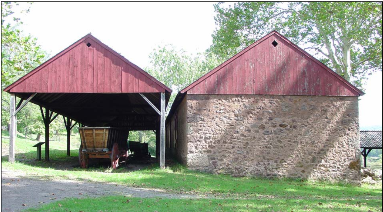
Figure 97. West elevations of the charcoal house (right) and cooling shed (left), September 2006.
