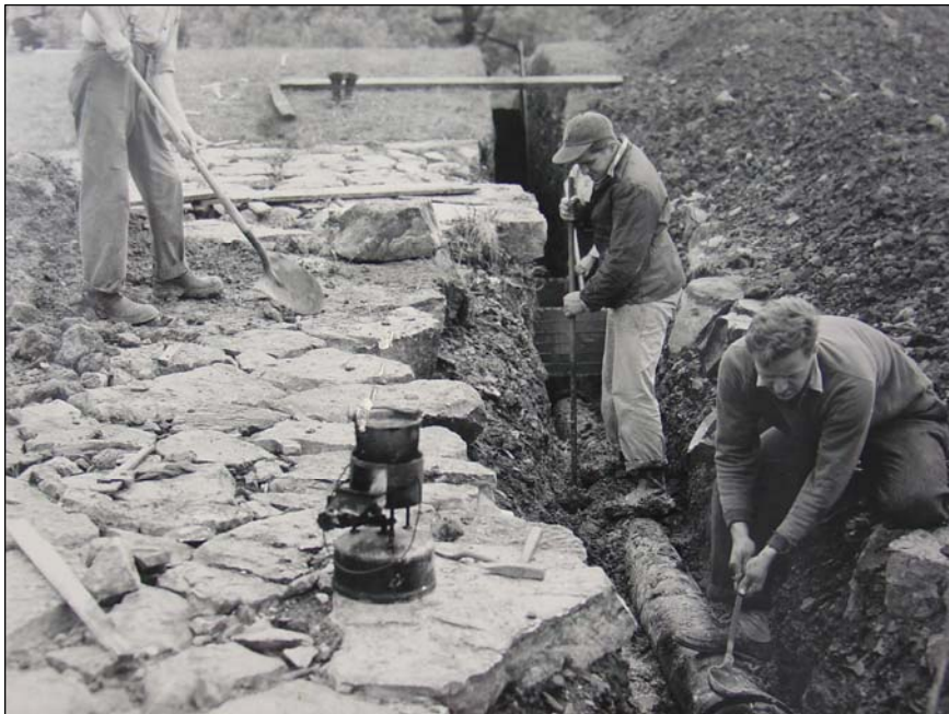
Figure 45. Work on the new underground pipe for the west head race, May 25, 1951.
