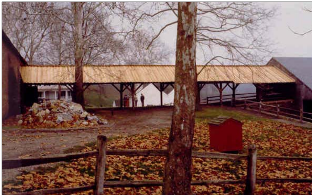
Figure 70. New roof on the connecting shed, Nov. 11, 1977.
