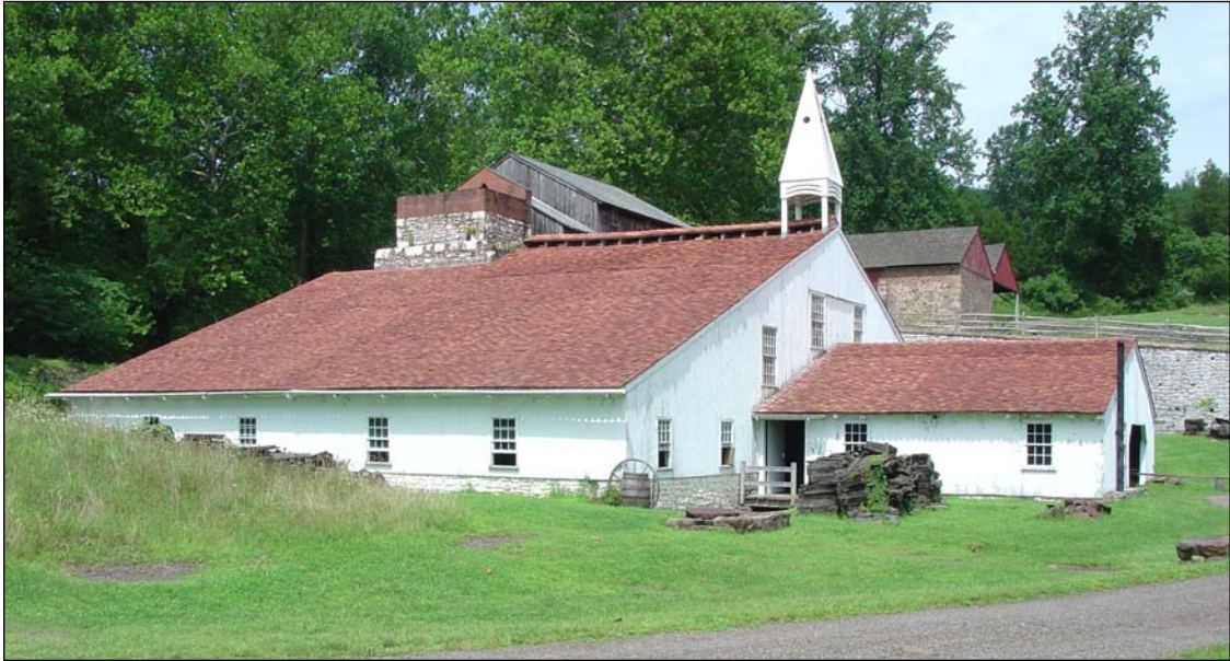
Figure 112. South and east elevations of the cast house and east shed, July 2006.
