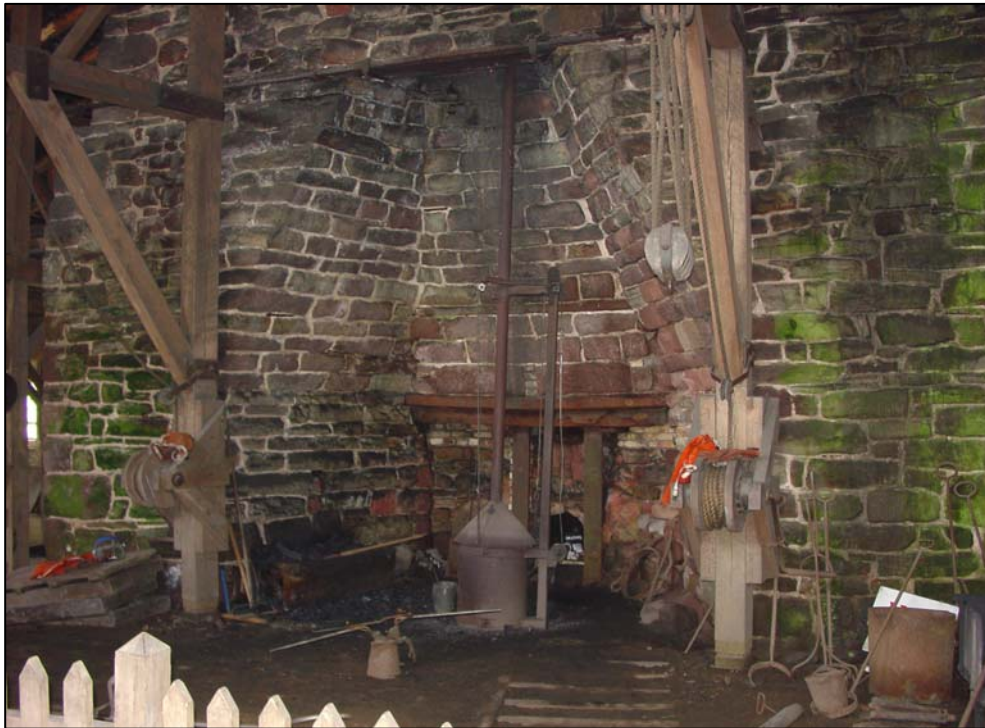
Figure 79. Cast arch on the east side of the furnace, July 2006.
