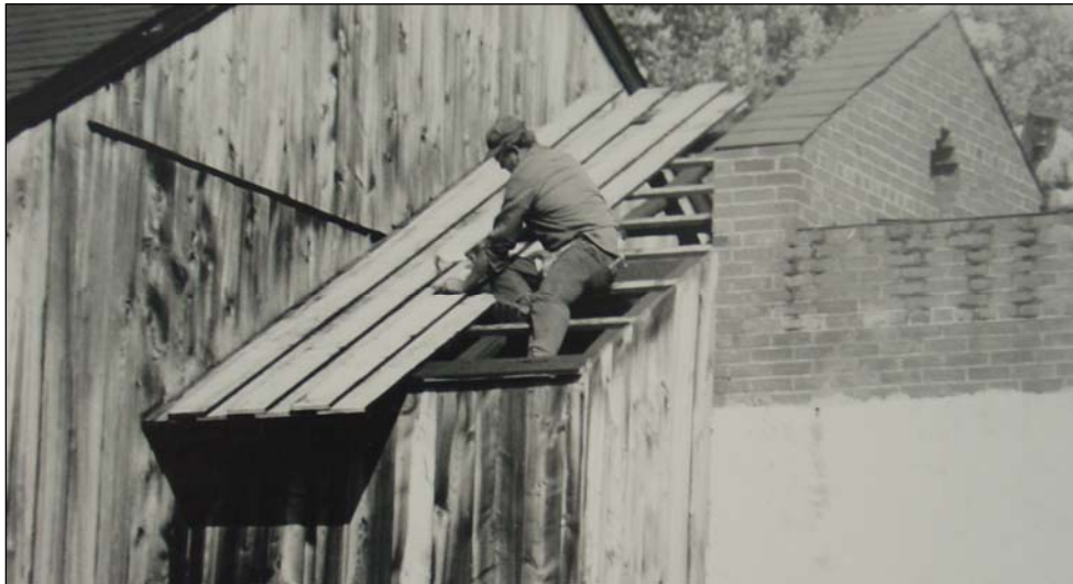
Figure 69. Reroofing the tunnel- head vestibule of the bridge house, November 1971.
