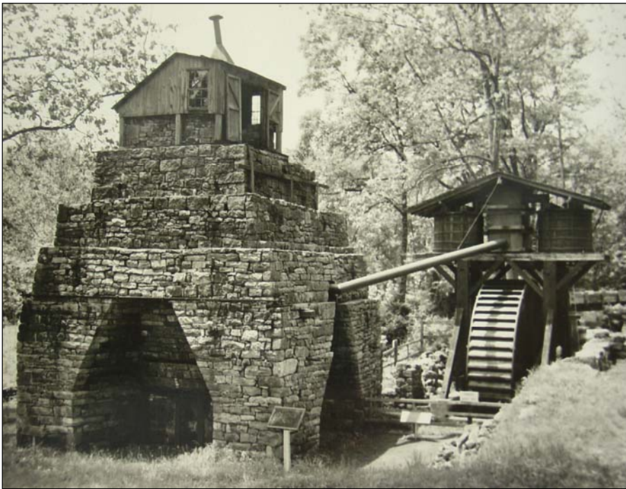
Figure 44. The completed water wheel and blast machinery with temporary roof, June 25, 1952. Note that the furnace walkway had been removed for this project and was not reinstalled.
