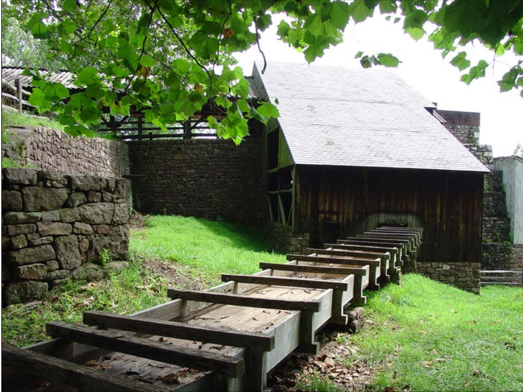
Figure 107. Flume of the west head race, view looking east towards the wheel house, July 2006.
