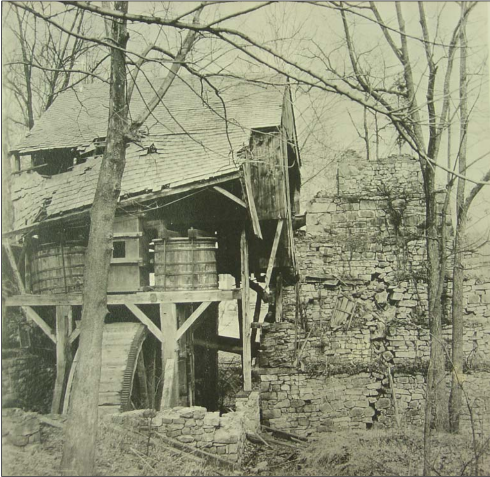
Figure 22. The wheel house and west elevation of the furnace, circa 1925.
