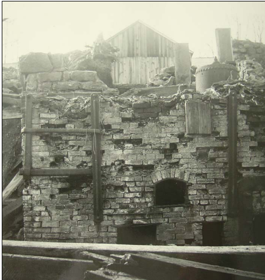
Figure 41. South brick wall enclosing the steam boiler prior to dismantling, 1950. Note also the south extension of the charcoal house in the background.
