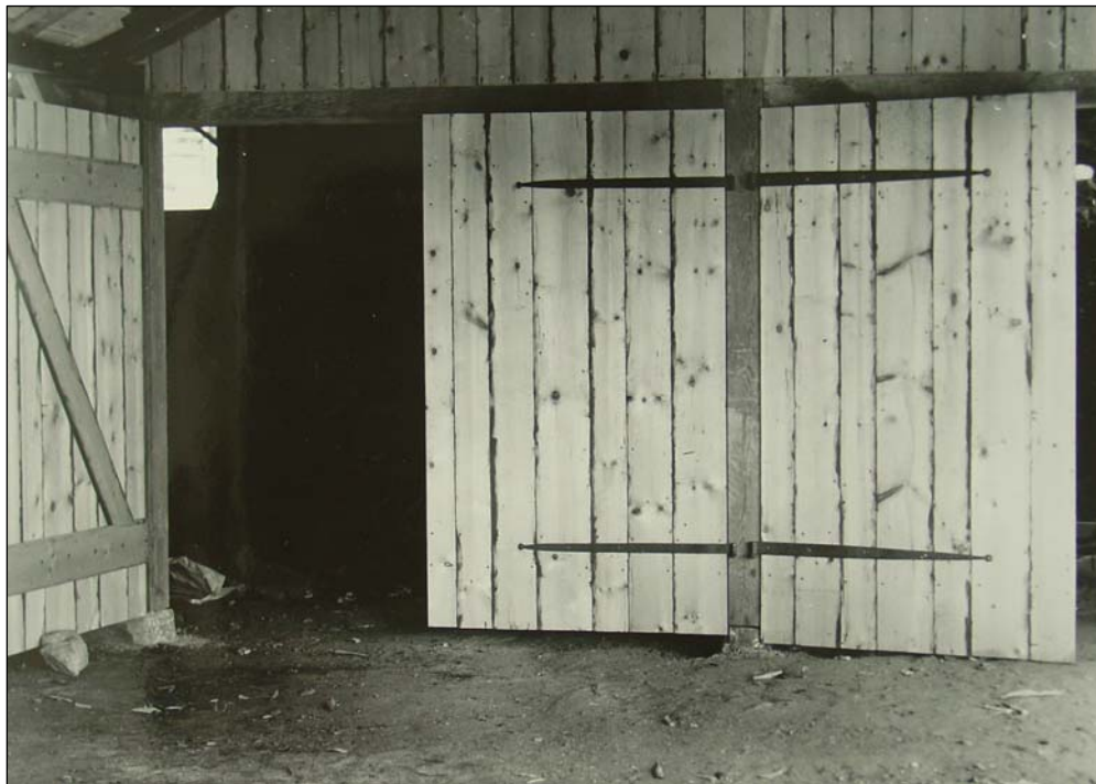
Figure 67. New south doors of the charcoal house, July 1965.
