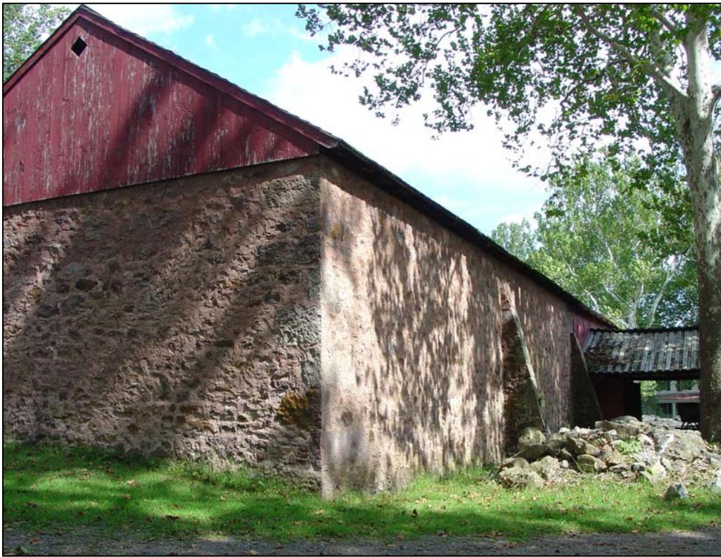
Figure 98. West and south elevations of the charcoal house, September 2006.
