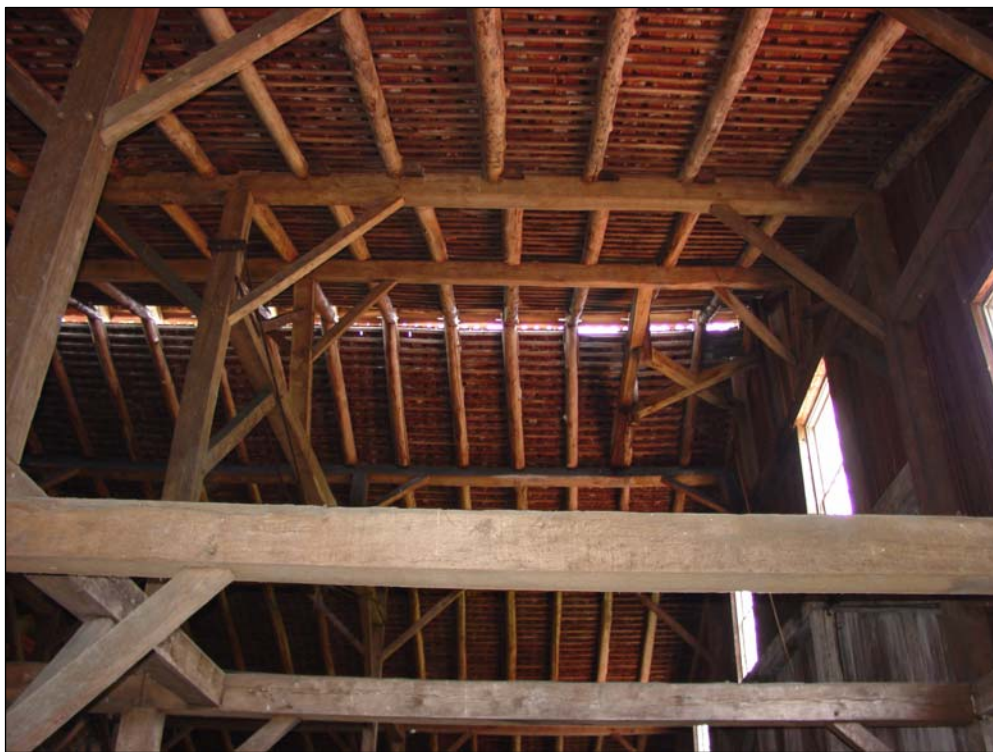
Figure 119. Detail of interior roof framing of the cast house at main ridge, July 2006.
