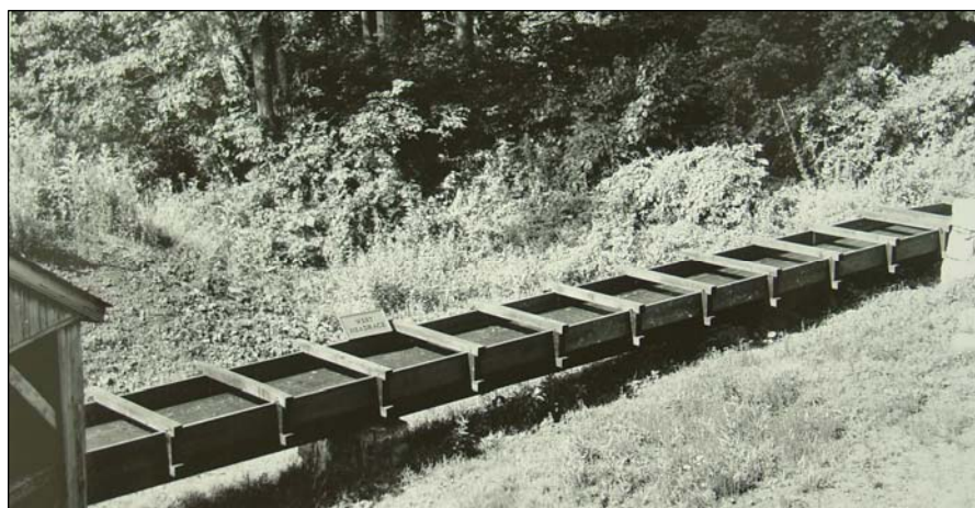
Figure 56. Reconstructed flume of the west head race, July 1964.
