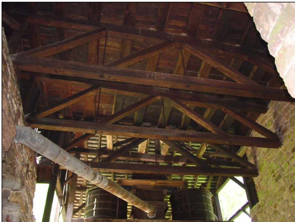
Figure 92. View of floor framing of the enclosed bridge house and tunnel-head vestibule, looking west, July 2006.
