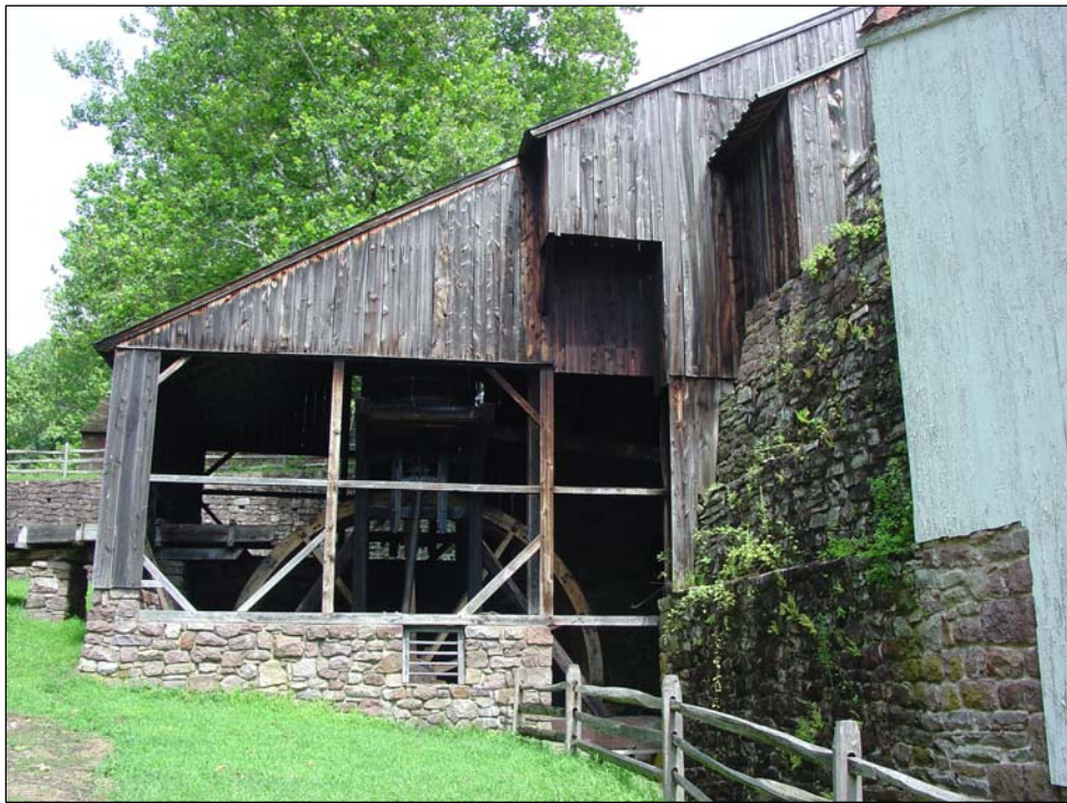
Figure 102. South elevation of the wheel house, July 2006.
