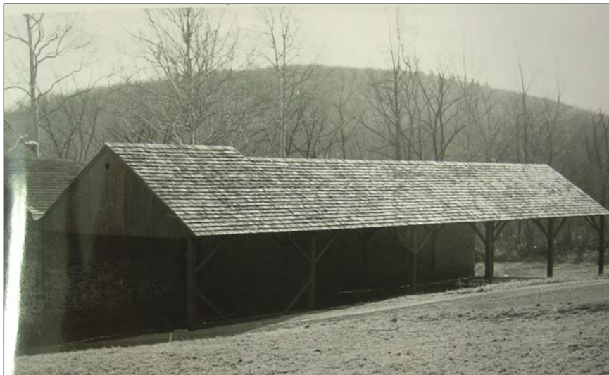
Figure 53. Northeast view of the completed cooling shed, November 29, 1958.
