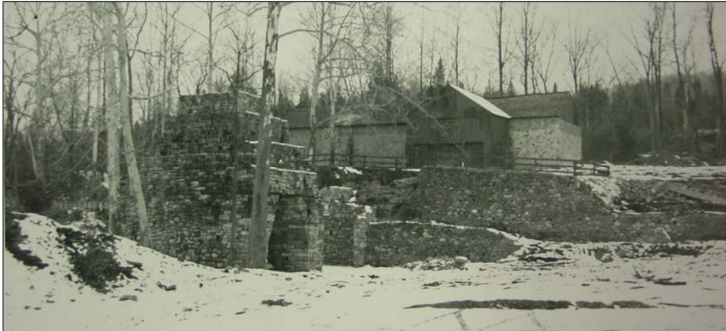
Figure 46. View duplicating the angle of the earliest (1887) photograph following closure of the Warwick- Birdsboro road, December 1955.
