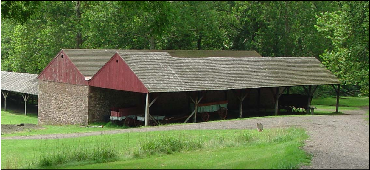
Figure 96. North and east elevations of the charcoal house and cooling shed, July 2006.
