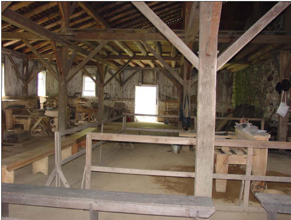
Figure 118. Interior south side of the cast house, view looking west, July 2006.
