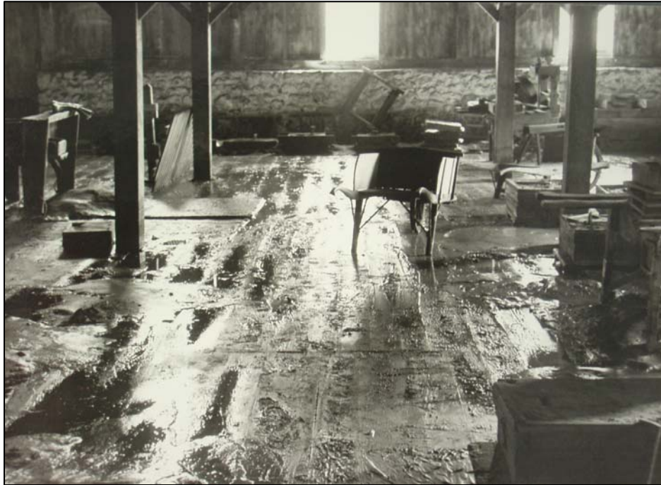
Figure 73. Post- hurricane damage in the cast house, 1987.
