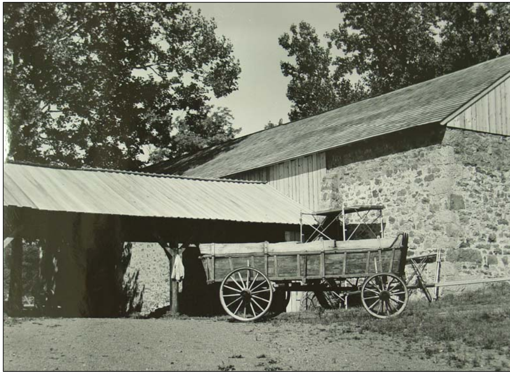
Figure 66. South and east elevations of the partially completed charcoal house, July 1965.
