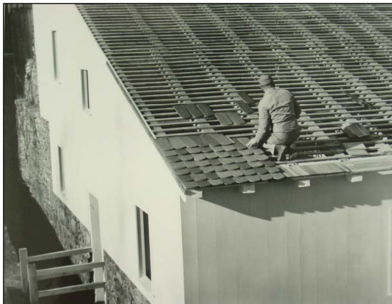
Figure 62. Installing tile shingles on the south slope of the cast house roof, November 17, 1964.
