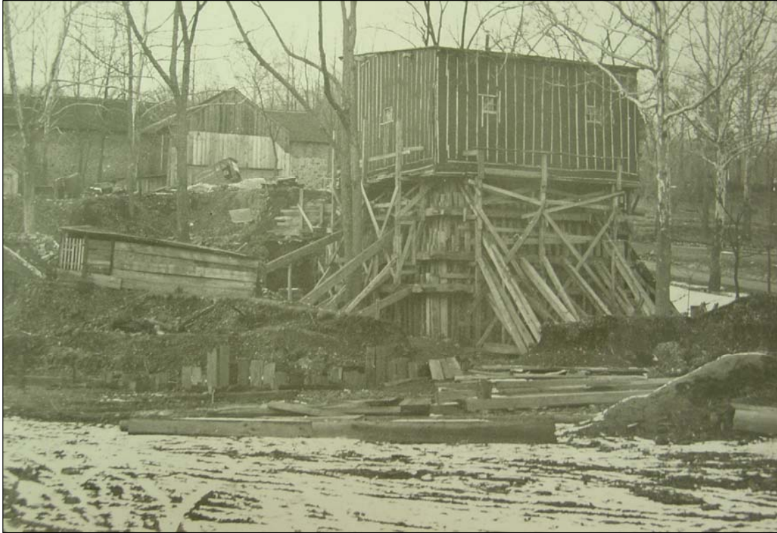
Figure 31. View looking northeast towards the charcoal house, showing temporary construction shed erected on top of the furnace stack, February 26, 1937.
