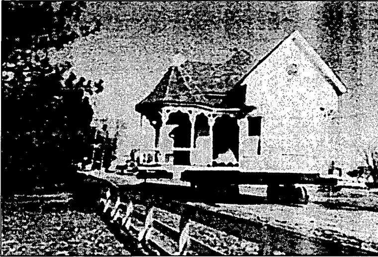
Figure 23. Relocation of 1903 C.E. Smith house (1969).
