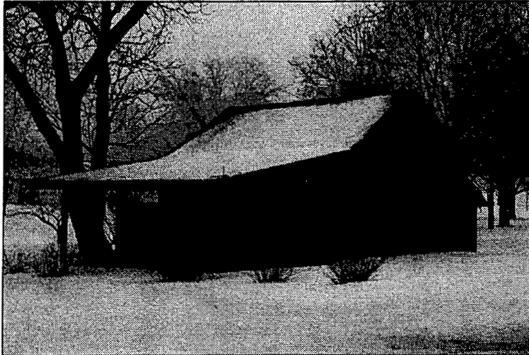
Figure 34. NPS maintenance structure in the historic core area.
