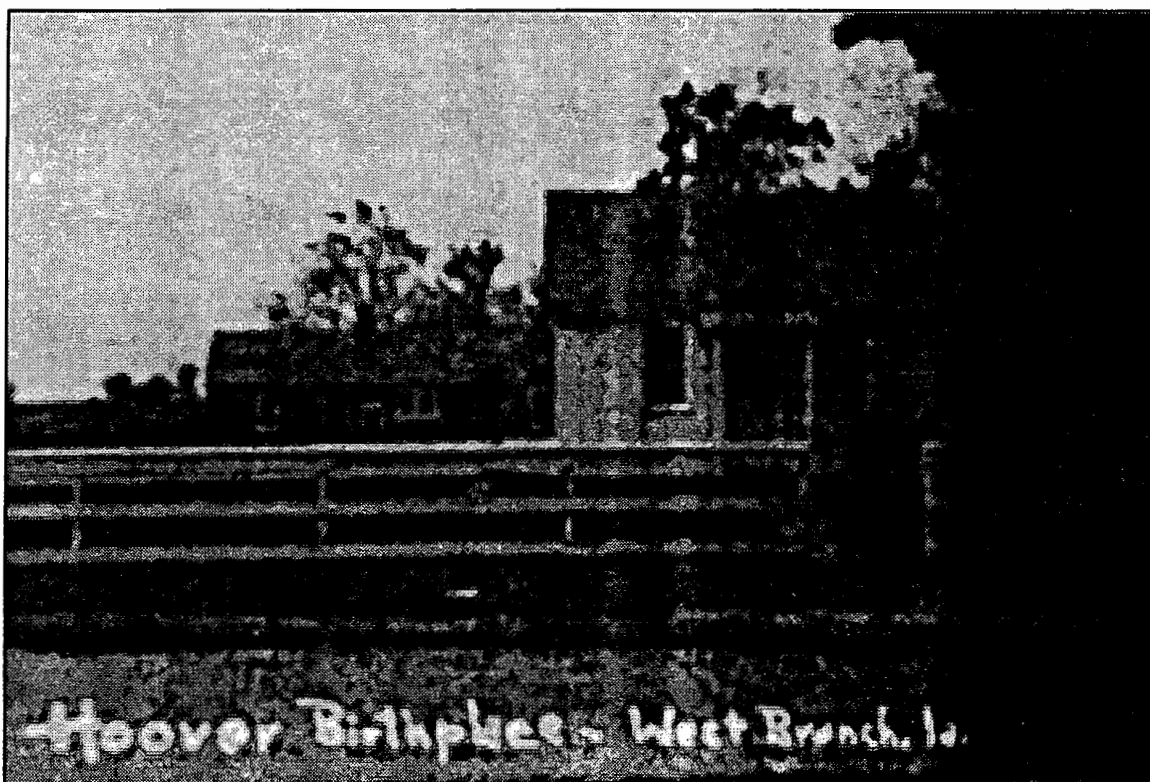
Figure 79. The birthplace cottage after restoration. The new caretaker's cottage visible in left background, 1938.
