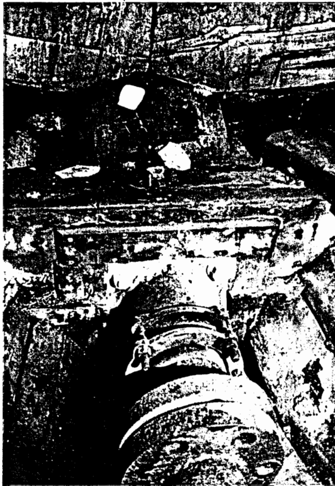
Fig. 23. Afterpeak, looking aft; stuffing box and shaft coupling. Pointer butt is seen over horn timber at top of photo. Note offset in coupling due to hull distortion. --TCM
