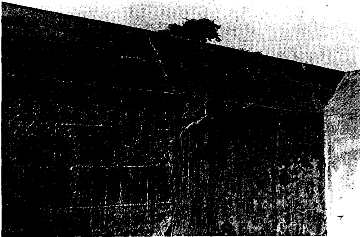
Plate 14. Concrete often retains evidence of how it was placed and finished. Different methods can still be seen today, and are expressions of building history. Battery Marcus Miller.
