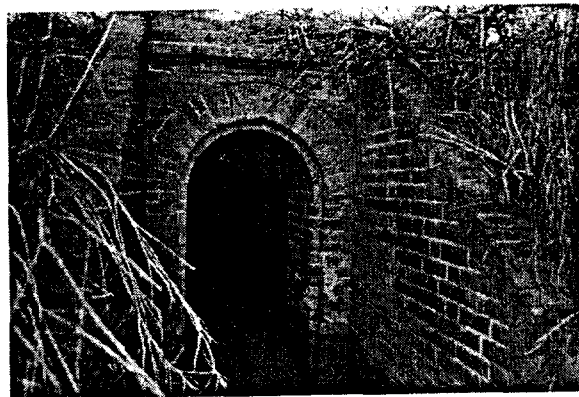
East Battery. Flooded magazine entry.
