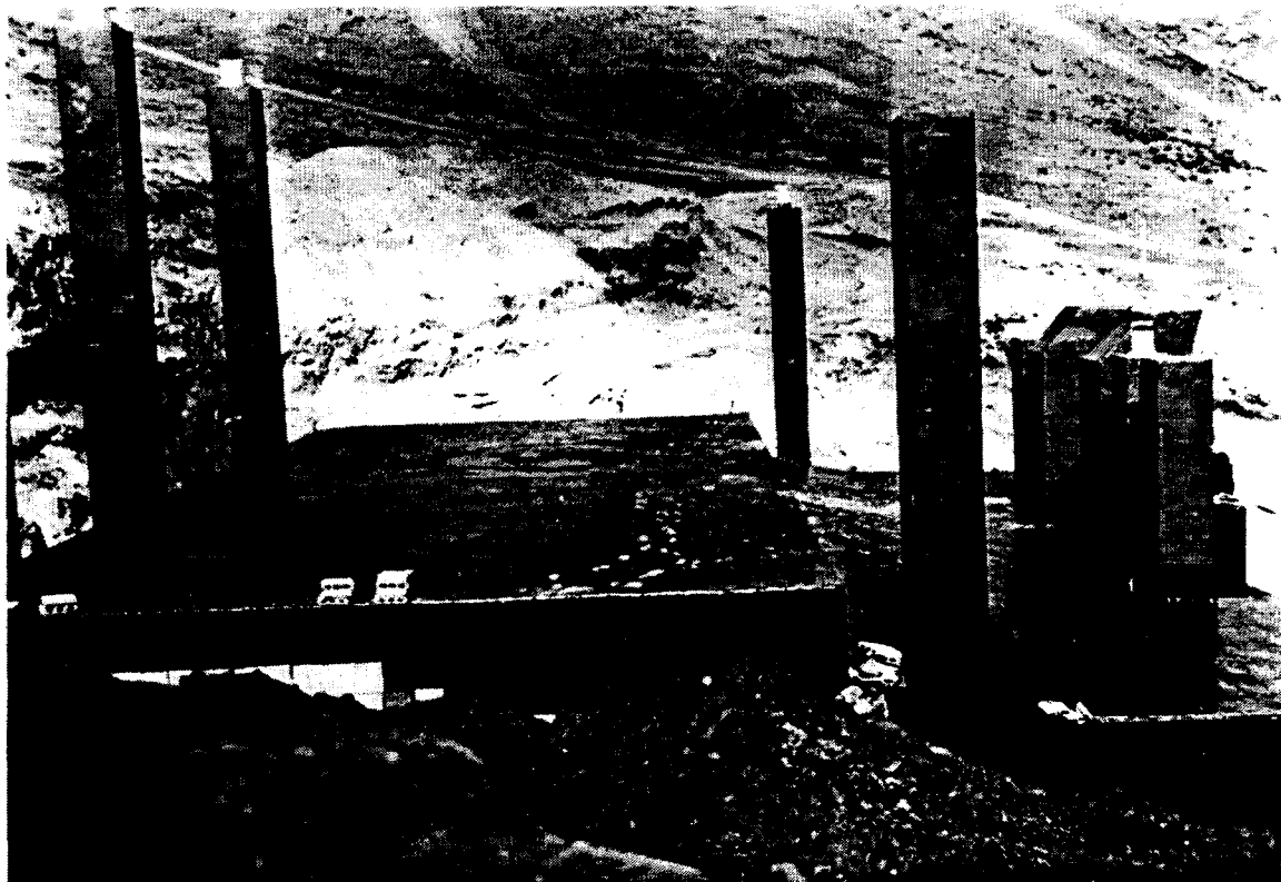
Plate 33. Battery Townsley, Fort Cronkhite, 1938-1940. Under construction, showing damp-proof membrane. Courtesy of the Park Archives of the Golden Gate National Recreation Area.
