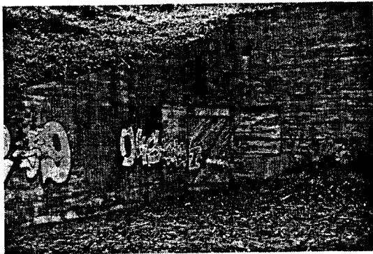
Battery Dynamite, emplacement three. Graffiti at rear corner, showing entry to cross-gallery. Also note debris accumulation and unique profile of sidewall.
