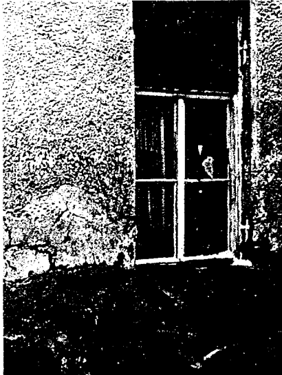
Rising damp in the underlying masonry caused this extensive surface coating damage.
