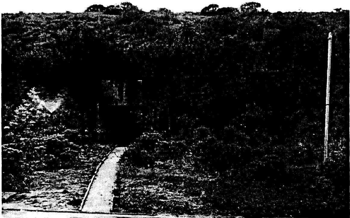
Plate 36. Battery Davis. Landscape camouflage at the power room entrance. View immediately post construction, September 1940. Courtesy of the Park Archives of the Golden Gate National Recreation Area.
