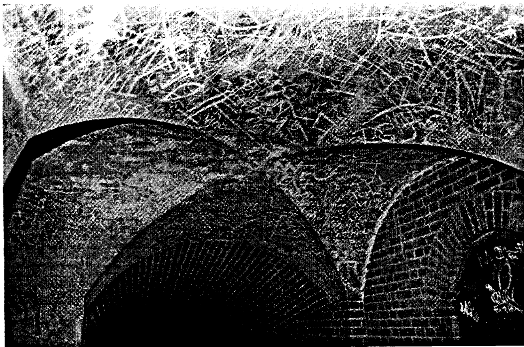
Plate 45. Although the batteries of the 1870s were built of earth and brick, concrete played an important role as well. Here a groin formed by the intersection of vaults in East Battery is made of concrete, displacing more expensive brickwork.
