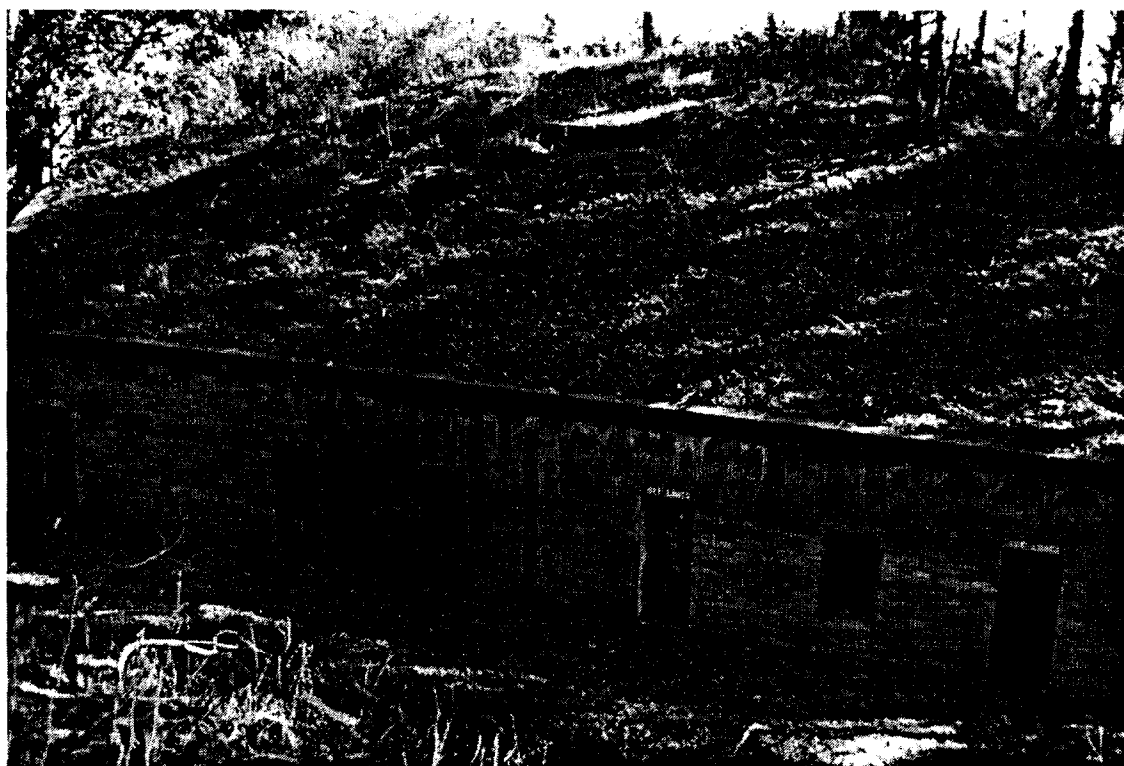
Plate 26. Battery Duncan. Rear of traverse showing fenestration, ladder to BC station, and BC station (overgrown at top of elevation).
