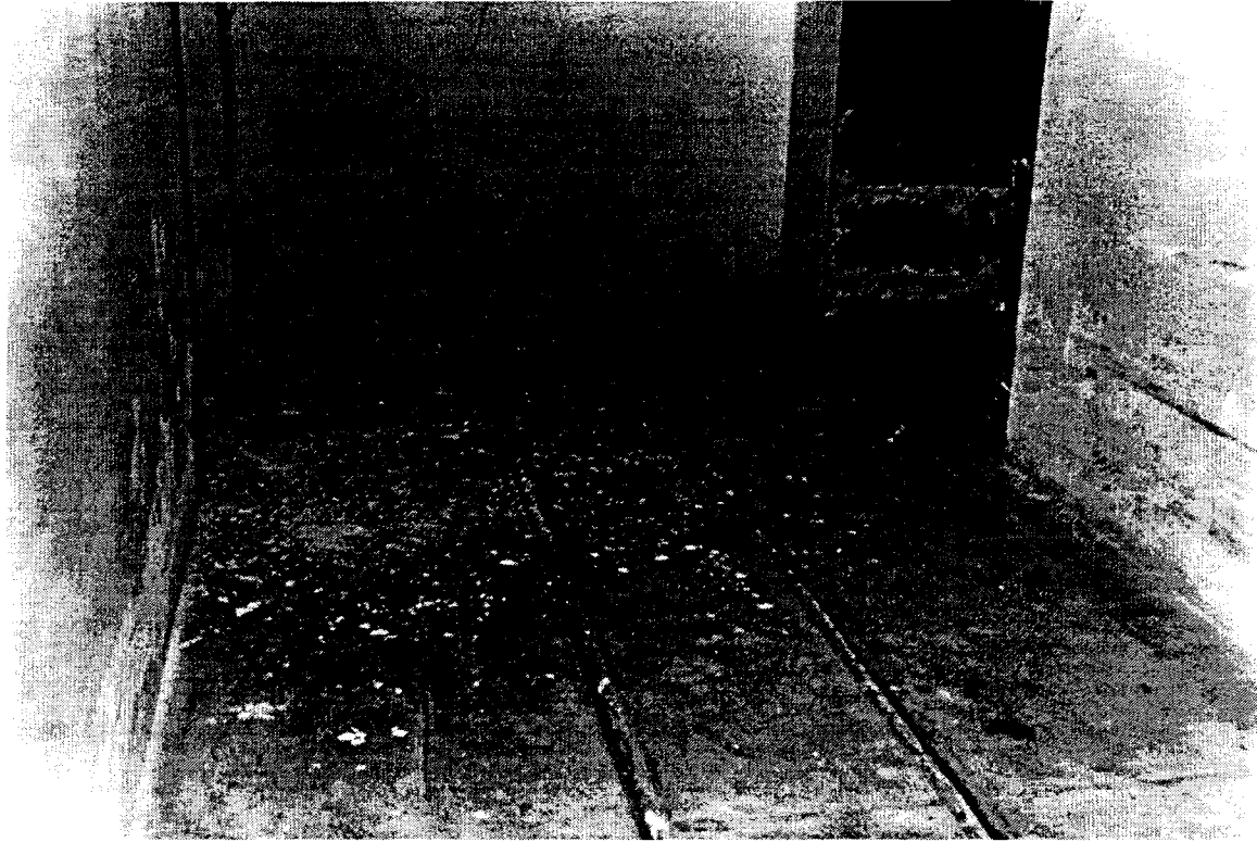
Plate 19. Tramways with turntables at intersections carried small rail cars that could be pushed by several men to carry ammunition into the interior of a battery. They were an uncommon feature of fortifications built in the United States. Battery Stotsenburg-McKinnon.
