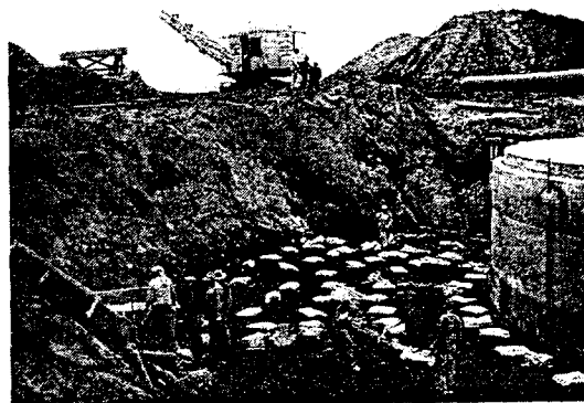
Battery Davis. Cement-soil stabilization, second operation, April 1938.
