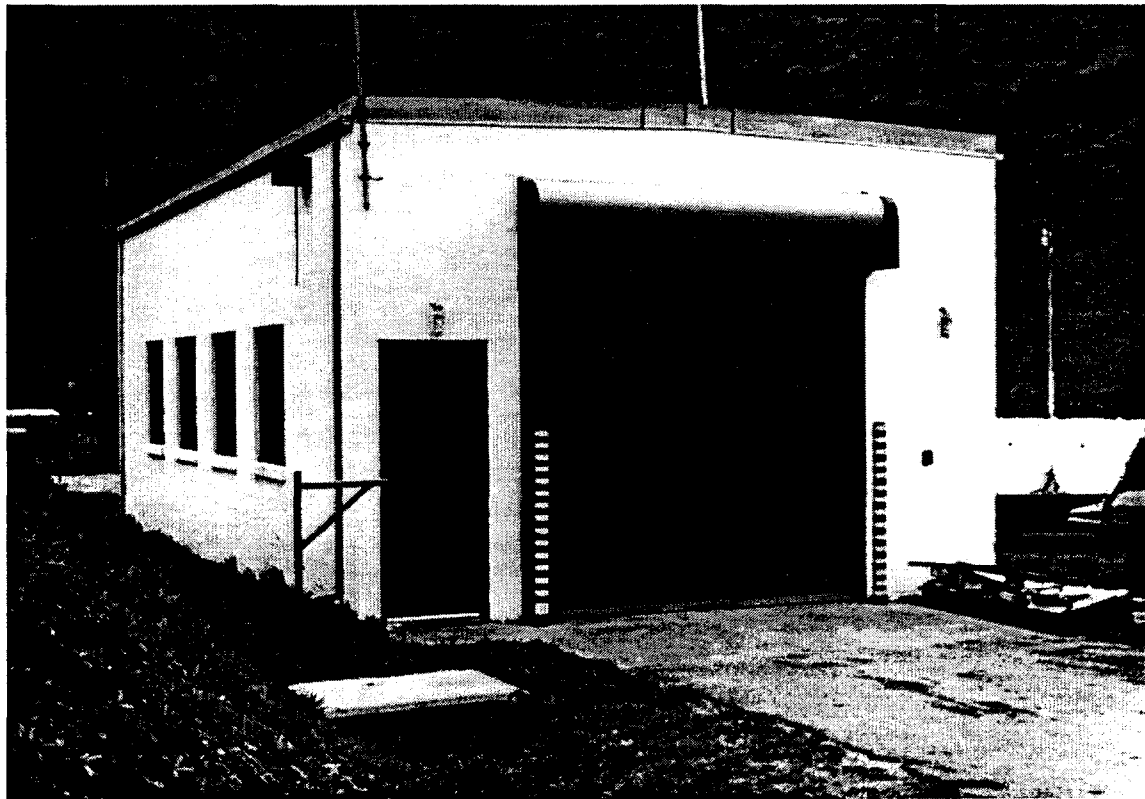
Plate 37. Nike Hercules Warhead Building, Nike Site SF-88L, Fort Barry, 1959. Courtesy of the Park Archives of the Golden Gate National Recreation Area.
