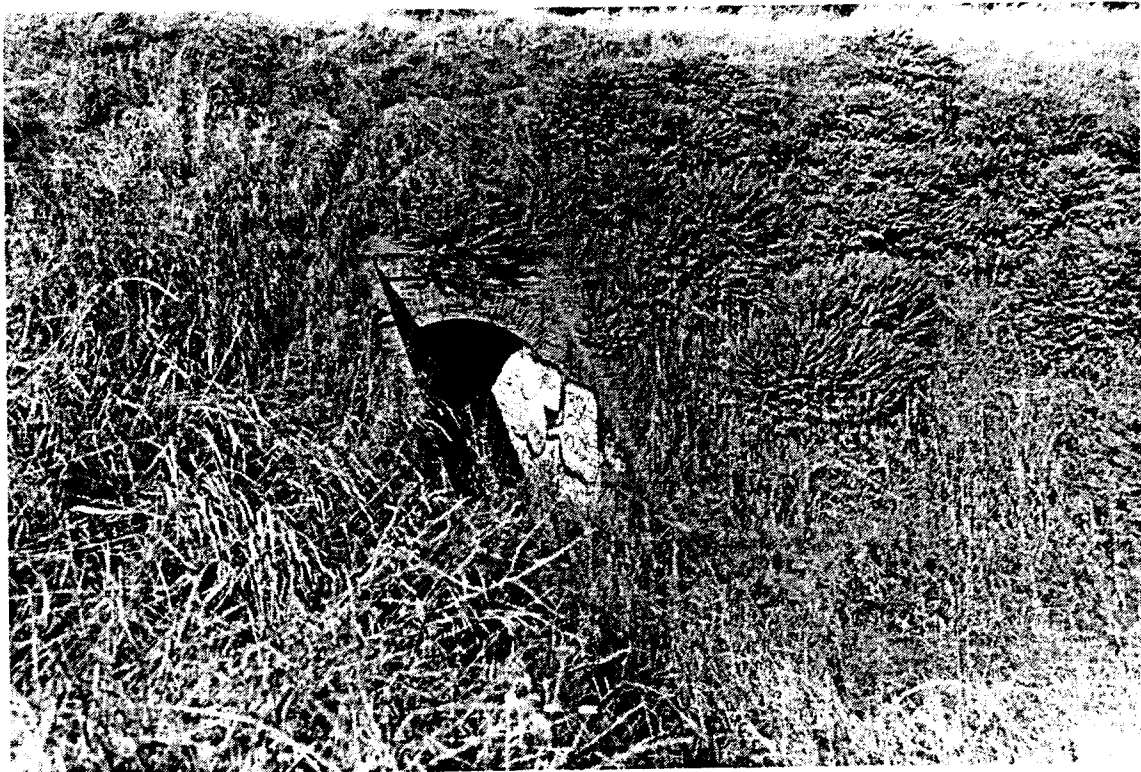
Plate 44. The design of Cavallo Battery called for the work to be accomplished in earth, and rendered in regular outlines. Those crisp outlines have been obscured by a century of plant growth.
