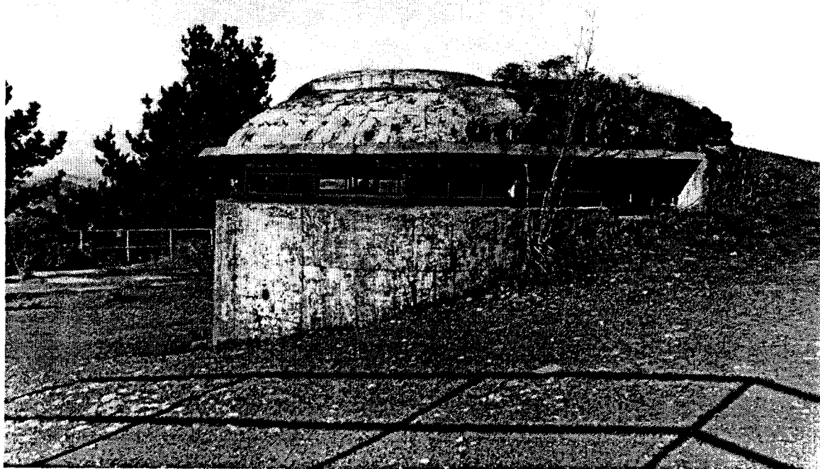
Plate 3. BC Station, Battery Construction #129, Fort Barry, constructed 1942-1944. Looking east.
