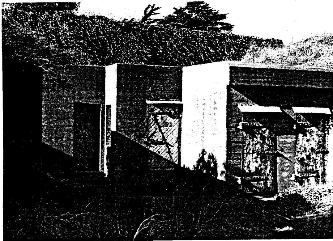
Plate 46. The designs for the earliest batteries did not anticipate the need for latrines, power plants, plotting rooms, and storage spaces. As a result, later building tacked on these components to fortifications completed only a few years before. These additions at Battery Godfrey are an example of the practice; they also portray the preference for steel doors in later construction.
