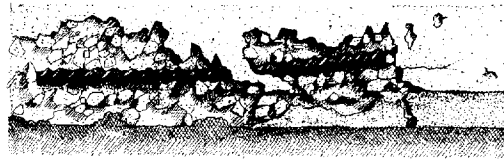
Battery Marcus Miller. Detail view of spalling concrete. Spalling can be caused by expansive corrosion acting on reinforcing steel.
