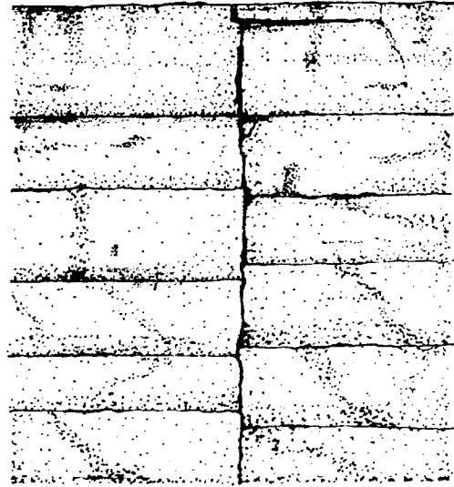
Typical concrete cold joint showing minor spalling, surface deterioration and original form marks. This cold joint is at Battery Marcus Miller.
