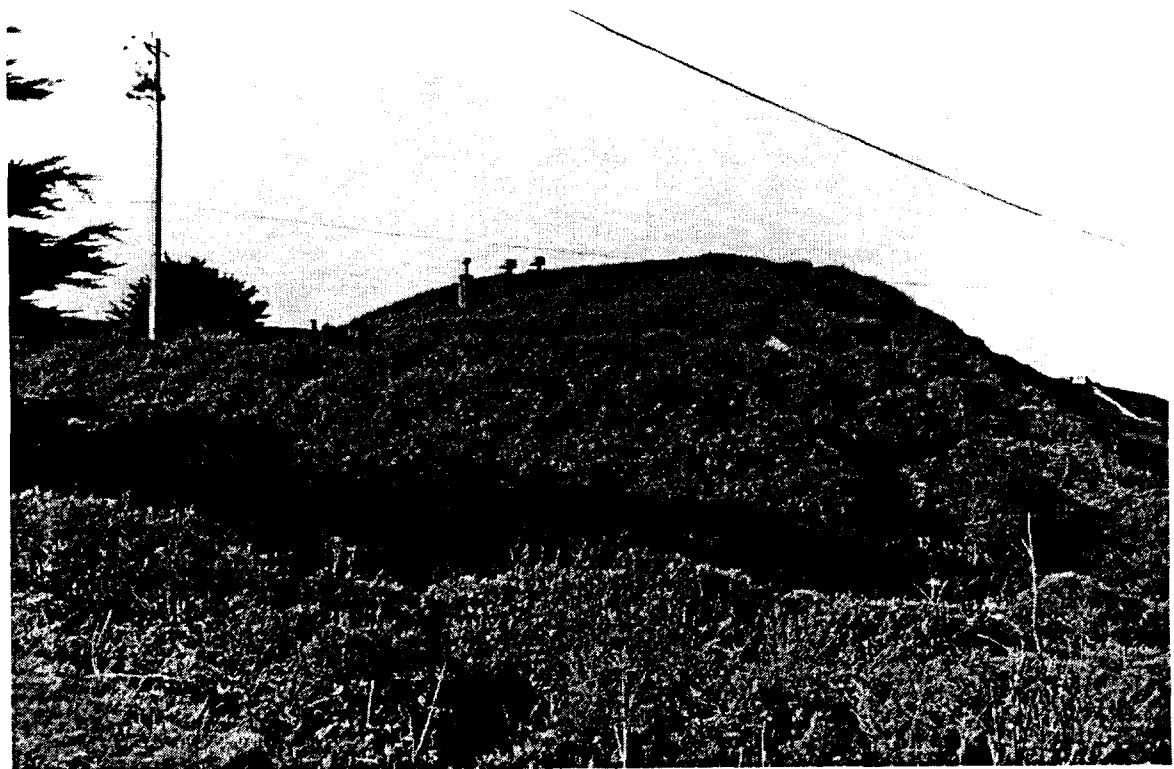
Plate 13. Earth remained a constant in the fortifications built after the Civil War. Here at the Fort Barry mine casemate, it covered a modern structure of reinforced concrete, rendering that structure invisible to eyes that might view it from the sea or the air.
