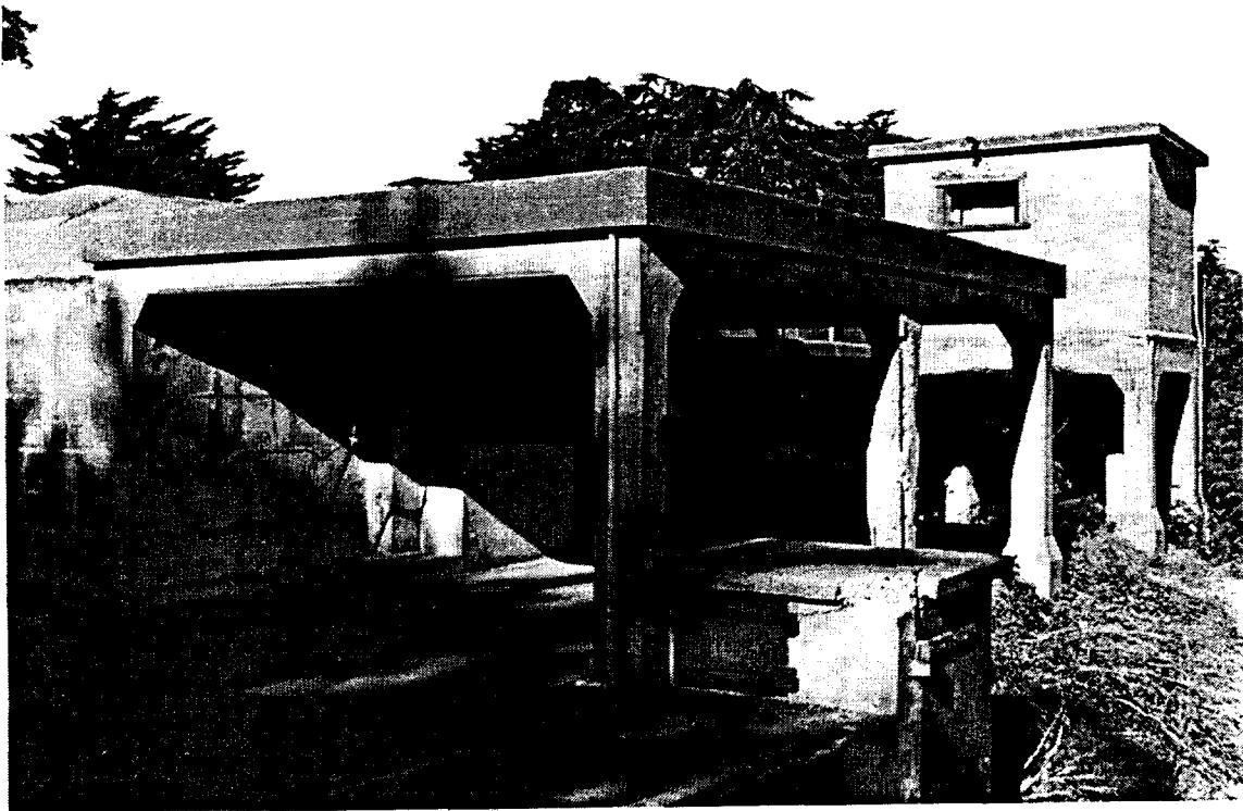
Plate 43. Even after the structures of the Endicott and Taft periods were completed, there was a pattern of improvements that also incorporated advances in concrete construction. The telautograph booth, ammunition hoist and splinterproof, and battery commander's station, shown here, were built between 1904 and 1912. These additions at Battery Marcus Miller were among the first attempts to use reinforced concrete in the fortifications.
