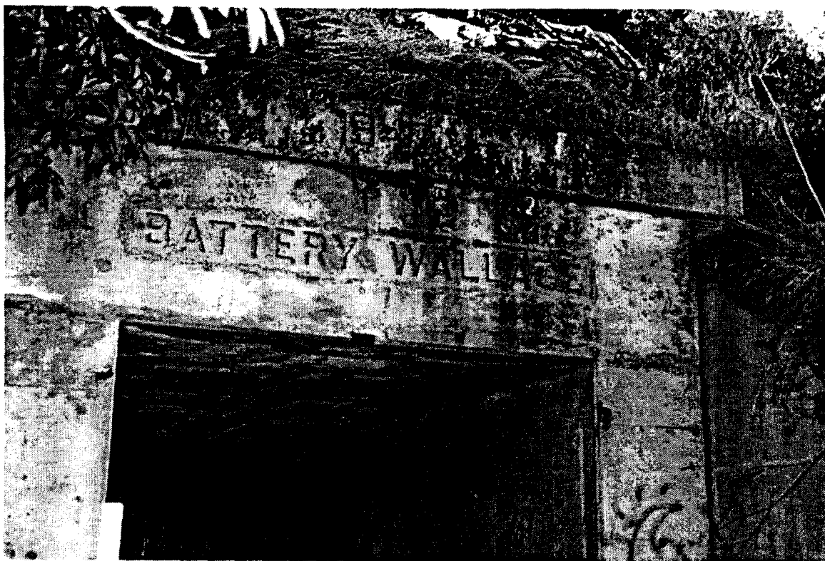
Plate 4. Battery Wallace, Fort Barry, constructed 1917-1921. With casemating of its two guns in 1942-1943. Emplacement entry.
