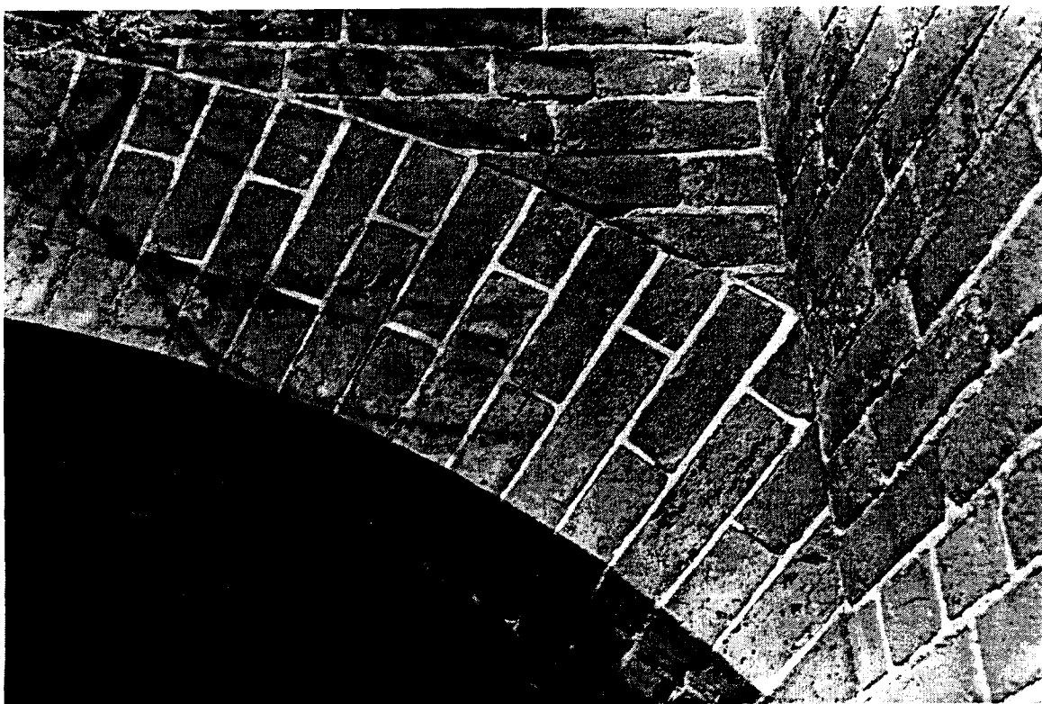
Plate 11. The quality of brickwork in the surviving elements of the 1870s is very high, reflecting both the careful selection of materials as well as the skill of the masons. Cavallo Battery.
