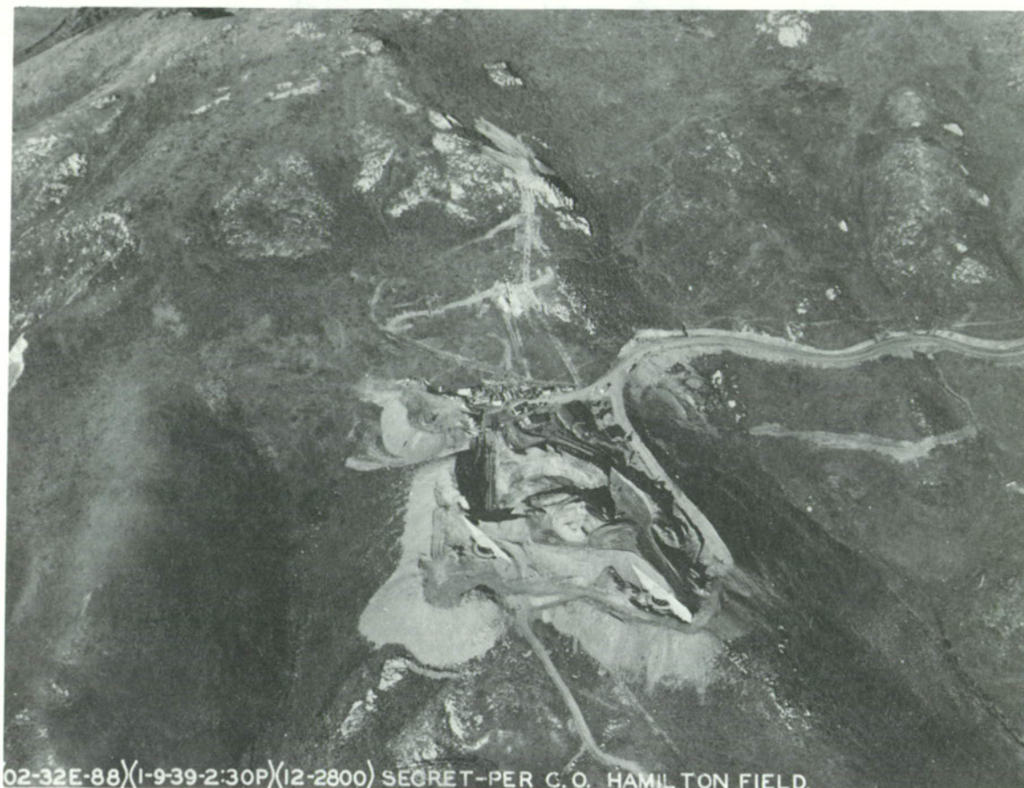
17. Battery Townsley nearing completion, Fort Cronkhite, 1939.
