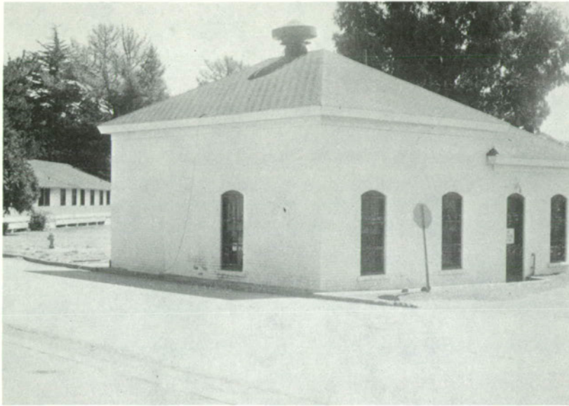
7. Pumphouse, Fort Baker, 1977.
