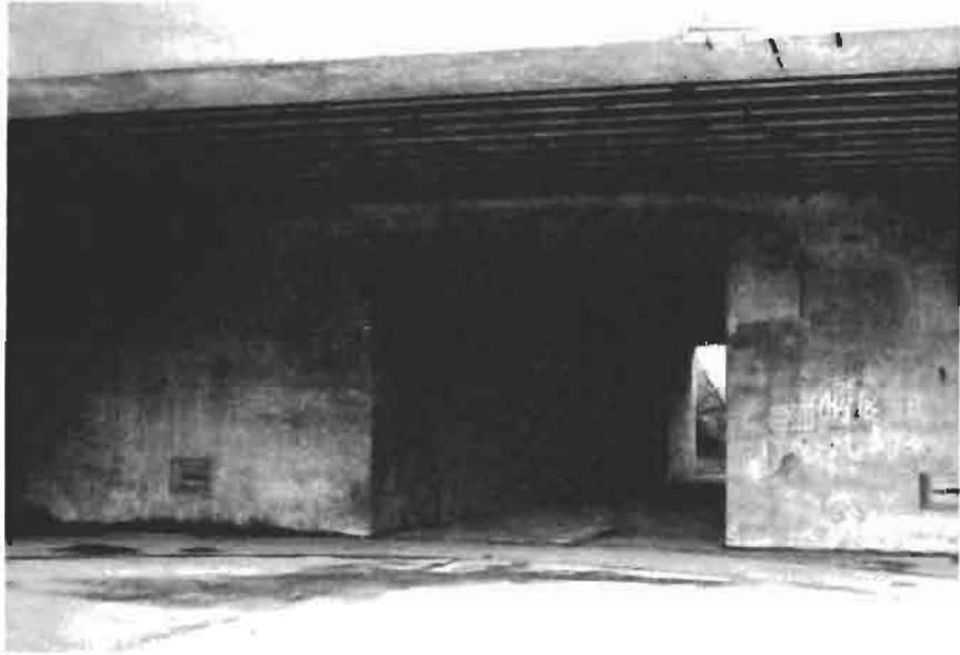
South view of Structure 410 Battery Harris 1979
