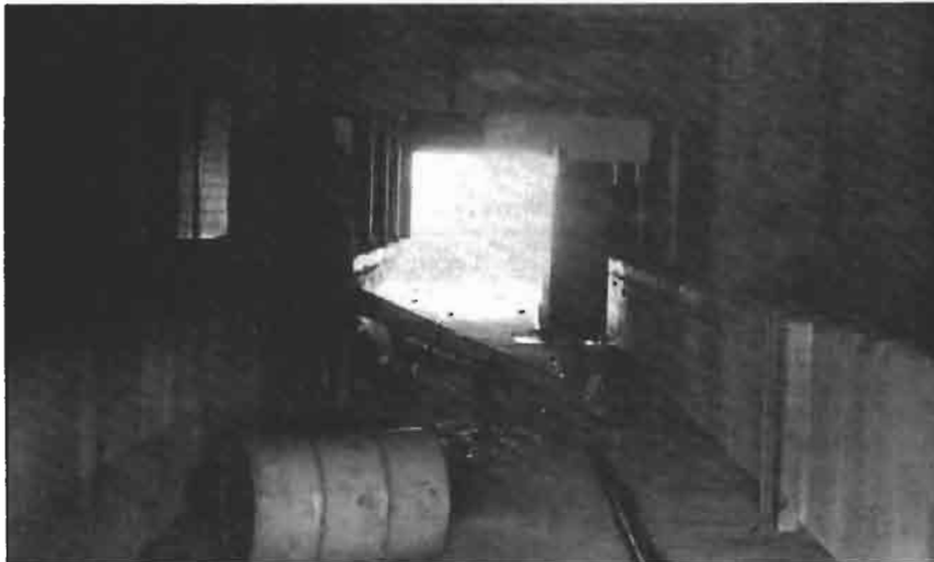
Illustration 20 Interior view of magazine Building 405 Battery Harris 1979
