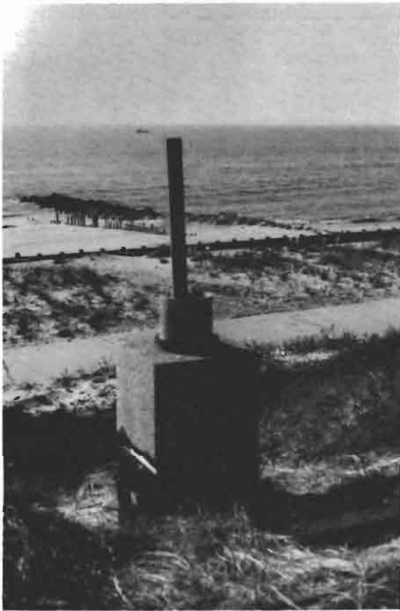
Illustration 15 Exhaust vent of Structure 321 Battery Kessler 1979
