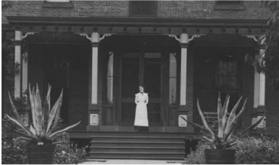
Figure 36. Officers Club, east- facade piazza, showing period paint scheme, ca. 1900.
