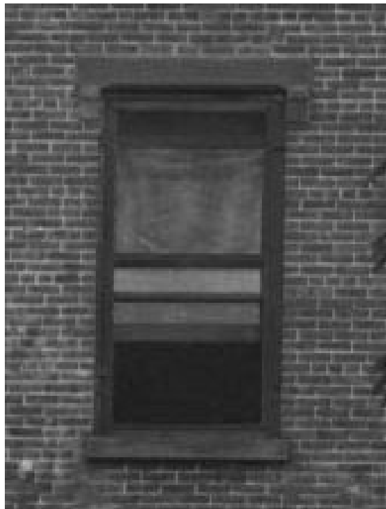
Figure 25. Officers Club, east façade, second story, showing typical window elements, ca. 1900.
