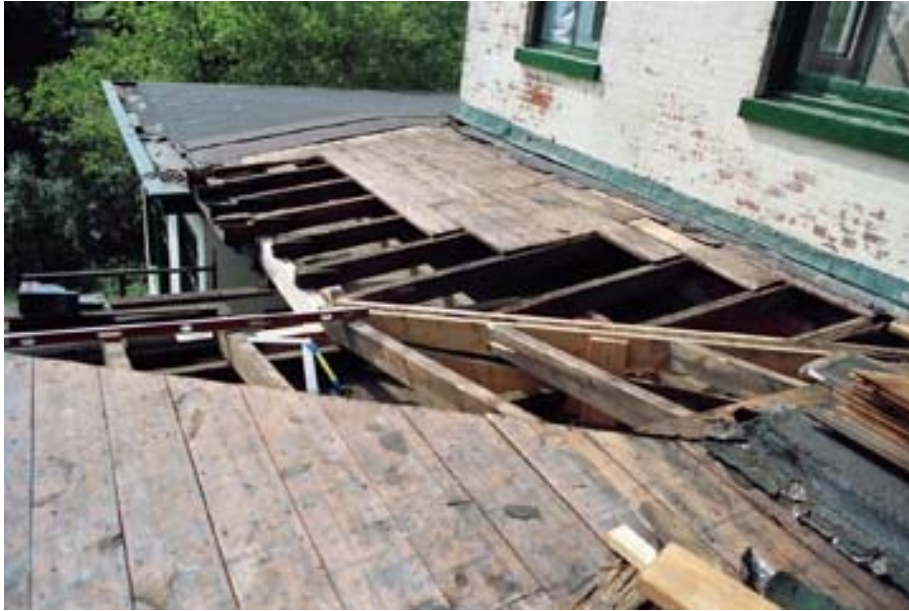
Figure 34. Officers Club, east façade, piazza roof, showing original framing and repairs, 1991.
