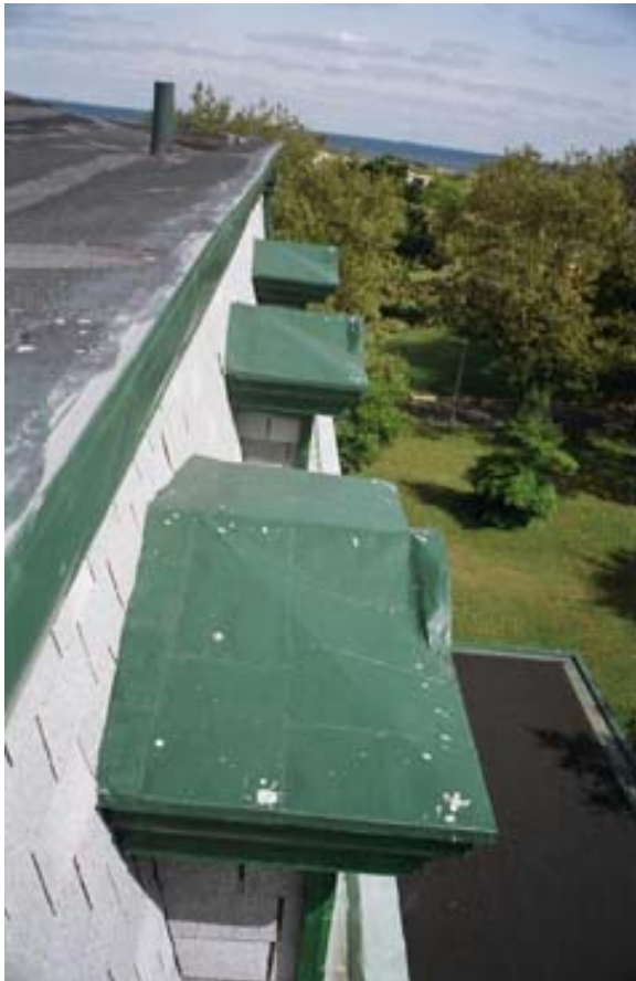
Figure 33. Officers Club, mansard roof, dormer roofing material, 1992.
