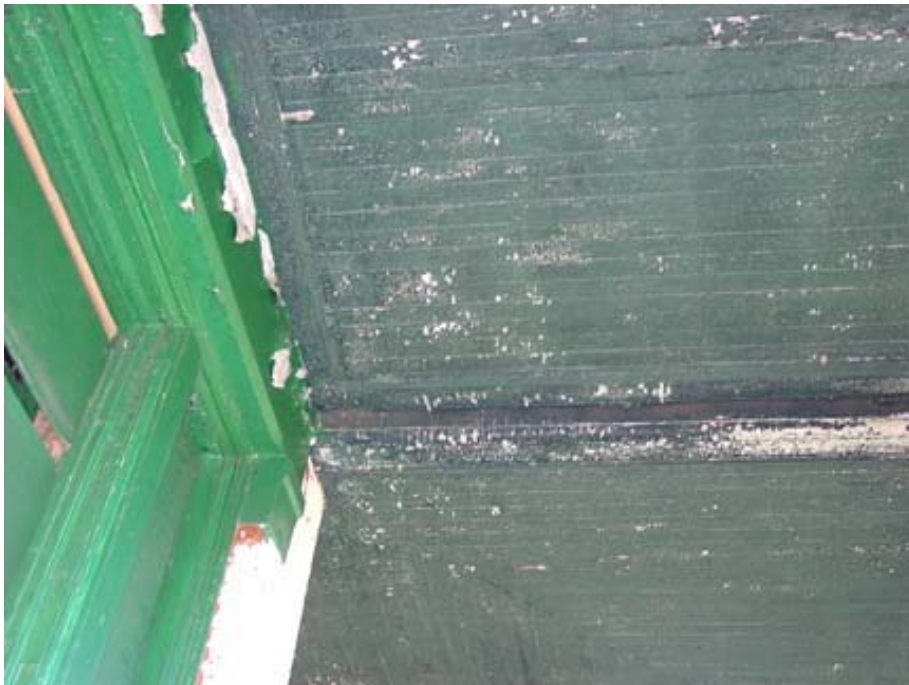
Figure 23. Officers Club, east façade , piazza ceiling, 2005.
