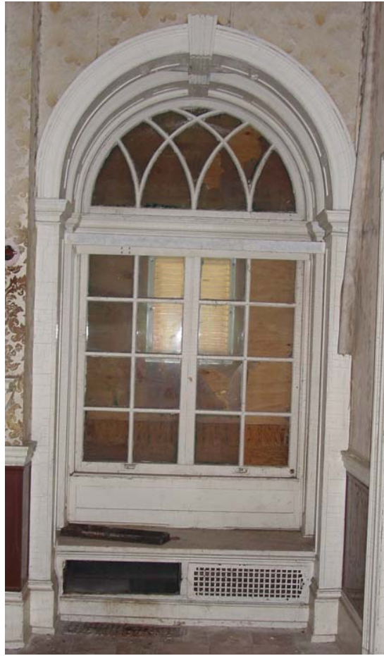
Figure 51. Officers Club, west- elevation window W124, seen from the Dining Room (Room 106), 2005.
