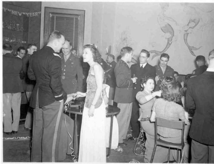
Figure 76. Officers Club, Men's Lounge (Room 104), showing trompe l'oeil painting on east wall, 1942.
