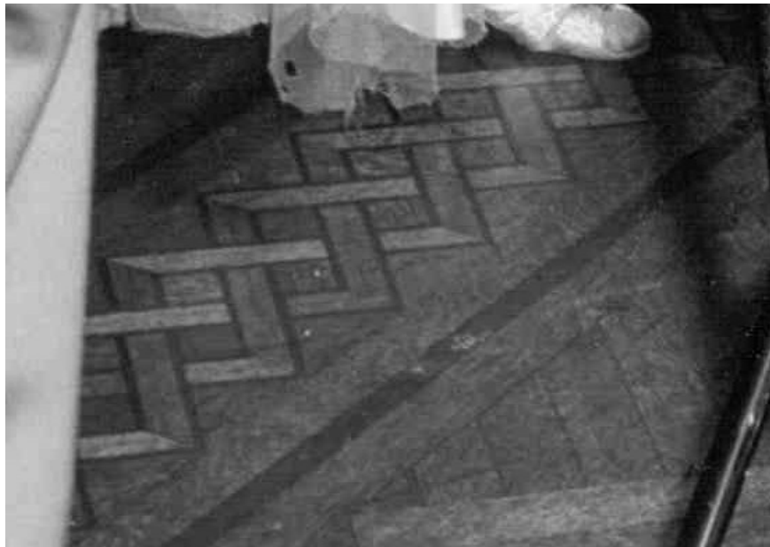
Figure 42. Officers Club, Men's Lounge (Room 104), detail from historic photograph showing parquetry floor no longer extant, ca. 1942.
