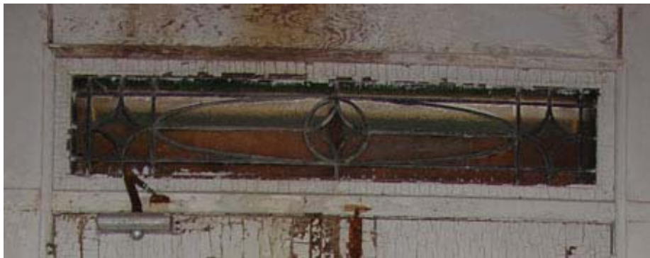
Figure 61. Officers Club, transom above east- façade main entrance, as seen from center hallway (Room 102), 2005.
