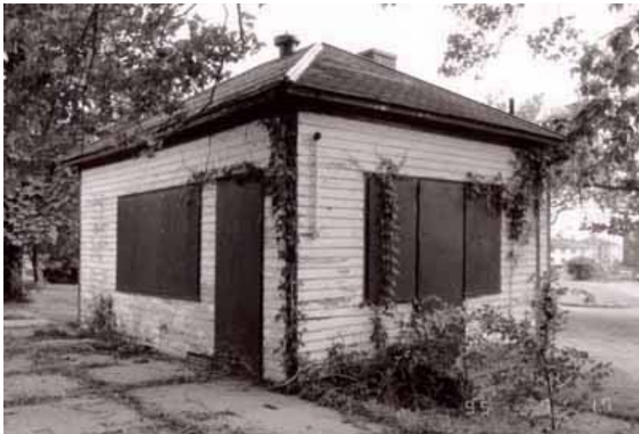
Figure 81. Laundry/Caddy House, Building No. 113, 1995.
