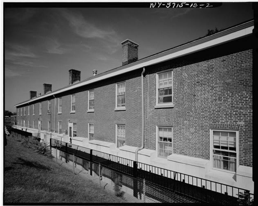
Figure 105. Rear elevation of the south barrack (Building 206), 1982- 83.
