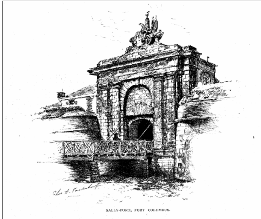
Figure 41. The “sally port,” or main entrance, of Fort Columbus, 1881.
