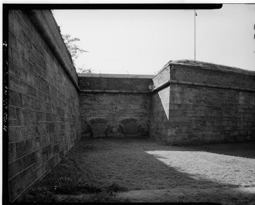
Figure 84. Ditch and northeast scarp of Fort Jay, 1982- 83.
