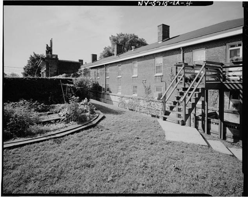
Figure 103. East elevation of the east barrack (Building 202) north of the sally port, 1982- 83.
