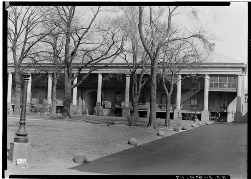
Figure 64. West elevation of the east barrack (Building 202) of Fort Jay, March 1934.
