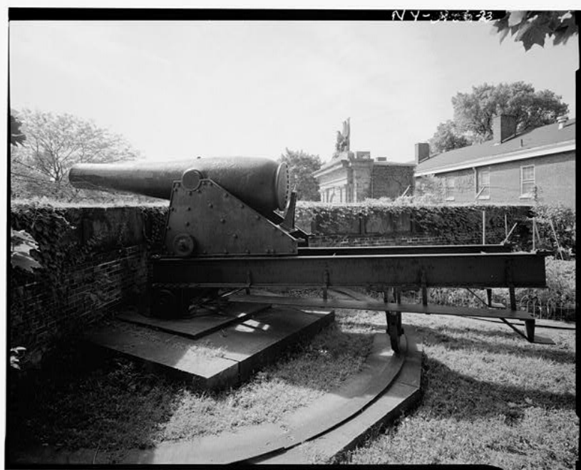
Figure 88. Gun emplacement on the northeast bastion of Fort Jay, 1982- 83.
