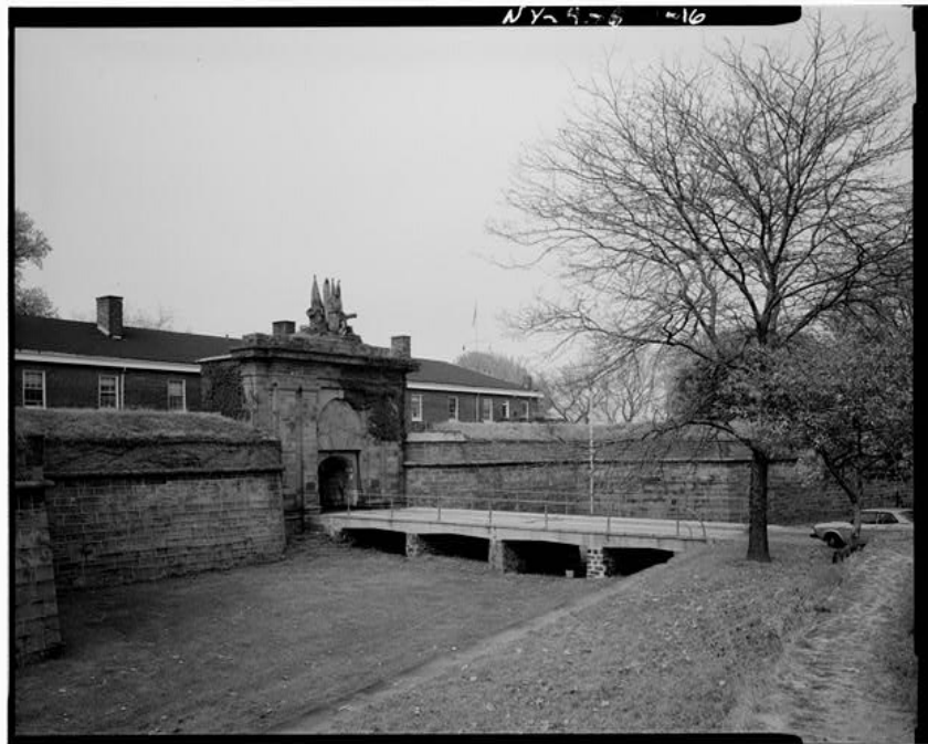
Figure 85. East entrance (sally port) of Fort Jay looking northeast, 1982- 83.
