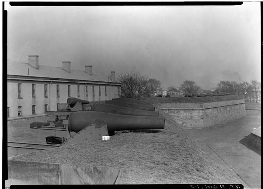
Figure 60. View from the southwest bastion of Fort Jay showing the back side of the south barrack (Building 206), March 1934.
