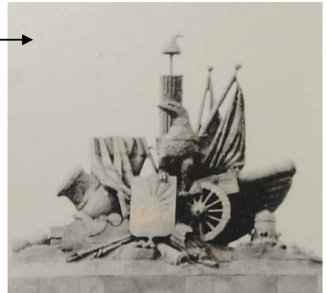
Detail view of the gateway sculpture. Note missing eagle wings and upper portion of the left flag.
