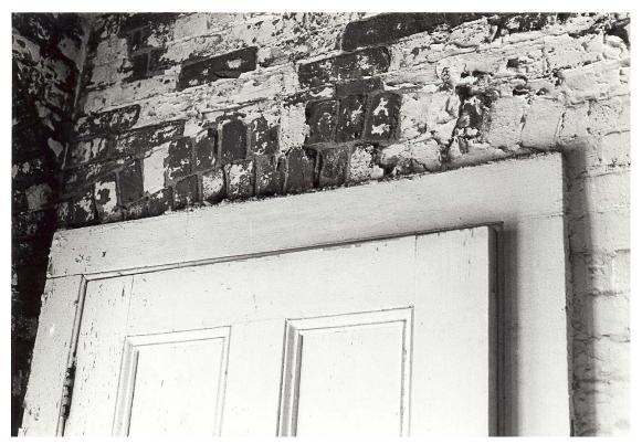
Figure 97. Tower interior: brick arch over doorway in sixth-landing room (1983).
