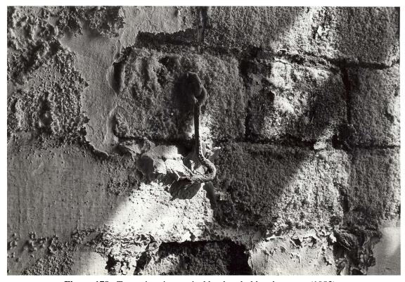
Figure 179. Tower interior: typical hook to hold sashes open (1983).
