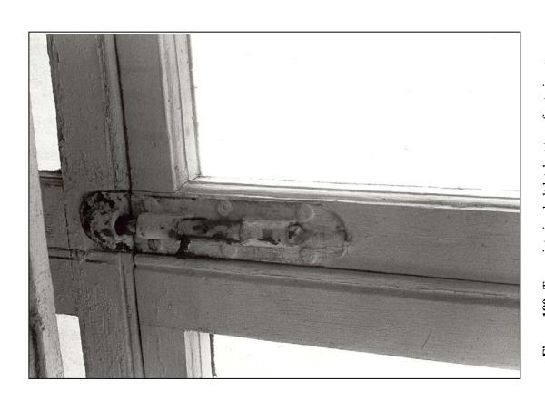
**Figure 180.** Tower interior: bolt latch at top of exterior storm sashes (1983).
