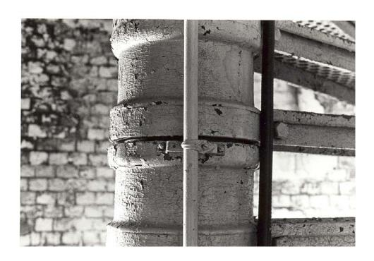
Figure 146. Tower interior: central column, seam separation (1983).
