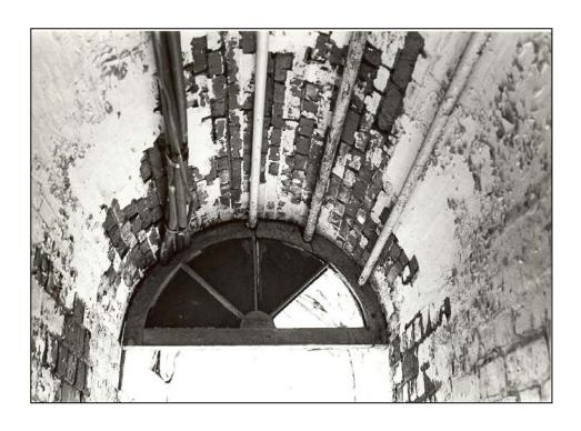
**Figure 151.** Tower interior: conduits entering through entrance-doorway fanlight (1983).
