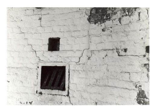
Figure 106. Tower interior: Watch Room, cracks in wall brickwork (1983).
