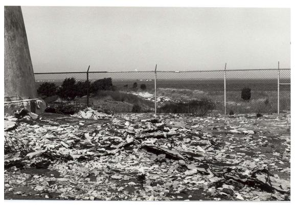
Figure 89. Tower exterior: protective coating debris at base of tower (1983).
