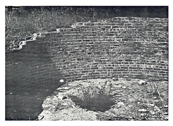
Figure 5. First Fire Island lighthouse: brick interior wall.
