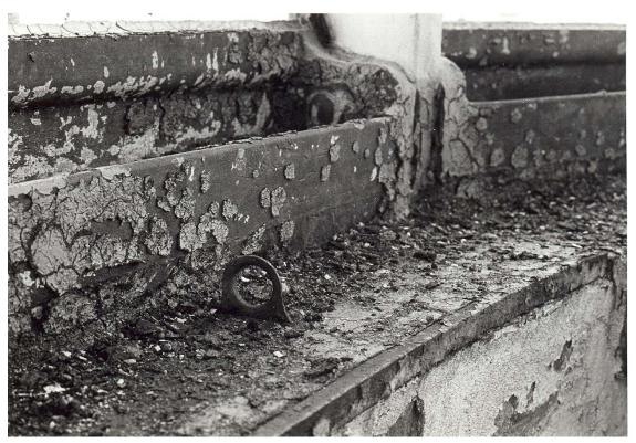
Figure 127. Tower interior: opening in lantern floor, traces of former trapdoor (1982).
