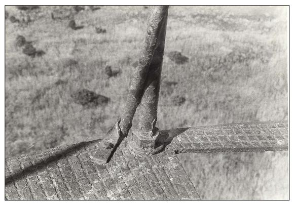
Figure 198. Tower exterior: diagonal brace tied to deck of upper balcony (1983).
