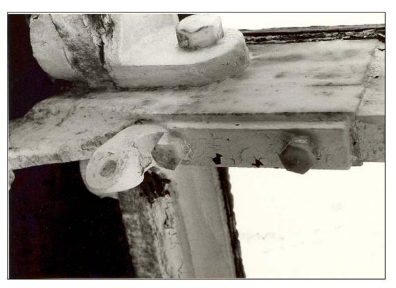
Figure 207. Tower interior: detail of bracket for lantern curtain (1983).
