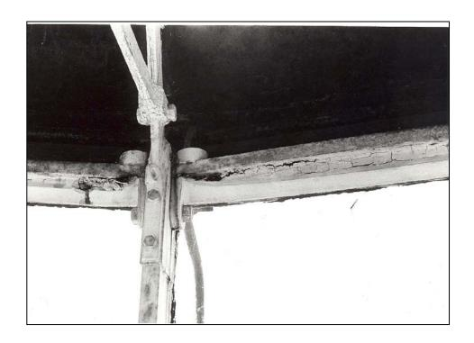
Figure 193. Tower interior: lantern cornice area, deterioration of fittings (1983).
