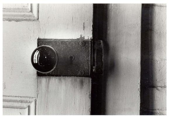
Figure 165. Tower interior: sixth-landing room, rim lock of door to main stairway (1983).
