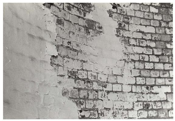
Figure 103. Tower interior: deterioration of wall whitewash (1982).
