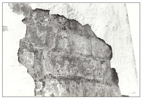
Figure 104. Tower interior: deterioration of wall whitewash (1982).
