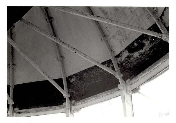
**Figure 189.** Tower interior: lantern roof, junction of spider frame and lower frame (1982).
