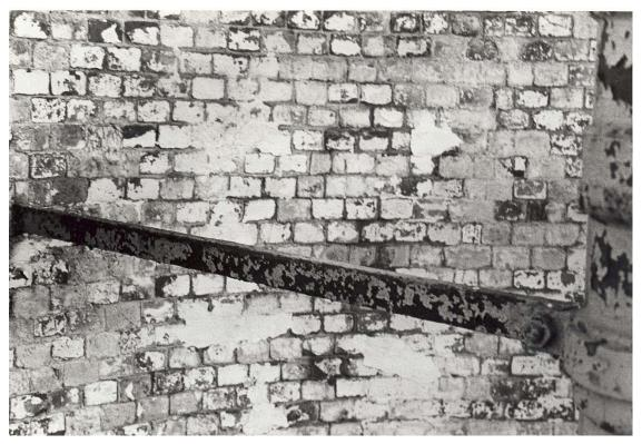
Figure 133. Tower interior: main stairway, girder of landing (1983).
