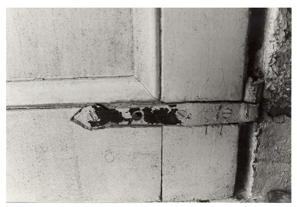
Figure 161. Tower interior: entrance door, strap hinge and pintle (1983).
