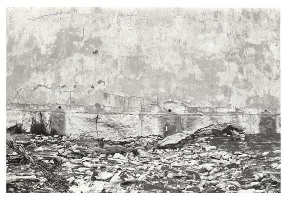
**Figure 80.** Tower exterior: plinth with ventilation holes (1983).
