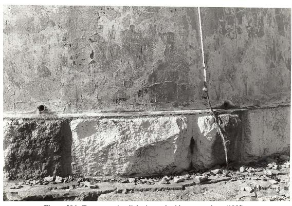
**Figure 206.** Tower exterior: lightning-rod cable at tower base (1983).
