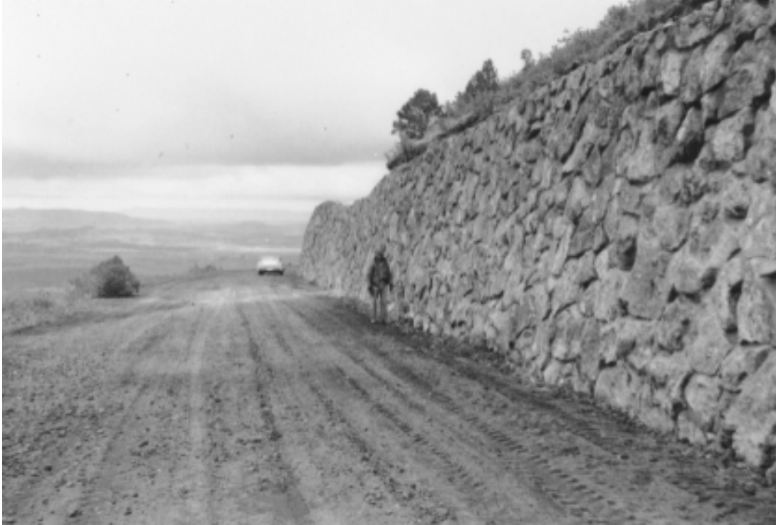
Fig. 7.16 Completed Retaining Wall, Circ. 1961, Photographer unknown, Completion Report, (Capulin: Capulin Volcano National Monument Administrative Records, Completion Reports), File D2621.
