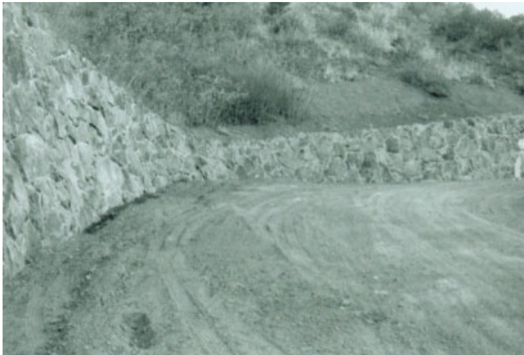
Fig. 7.22 Completed Retaining Wall, Circ. 1961, Photographer unknown, Completion Report, (Capulin: Capulin Volcano National Monument Administrative Records, Completion Reports), File D2621.
