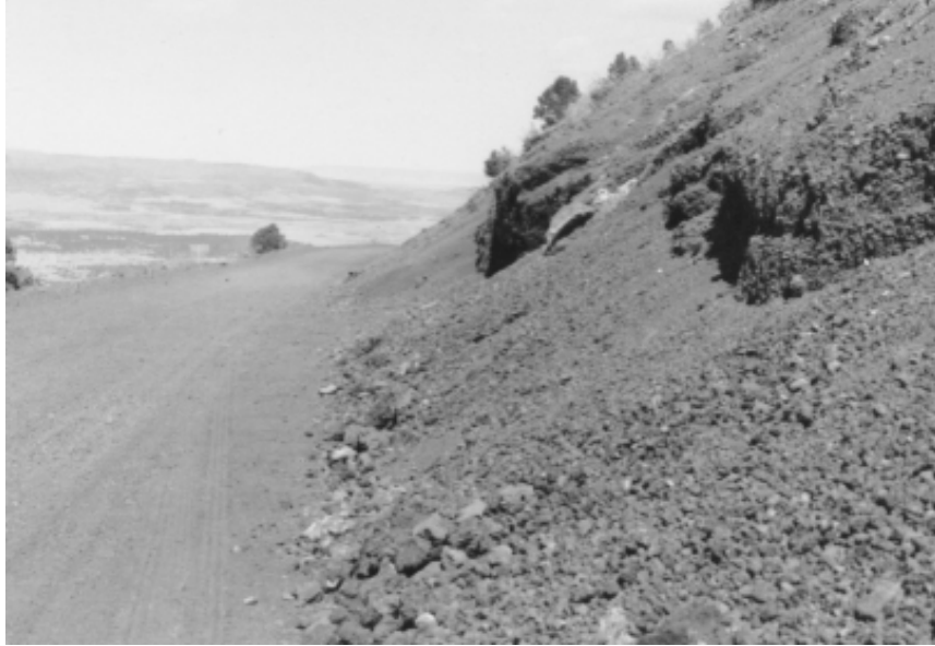
Fig. 7.12 Crater Ascent Road Before Retaining Wall Construction, Circ. 1960, Photographer unknown, Completion Report, (Capulin: Capulin Volcano National Monument Administrative Records, Completion Reports), File D2621.
