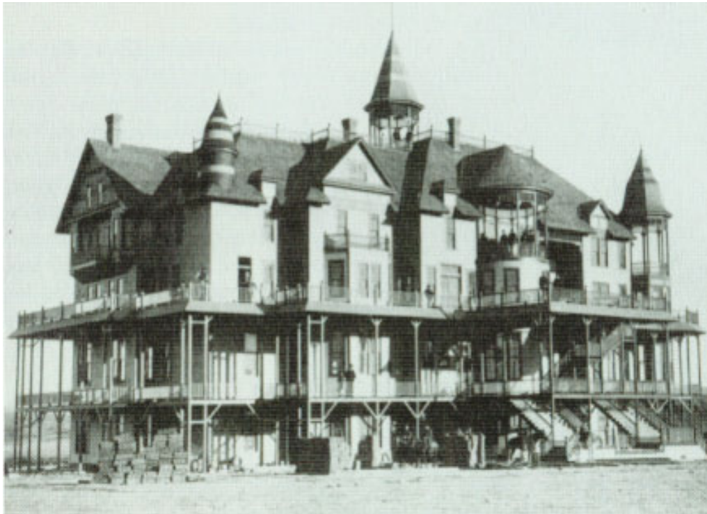
Fig. 3.3 The Big Hotel or Capulin Hotel Photograph courtesy of Mary Owen-Doherty and Emma Hardesty-Adams, The Folsom, New Mexico Story and a Pictorial Review (Folsom: No Publisher Listed, June, 1976), 15.
