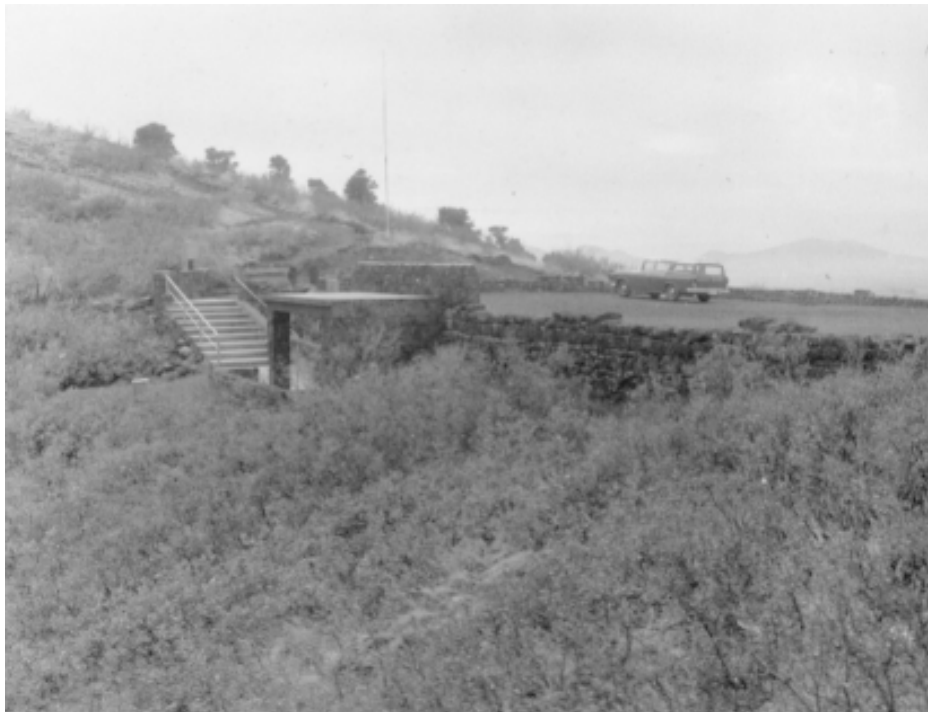
Figs. 7.5 Exhibit Shelter and Stairs looking towards the rim parking, Circ. 1955. Photographer unknown. Capulin: Capulin Volcano National Monument Administrative Records, Completion Reports, File D2621.
