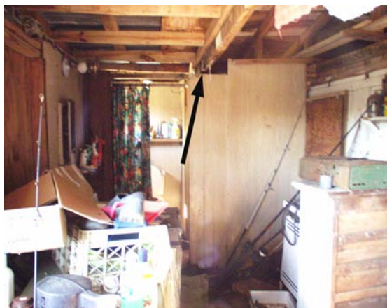
Figure 42 View northwest in Room 105. Arrow marks header at outside of historic porch. (NPS-SERO-CR, 2002)
