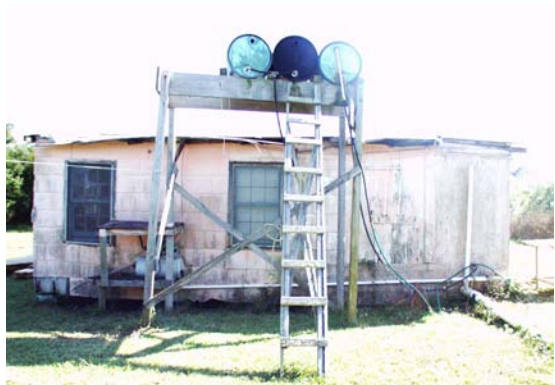
Figure 22 View of water tanks at rear of house. (NPS-SERO-CR, 2002)
