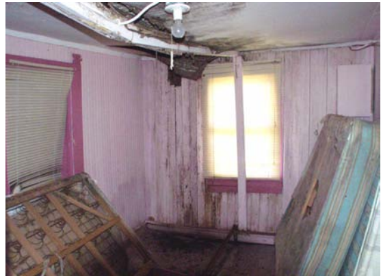
Figure 40 View to west in Room 104. (NPS-SERO-CR, 2002)
