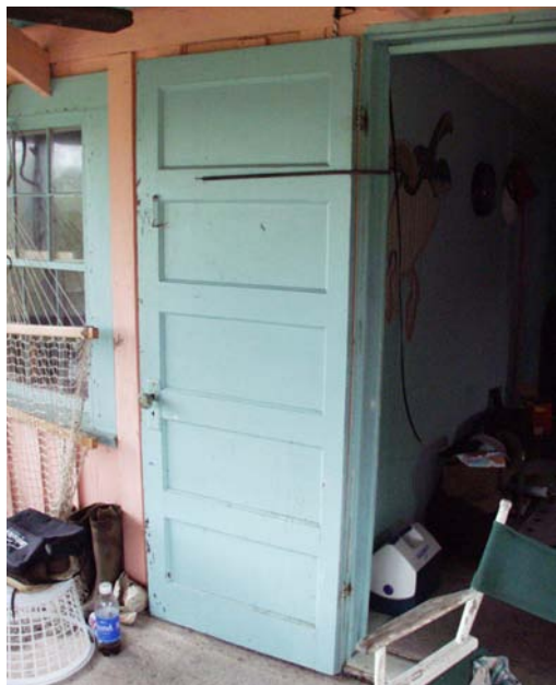
Figure 30 View of front door D-1. (NPS-SERO-CR, 2002)
