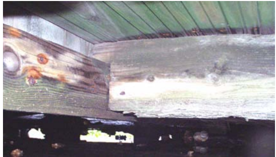
Figure 24 View of typical joist sill connection. (NPS-SERO-CR, 2002)
