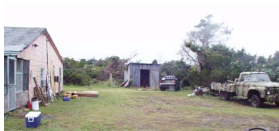
Figure 21 View to northwest, showing metal storage building in rear yard. (NPS-SERO-CR, 2002)
