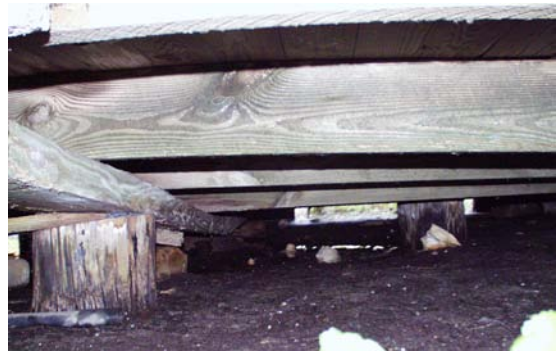
Figure 23 View of crawl space and piers. (NPS-SERO-CR, 2002)
