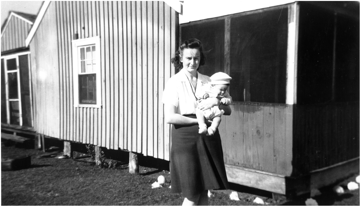
Figure 16 View of Lewis-Davis House in 1942. (CALO Coll., Royer photographs)
