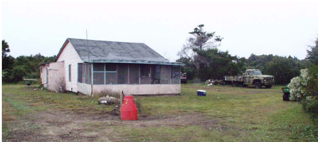
Figure 20 View to north of Carrie Davis House. (NPS-SERO-CR, 2002)
