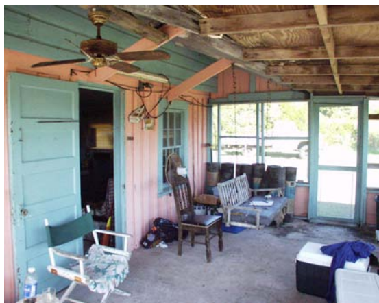
Figure 31 View to north on front porch. (NPS-SERO-CR, 2002)
