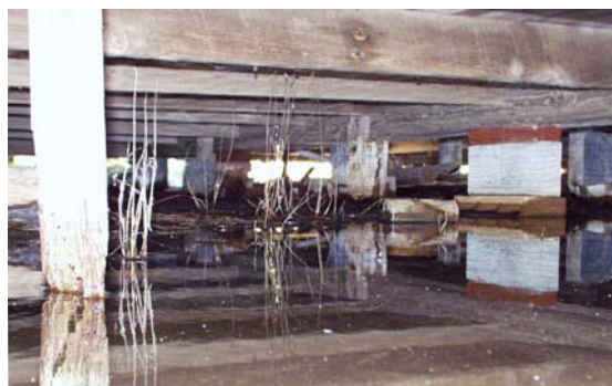
Figure 16 View to south from rear of house, showing standing water several days after rain. (NPS-SERO-CR, 2003)
