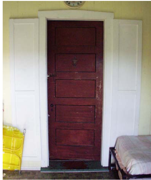
Figure 22 View of front door. Shutters and possibly the shaped header are modern additions. (NPS-SERO-CR, 2003)
