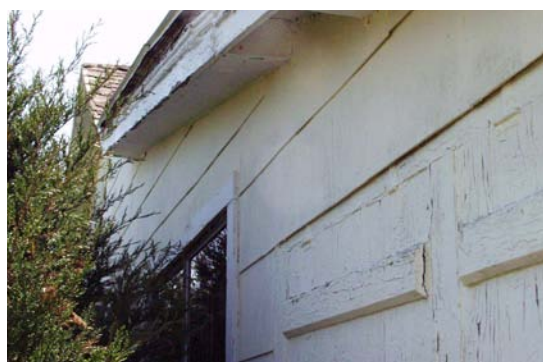
Figure 26 View of typical exterior finishes including top-hinged shutters from original back porch. (NPS-SERO-CR, 2003)
