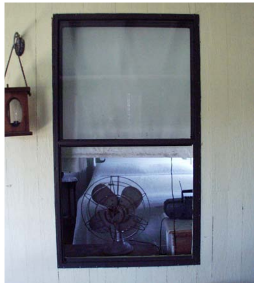
Figure 23 View of typical modern storm window that replaced all of the historic wooden sash. (NPS-SERO-CR, 2003)
