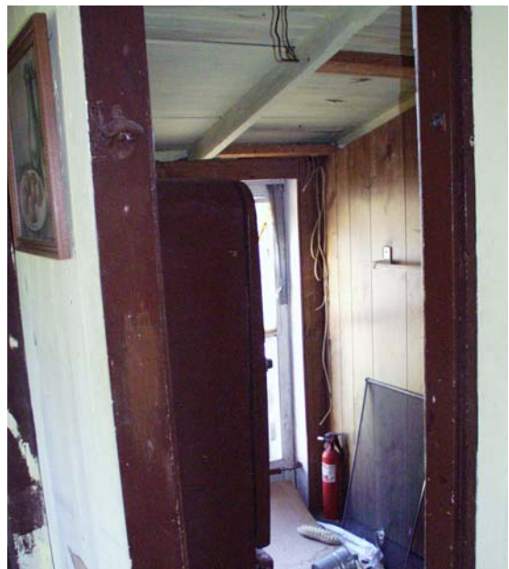
Figure 40 View to north of Room 105. (NPS-SERO-CR, 2003)
