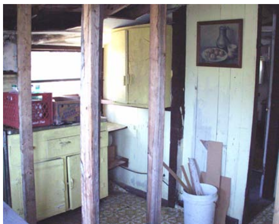
Figure 38 View to north in Room 103. Posts in foreground have been added to stabilize roof structure where wall was removed. (NPS-SERO-CR, 2003)
