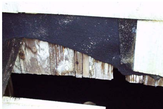
Figure 24 View of typical wood siding and asbestos-cement siding. (NPS-SERO-CR, 2003)
