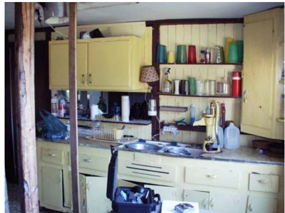
Figure 36 View of kitchen counter and cabinets in Room 103. (NPS-SERO-CR, 2003)
