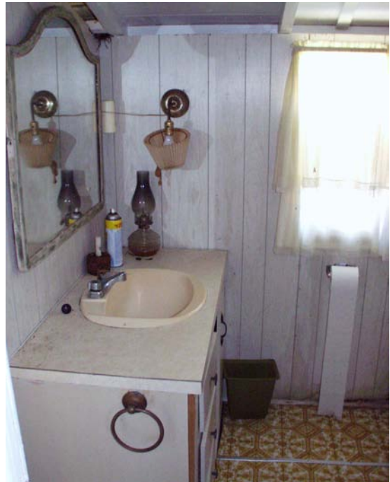
Figure 39 View northwest of bathroom. (NPS-SERO-CR, 2003)
