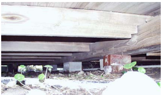
Figure 20 View west under Room 101. (NPS-SERO-CR, 2003)
