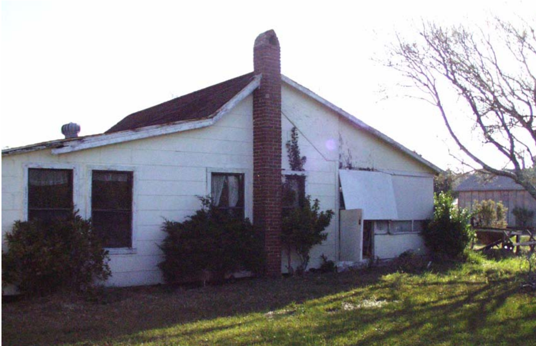
Figure 17 View east of house. (NPS-SERO-CR, 2003)
