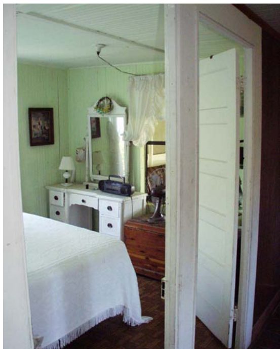
Figure 29 View to east of Room 101, through double doors that originally opened into two separate rooms. (NPS-SERO-CR, 2003)
