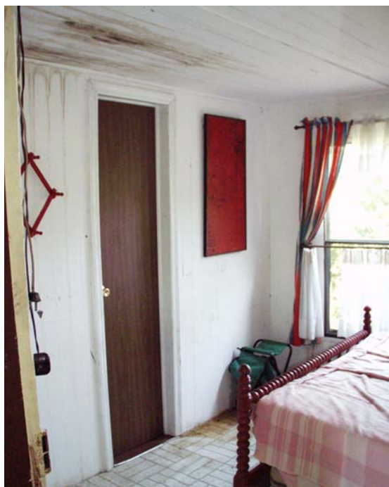
Figure 34 View north of Room 102, showing door added for bathroom. Note water damage to ceiling. (NPS-SERO-CR, 2003)
