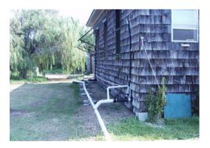
**Figure 39** View of waste lines at rear of house. (NPS-SERO-CR, 2003)
