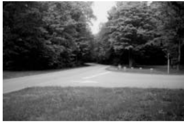
FIGURE 43. View of the confusing transition between New Garden Road's modern and historic courses, as seen from the island situated between the visitor center's divided entrance drives. Note the close proximity of the paved bypass (shown curving into the background) to the restored trace (the beginning of which is blocked by bollards).
