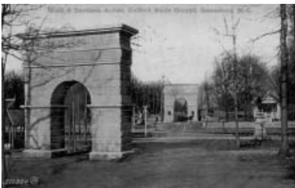
FIGURE 20. The Nash & Davidson Arches (erected 1905, dismantled 1937).
