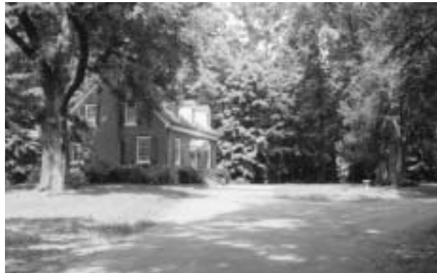
FIGURE 55. The Superintendent's Residence (Quarter's No. 1)
