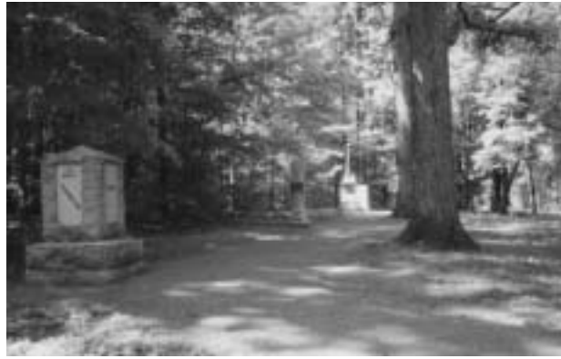
FIGURE 54. View of Monument Row, looking westward down the exposed-aggregate path that links the New Garden trace to the visitor center hardscape.
