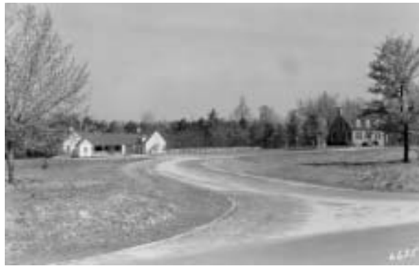
FIGURE 28. Superintendent's Residence - Maintenance Complex, 1935.
