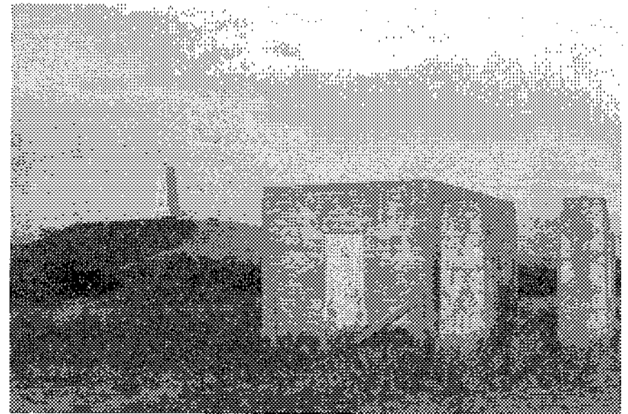
Figure 38. Abandoned entrance station, 1977.
