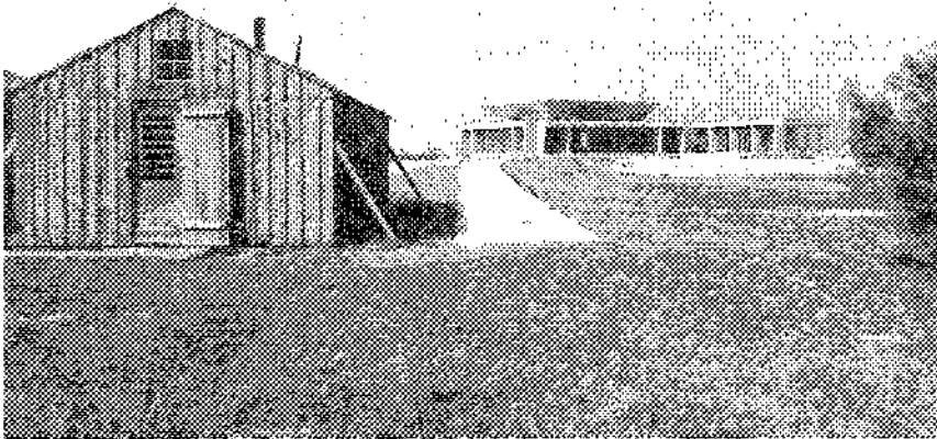
Figure 33. Camp buildings and visitor center, 1960.
