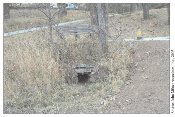
Figure 3-200 (E-08) Stone culvert beneath sidewalk at Visitor Center.
