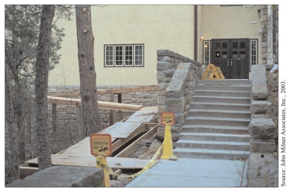
Figure 3-120 (E-16) Wheel chair accessible ramp at north end of Visitor Center during construction.
