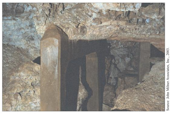
Figure 3-82 (CB-01) Painted concrete reinforcement pillars.
