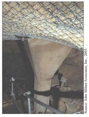
Figure 3-81 (CA-05) Concrete pillars and chain link fence for stabilization with handrail and light fixture.
