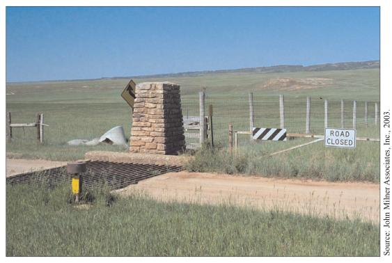
Figure 3-62 (2A-03) Woven-wire perimeter fencing and cattle guard at park's boundary at NPS 5.
