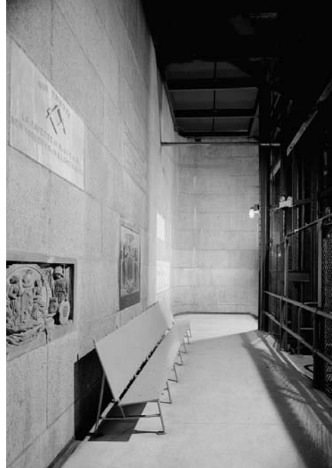
Figure 2. 160-ft. level, 1994. [Historic American Buildings Survey, HABS DC, WASH, 2-102; Prints and Photographs Division, LOC.]
