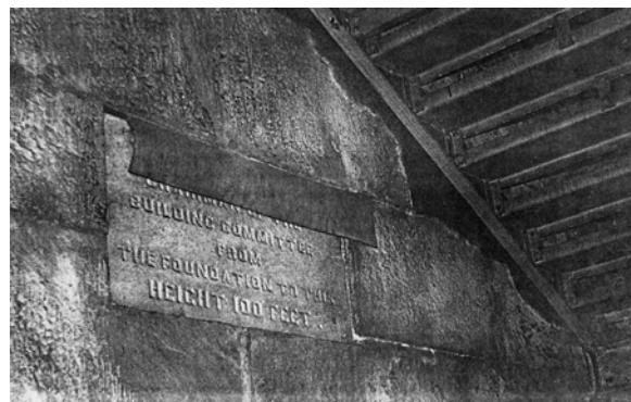
Figure 11. Lead flashing covers the top third of Chairman of the Building Committee. [1974 photo.]
