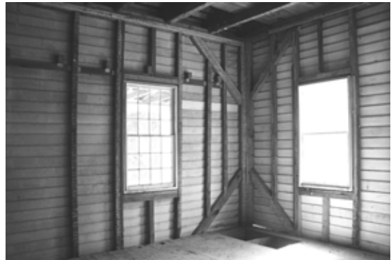
Figure 40 View of northeast corner of frame. NPS SERO 2001.
