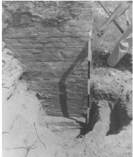
Figure 27 Excavated foundation at southeast corner of house, 1965. VICK Coll.
