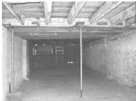
Figure 63 View east in Room 001. NPS SERO 2001.
