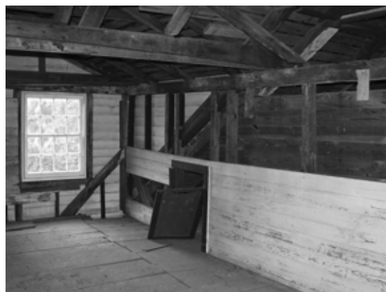
Figure 69 View to northeast in Room 200. NPS SERO 2001.
