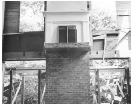
Figure 31 View east after removal of floor in Room 105, May 1966. VICK Coll.
