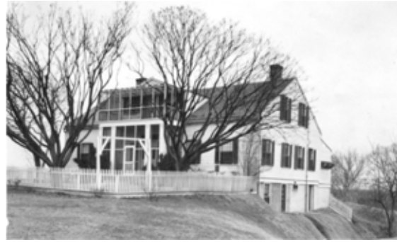
Figure 19 View of front of house, 1940, showing screening of porch and balcony. VICK Coll.
