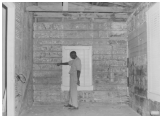
Figure 26 View west in Room 103, with original board wall intact, pointing out Civil-War-era bullet hole. VICK Coll.
