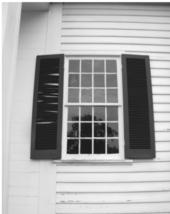
Figure 44 View of typical first floor window and finishes. NPS SERO 2001.
