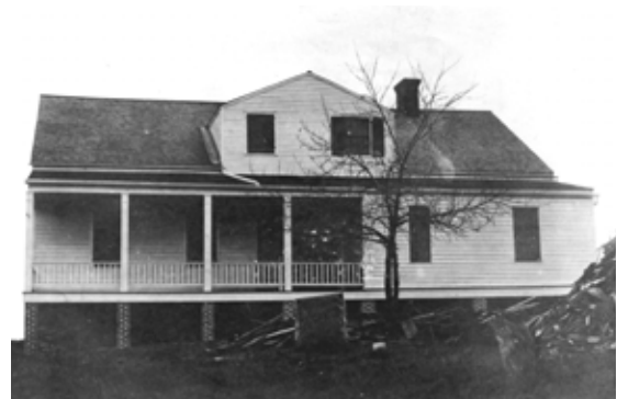
Figure 12 North (rear) elevation after the restoration work accomplished September 26 to November 14, 1902. Note large pile of debris at lower right. HABS File No. MISS, 75-VICK, V. 3-11.
