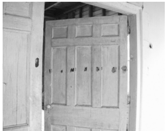
Figure 59 View from Room 105 of double doors in Figure 42. NPS SERO 2001.
