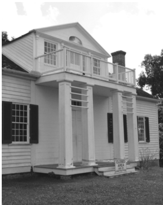
Figure 36 View of front portico and second floor balcony. NPS SERO 2001.
