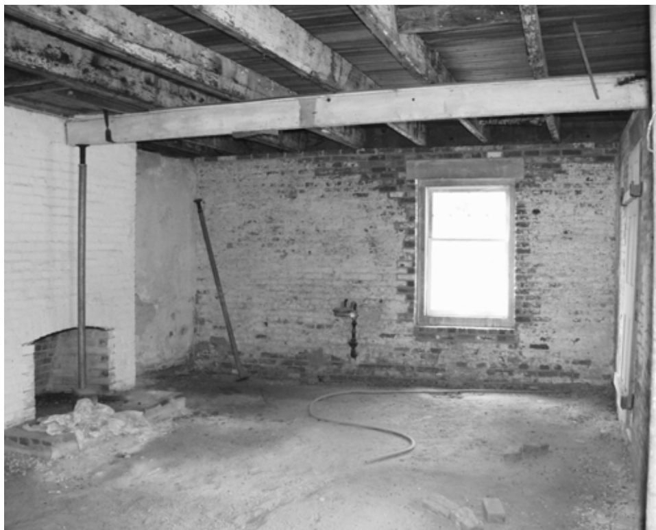
Figure 64 View of western end of dining room. NPS SERO 2001.
