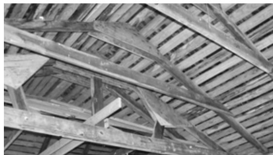
Figure 42 View of roof framing showing added plywood reinforcement. NPS SERO 2001.
