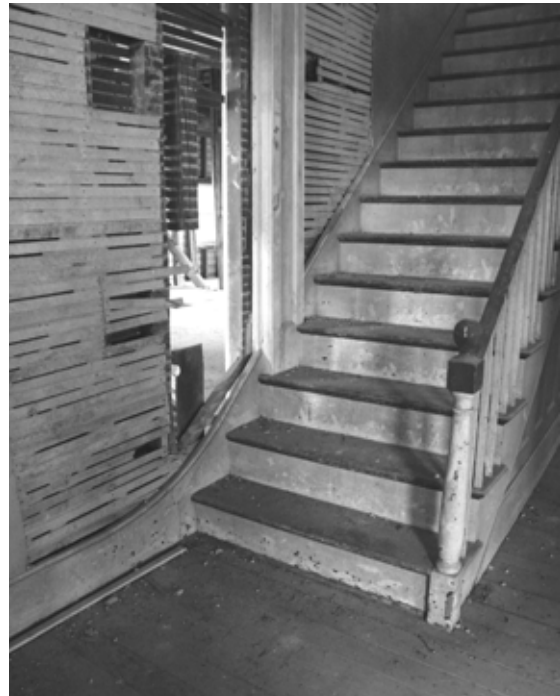
Figure 52 View of main staircase. NPS SERO 2001
