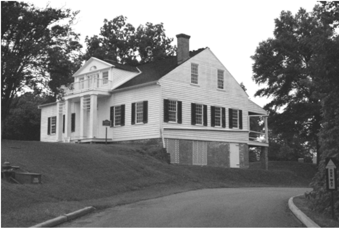
Figure 37 View northwest along Union Avenue. NPS SERO 2001.
