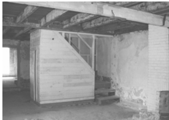
Figure 62 View east of stairs added in 1932. NPS SERO 2001.
