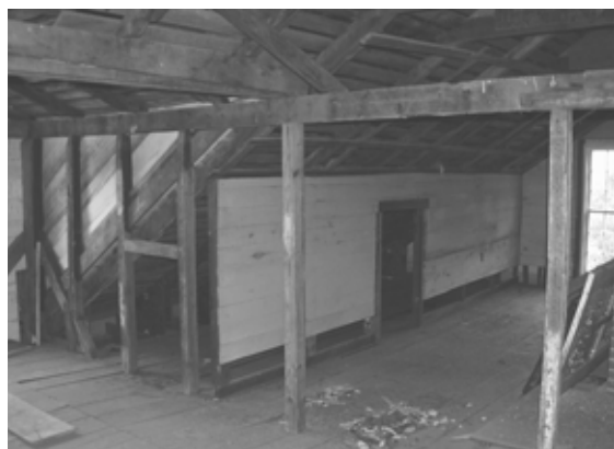
Figure 68 View southwest in Room 200. NPS SERO 2001.
