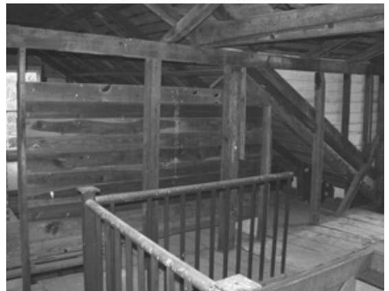
Figure 66 View northwest in Room 200. NPS SERO 2001.
