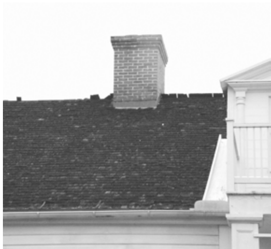
Figure 43 View of south slope of roof and west chimney. NPS SERO 2001.
