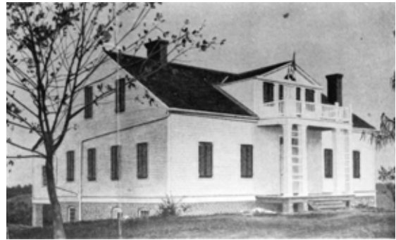
Figure 11 View from southwest after restoration work accomplished September 26 to November 14, 1902. HABS File No. MISS, 75-VICK, V. 3-9.
