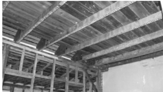
Figure 41 View of typical first floor ceiling framing. NPS SERO 2001.
