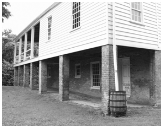
Figure 38 View of basement and porches on north side. NPS SERO 2001.
