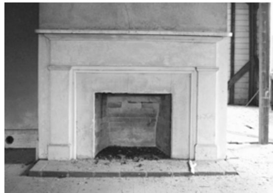
Figure 56 View of reconstructed mantle in Room 102. NPS SERO 2001.
