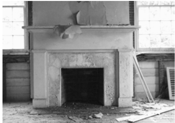
Figure 61 View of mantle piece installed in Room 105 in 1939. NPS SERO 2001.
