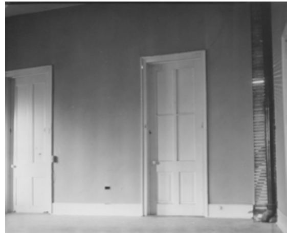
Figure 23 View north in 102, showing doors into Room 103, November 1965. VICK Coll.
