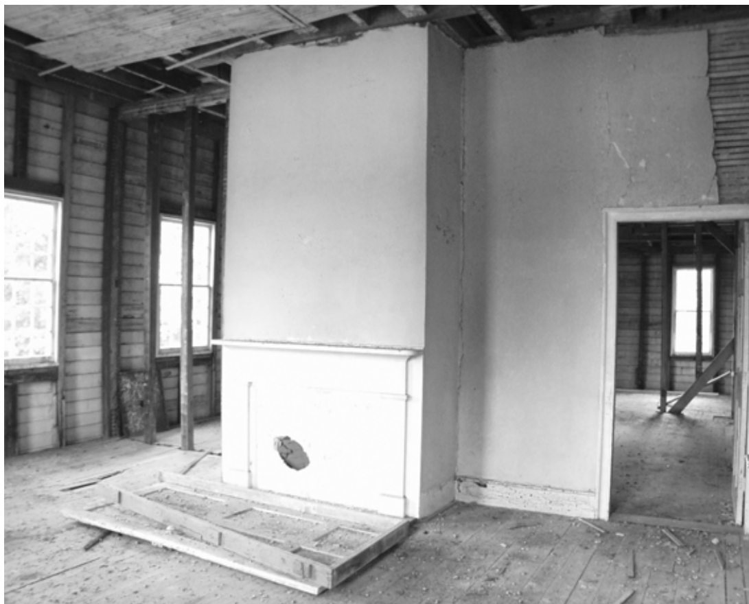
Figure 54 View to northwest in Room 101. NPS SERO 2001.
