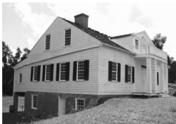
Figure 33 View of house from southwest. NPS SERO 2001
