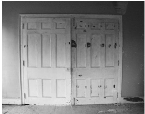
Figure 58 View of double doors between Rooms 104 and 105. NPS SERO 2001.
