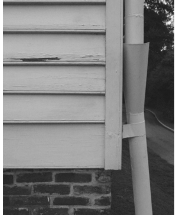
Figure 45 View of typical siding and corner trim. NPS SERO 2001.
