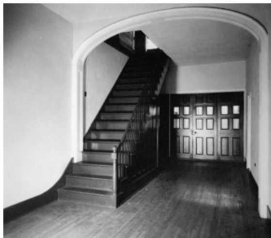
Figure 17 Central hallway, looking north, 1940. Note glass added in back doors. HABS File No. MISS, 75-VICK, V.3-20.
