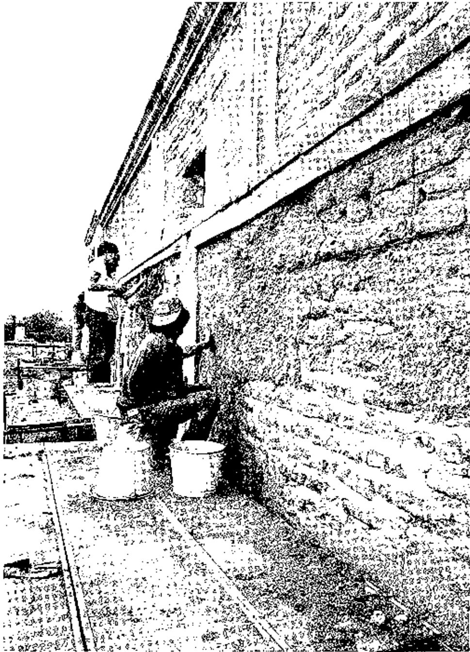
1. West church wall during the filling of voids.
