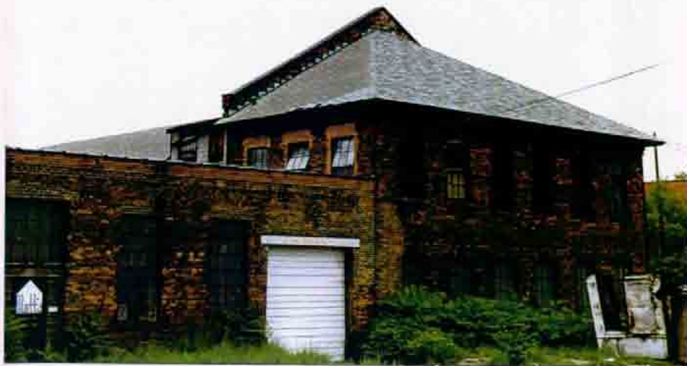
Figure 3.14 Detail of the east elevation of Infill Bay 3 (to the left of Bay 4).
