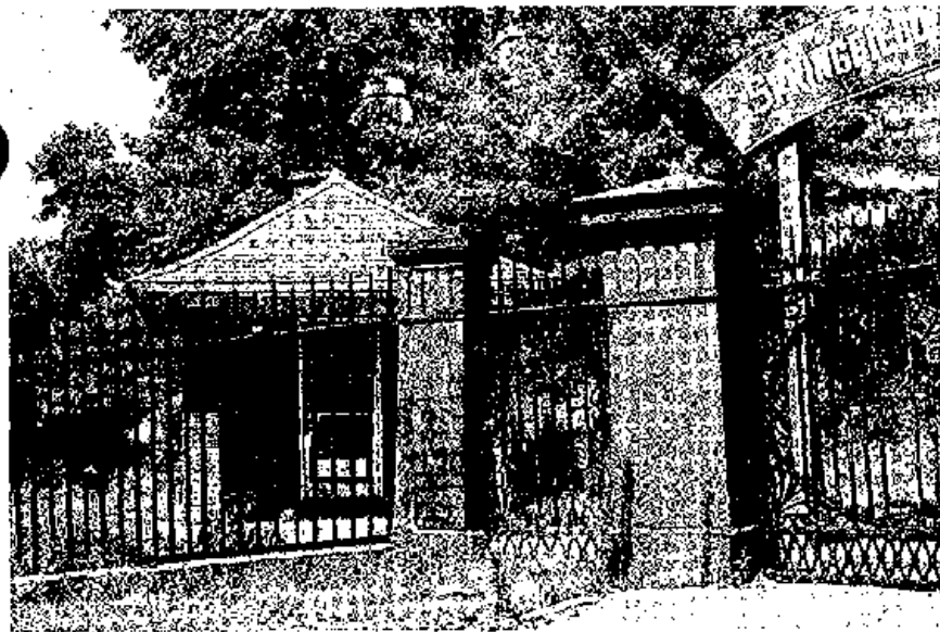
Illustration 118 Fence South Gate and Gatehouse
